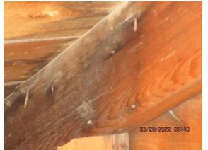
Attic Framing/Sheathing: Garage attic space with limited visibility. Evidence of past water intrusion.
