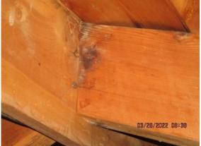
Attic Framing/Sheathing: House attic. Evidence of past water intrusion. Does not appear to be any new leaks with new roof installed.
