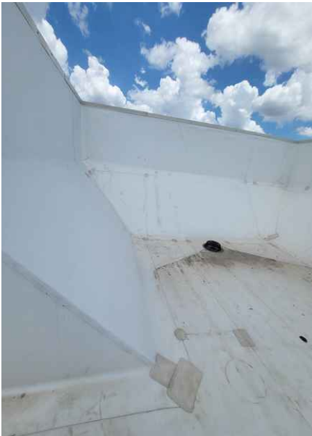
Roof to wall flashing
