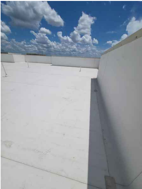
Roof to wall flashing
