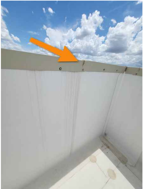
Poorly sealed allowing moisture intrusion
