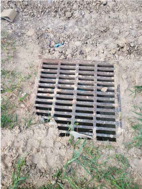
Strom drains - grate inlet
