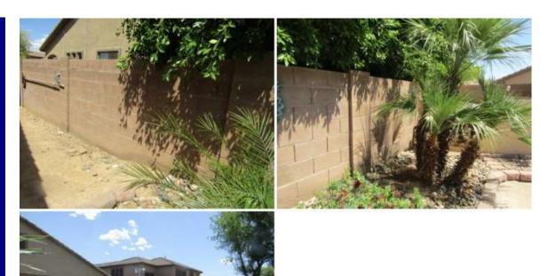
Repair: A couple of the column caps are loose on the fence around the yard. This should be corrected for the safety of anyone playing around the fence, especially children.
