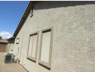
Note: The overall stucco is in good condition and is sealed with most minor cracks or blemishes being a cosmetic condition only. However, penetrations through the wall and joints between dissimilar materials need to be caulked periodically.
