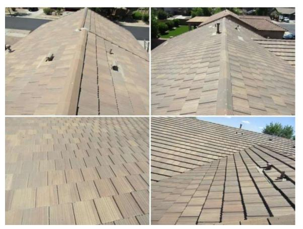
**Repair:** There is one cracked/broken field tile that should be replaced to prevent the possibility of water draining under the tiles and having access to the underlayment and needs to be repaired by a qualified contractor. The tile is on the east facing.
