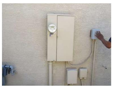
The service voltage available to this building was single phase 120/240 volts. Branch circuit overload protection was provided by circuit breakers and the available ampacity provided through the service was 200 amps.
