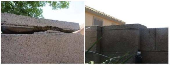
**Monitor:** The fence is cracking, most likely from tree roots. Although it is still sturdy, it should be monitored to ensure the safety of anyone playing around the fence, especially children.
