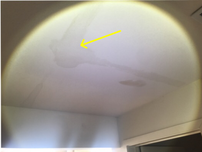
Evidence of moisture. Break room area ceiling. Dry
