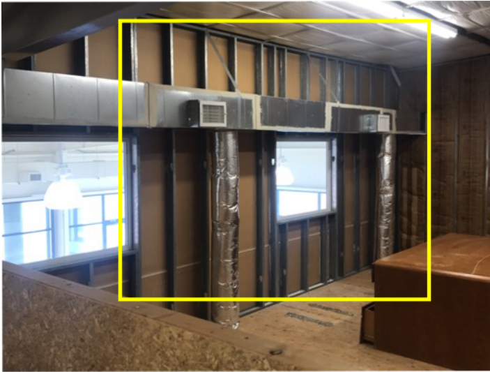
Missing vertical insulation. Unfinished upstairs Building 2 area
