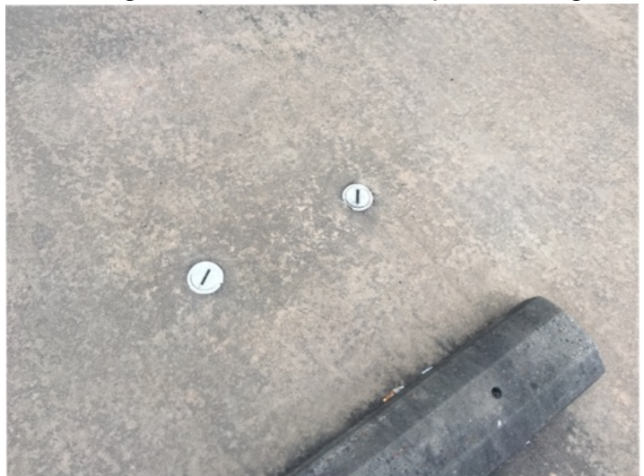
Building 1 sewer clean outs. Rear
