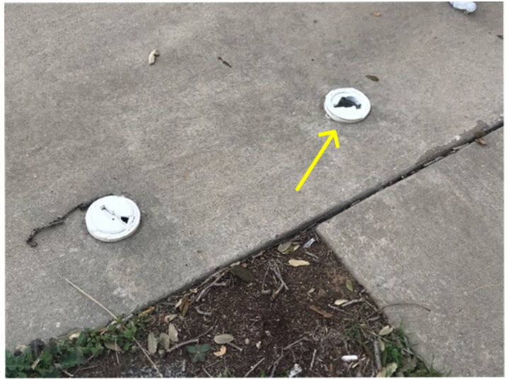
Building 2 clean out. Broken caps. Front right
