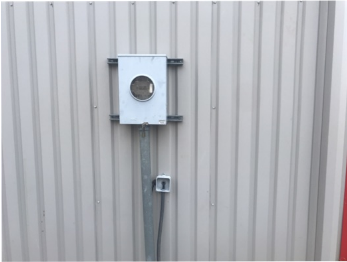
Building 2 main electrical meter
