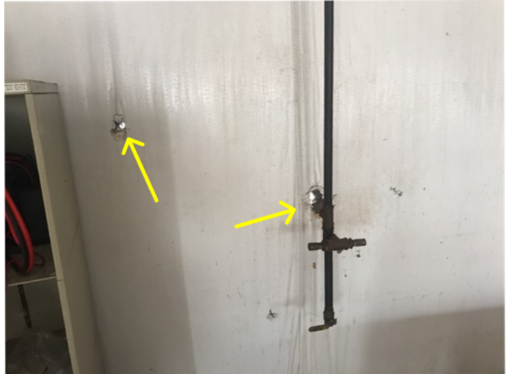
Building 2 walls holes. Rear
