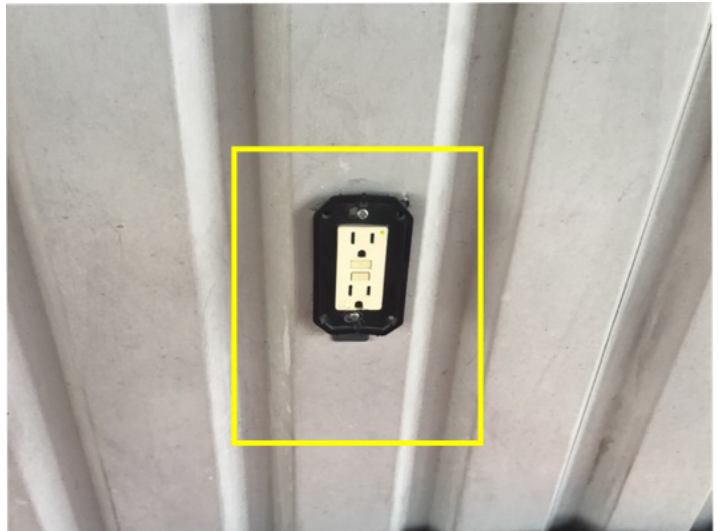
Missing switch cover. Building 1 service bay
