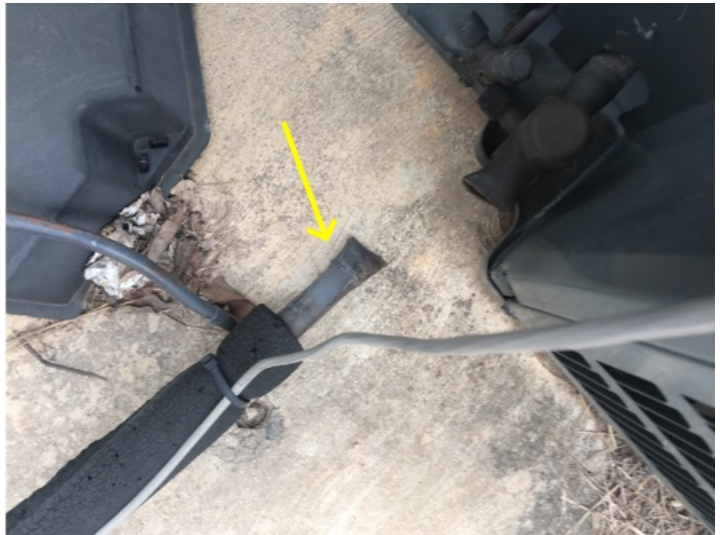
Broken refrigerant line. Condenser 2
