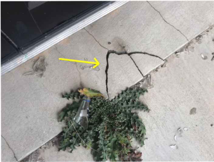
Damaged thresholds. Several exterior doors
