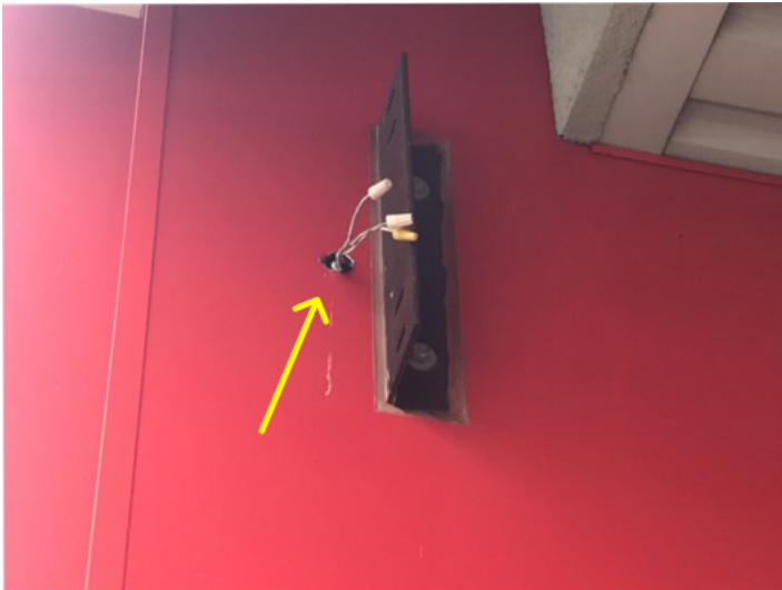
Exposed wires. Front
