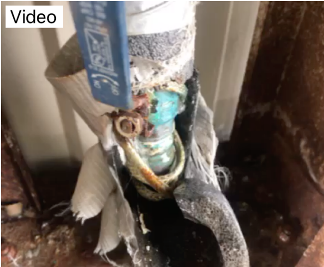
Water leak. Service bay
