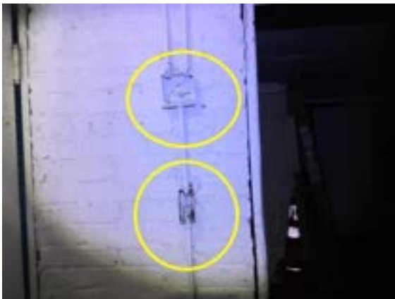
Interior Foundation Left: open junction boxes
