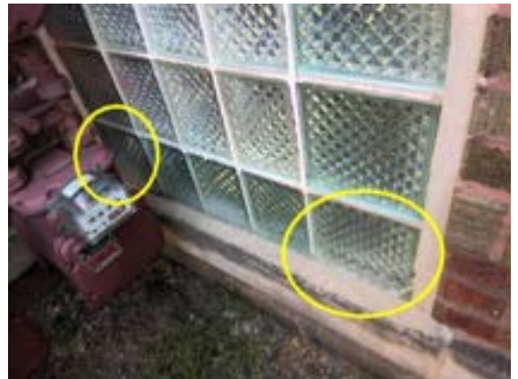
FENESTRATION SYSTEMS: cracked front
