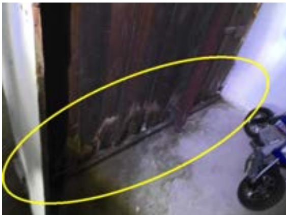
INTERIOR FOUNDATION RIGHT: mold/rot
