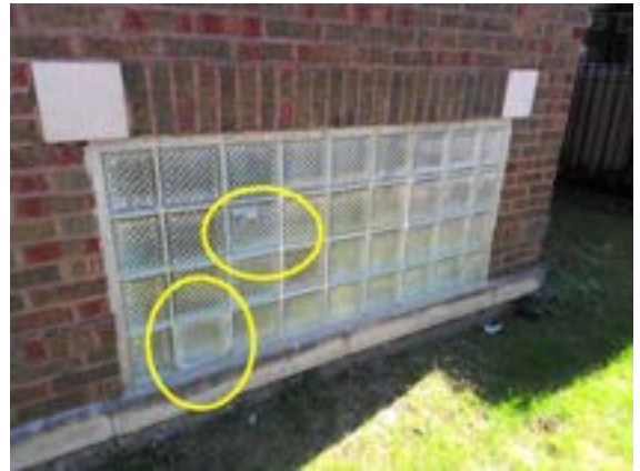
Fenestration Systems: cracked front
