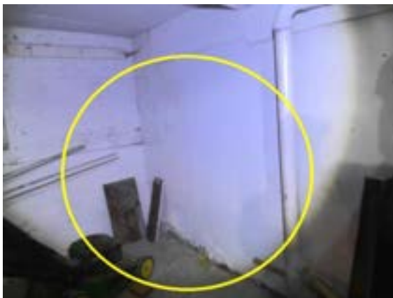
INTERIOR FOUNDATION RIGHT: mold/moisrure
