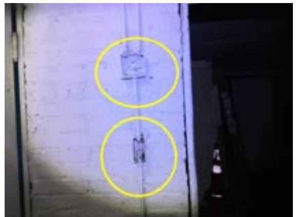
INTERIOR FOUNDATION LEFT: open junction boxes
