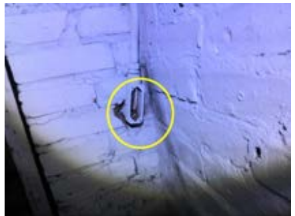
INTERIOR FOUNDATION LEFT: exposed wires
