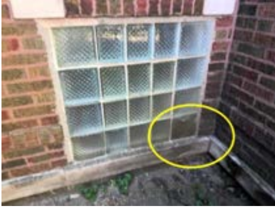
Fenestration Systems: cracked front
