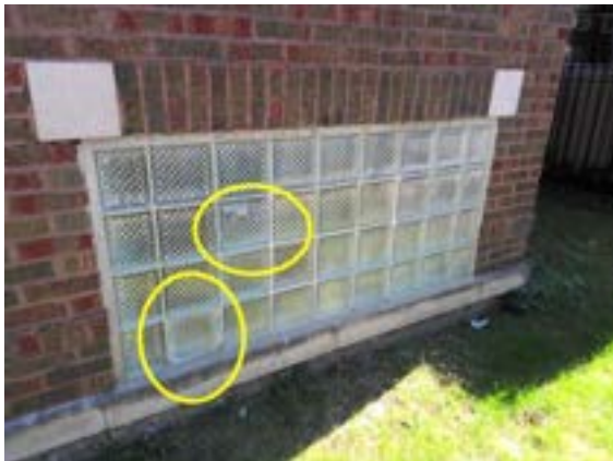
FENESTRATION SYSTEMS: cracked front
