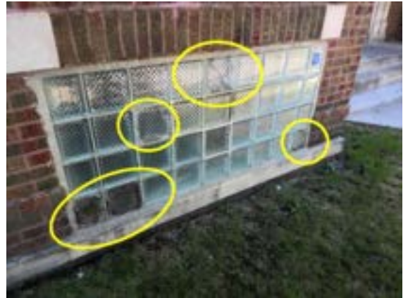
FENESTRATION SYSTEMS: cracked front
