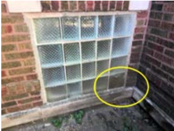
FENESTRATION SYSTEMS: cracked front
