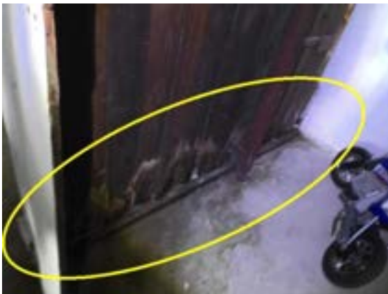
Interior Foundation Right: mold/rot
