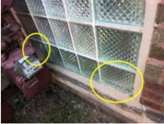
Fenestration Systems: cracked front
