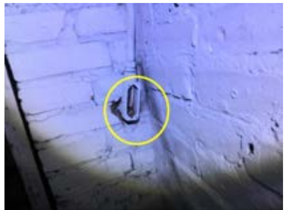
Interior Foundation Left: exposed wires
