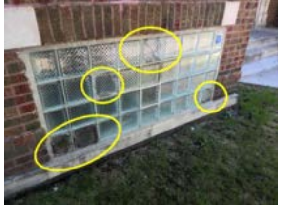
Fenestration Systems: cracked front
