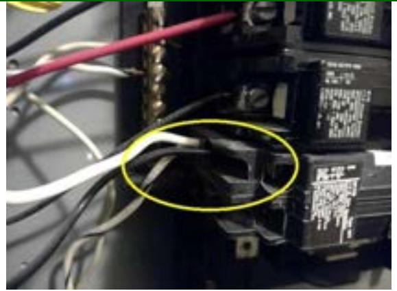
ELECTRICAL: Triple wire tapped.
