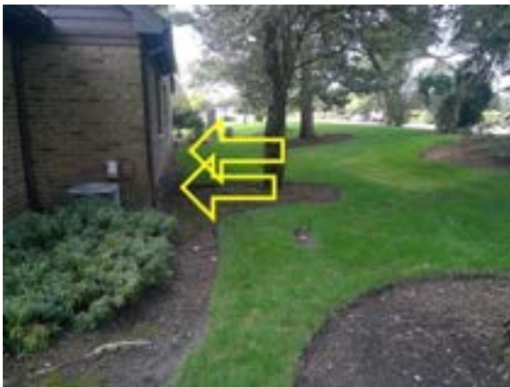
Grading / Drainage: Negative slope.
