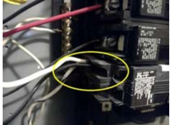
Electrical: Triple wire tapped.
