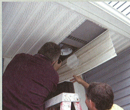
Workers open the porch roof for inspection.
