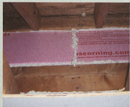
The finished product—the gap in the sheathing after sealing.
