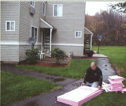
Hundreds of pieces of insulation are cut for air sealing.
