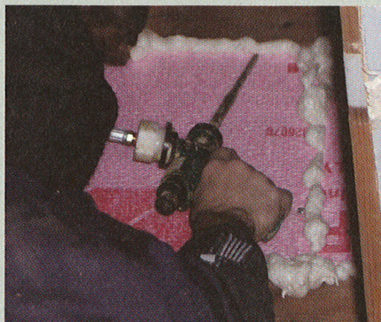
The sheathing is being sealed with rigid insulation and spray foam.
