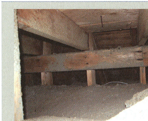
There is not much space to access the existing attic.
