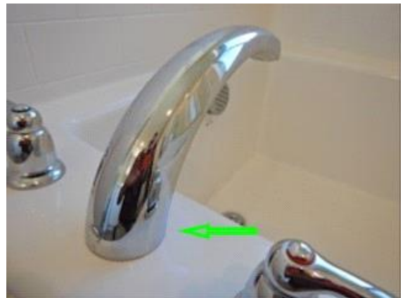
Bathroom 3: tub faucet is loose at the base
