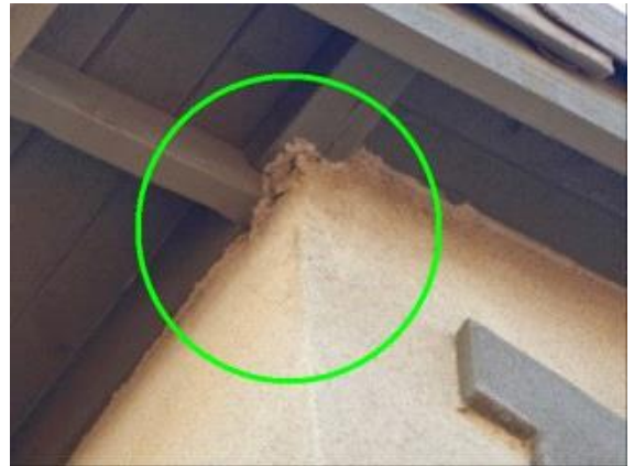
Exterior Surface: cracks and chipping stucco located on the upper north west corner exterior wall
