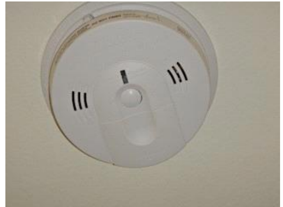
Electrical: first floor smoke detector/carbon monoxide combination unit
