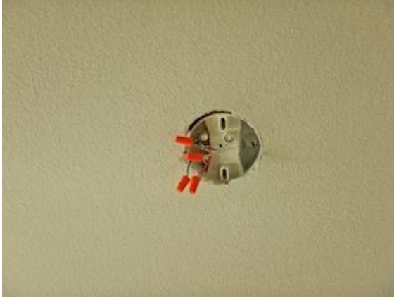
Loft: junction box is missing the cap
