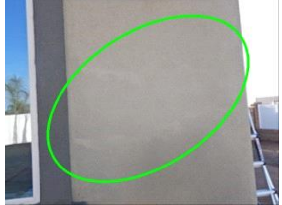
Exterior Surface: observed mismatch color on the east facing stucco wall
