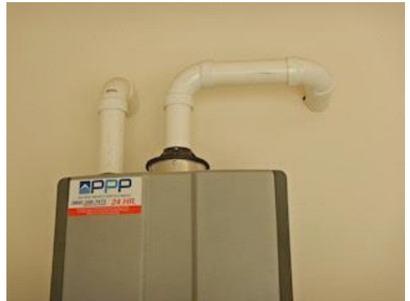
Draft Control/Vent: water heater
