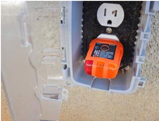
Electrical: patio outdoor outlet is not energized
