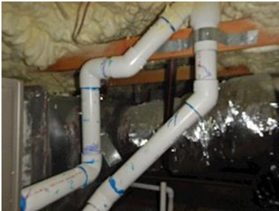
Draft Control/Vent: furnace
