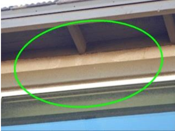
Exterior Surface: stain on the north facing exterior wall
