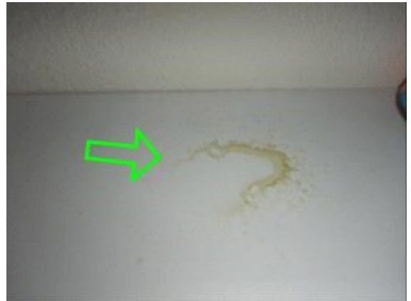
Bathroom 2: noted evidence of a drain leak under the second sink
