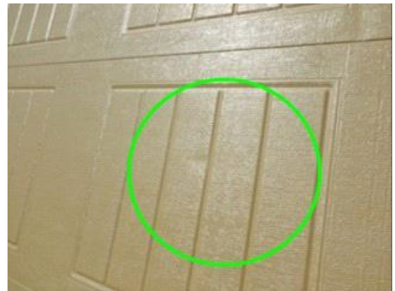
Overhead Garage Doors: noted a dent on the small garage door
