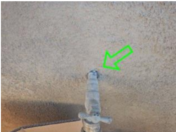
Exterior Surface: noted a gap on the patio hose Bibb at the wall
