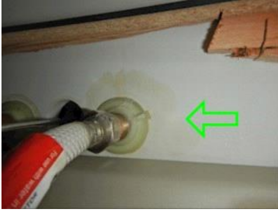
Bathroom 3: evidence of a water stains under the faucet
