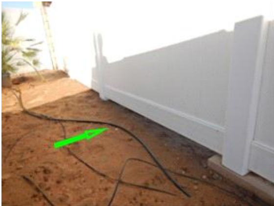
Fences / Gates: observed footing missing on the north facing vinyl fence, possible future soil erosion
