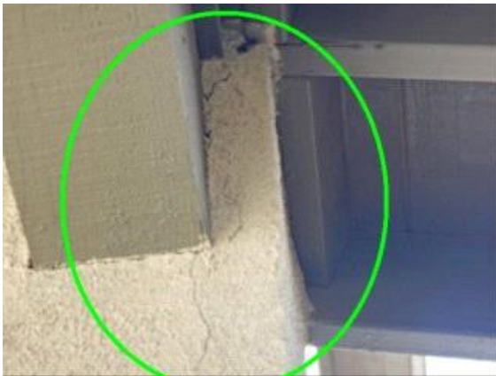
Porches / Stoops: observed stucco cracks on the porch ceiling
