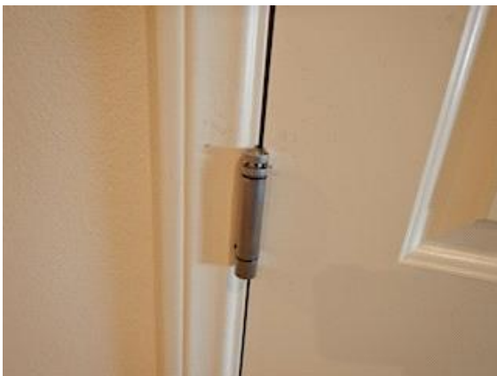
Garage Pedestrian Door into House: adjustable hinge
