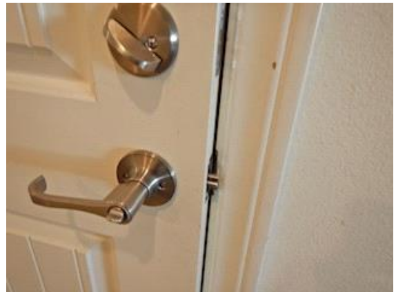
Garage Pedestrian Door into House: the self closing device on the pedestrian door is not functioning ( door is not closing )
