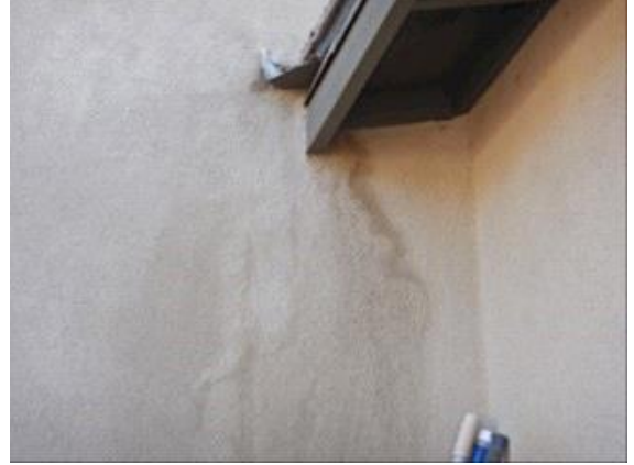
Exterior Surface: observed dark stains on the west exterior wall
