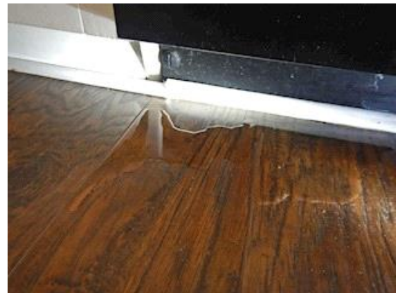
Kitchen: the dishwasher is leaking water
