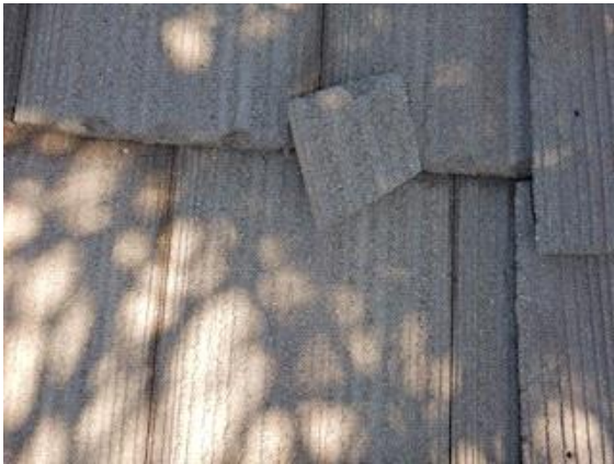
Roofing: noted a piece of roof tile on the rear side
