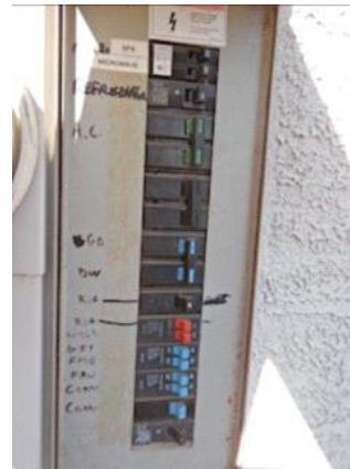
Electrical: not all breakers are clearly labeled
