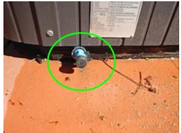
Hot Tub / Spa: observed a water leak
