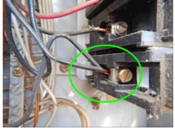
Electrical: noted a breaker with double tap wires
