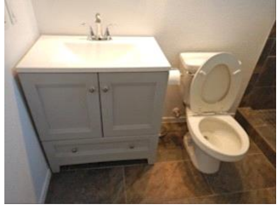
Bathroom 1: the sink is missing the splash guard
