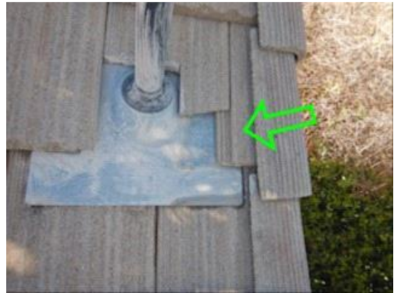
Roofing: noted a piece of roof tile missing, the loose piece is still on the roof
