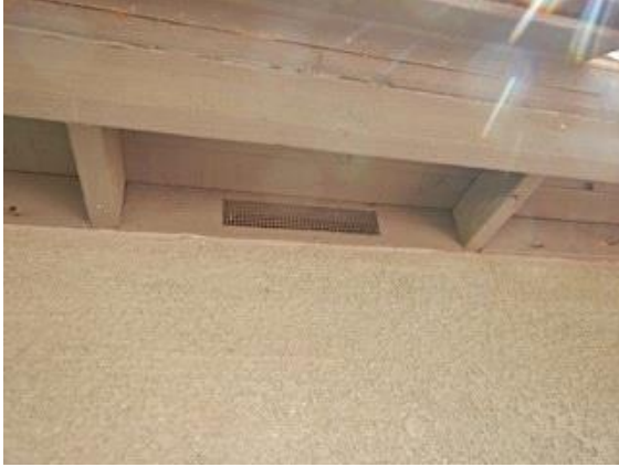
Attic Ventilation: soffit
