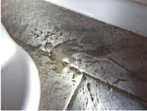
Bathroom 1: observed a water leak under the toilet tank
