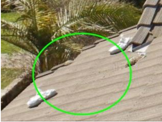
Garage/Carport: roof area of the garage where water is leaking from
