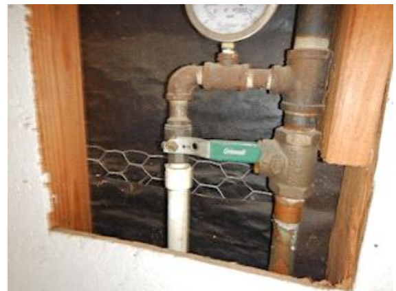
Plumbing: the fire sprinkler valve is on the off position
