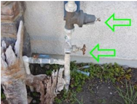
Plumbing: water regulator and water shut off
