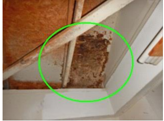
Garage/Carport: observed wet roof sheathing on the garage ceiling
