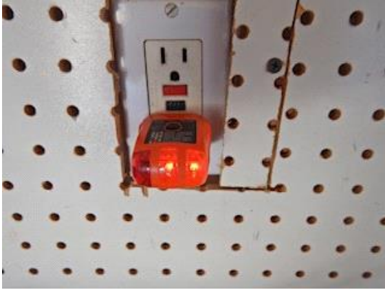
Garage/Carport: garage GFCI outlet protects both bathrooms
