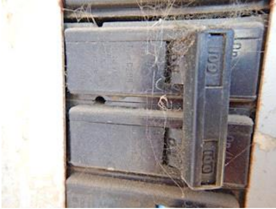
Electrical: main breaker 100 amps
