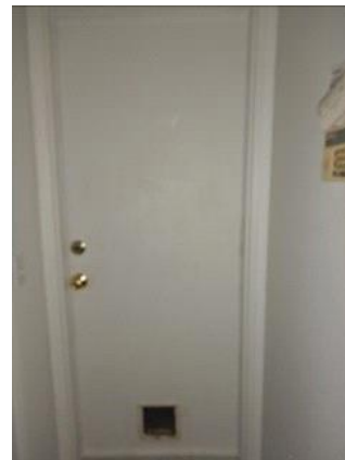
Garage Pedestrian Door into House: garage fire door with a pet access door
