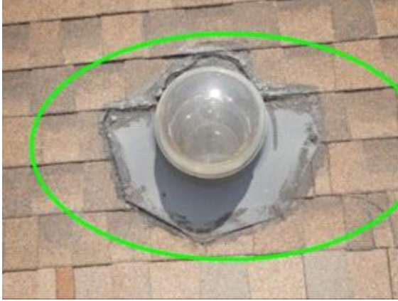
Skylights: noted cracked sealant around the skylight
