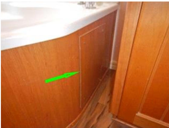
Bathroom 3: tub plumbing access panel
