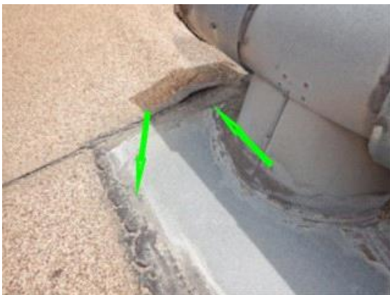
Flashing/Valleys: noted lifting roofing material and cracked sealant
