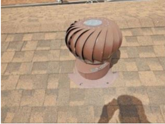
Garage/Carport: the garage turbine vent is not turning
