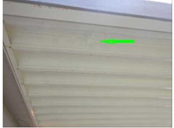
Patio: noted dent on the patio metal roof
