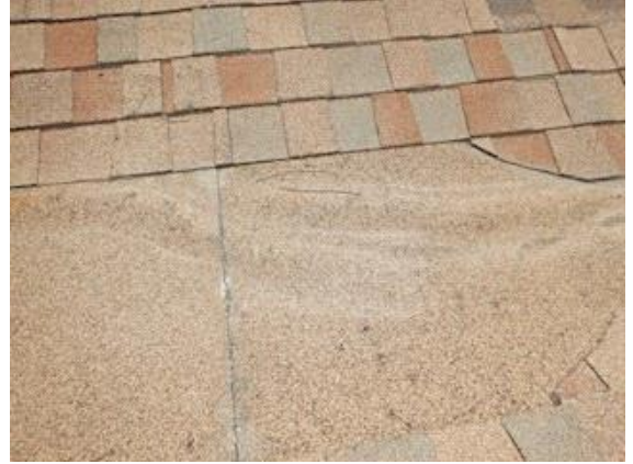
Roofing 1: roof valley shows evidence of pooling water and wrinkled rolled on asphalt roofing material
