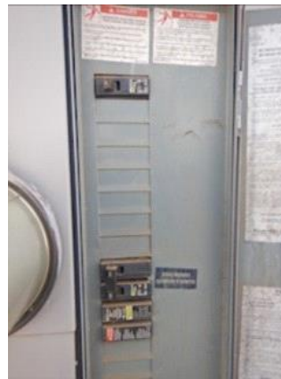
Electrical: left side electrical panel breakers are not labeled for safety
