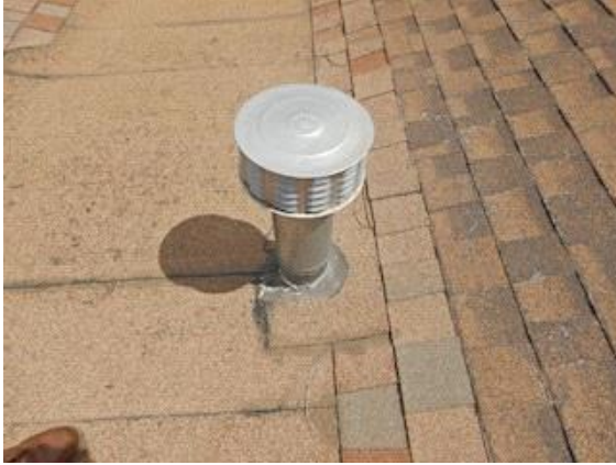
Draft Control/Vent: home heating unit
