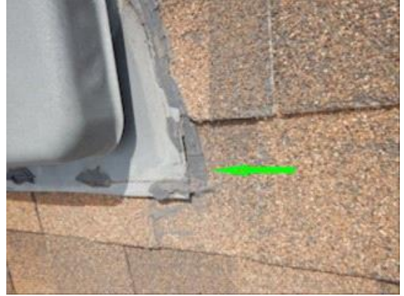
Flashing/Valleys: cracked sealant
