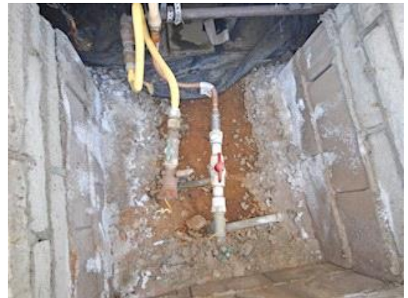
Plumbing: main water shut off
