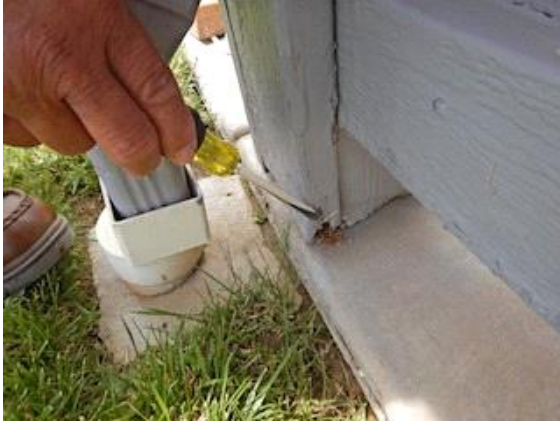
Exterior Surface: noted wood rot on the porch composite trim
