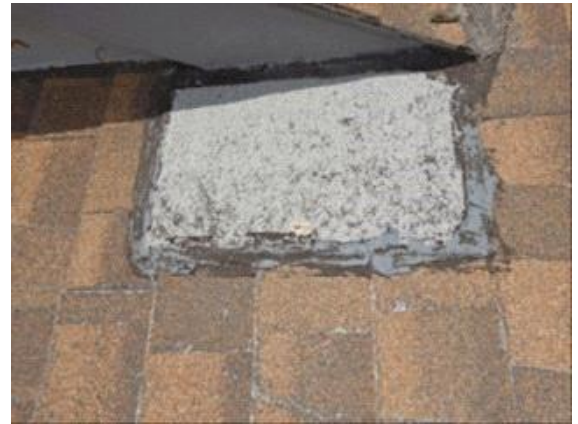
Roofing Dormer over the living room: cracked sealant
