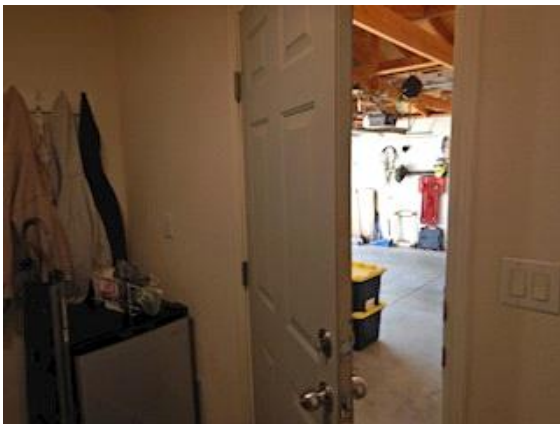
Garage Pedestrian Door into House: the house/ pedestrian door is not self closing
