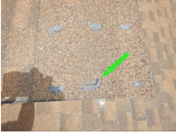
Roofing Dormer over the living room: exposed roof staples
