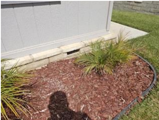
Crawl Space: crawl space vents
