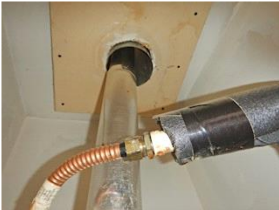
Draft Control/Vent: water heater vent pipe
