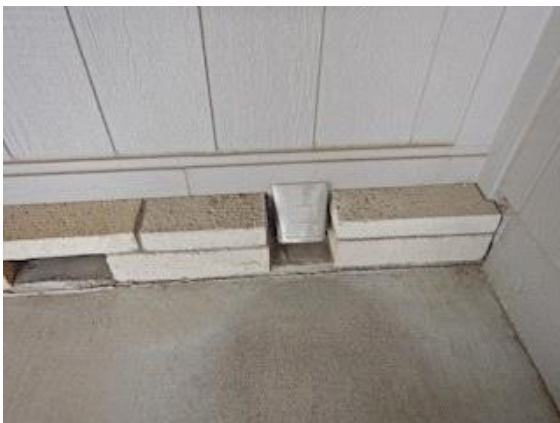
Laundry Facilities: dryer exhaust pipe
