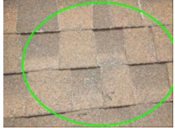
Roofing 1: missing granules
