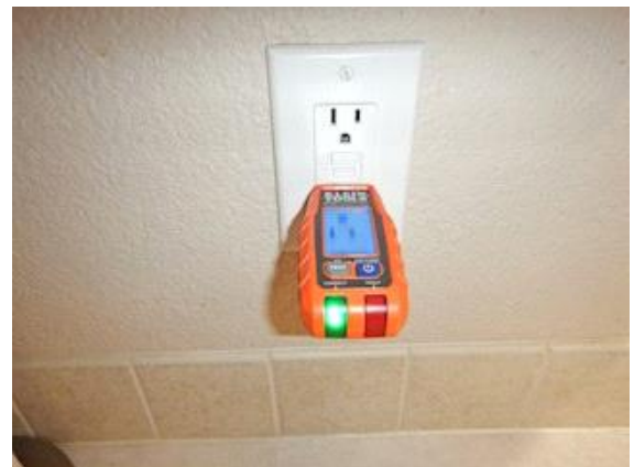
Kitchen: the GFCI is functioning as designed
