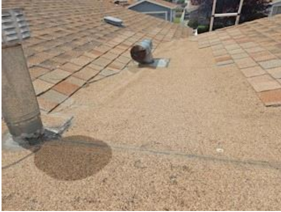
Roofing 1: roof valley
