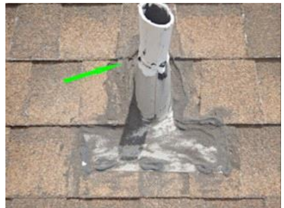
Flashing/Valleys: cracked sealant
