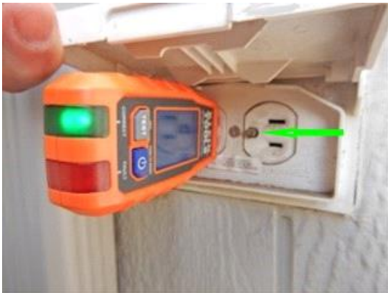
Exterior Surface: noted a ground prong stuck inside opening
