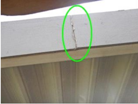
Patio: metal patio molding has evidence of cracked sealant on the seam
