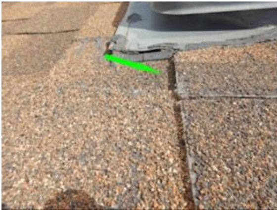
Roofing 1: missing granules on the asphalt shingles
