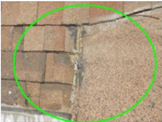
Roofing 1: cracked sealant
