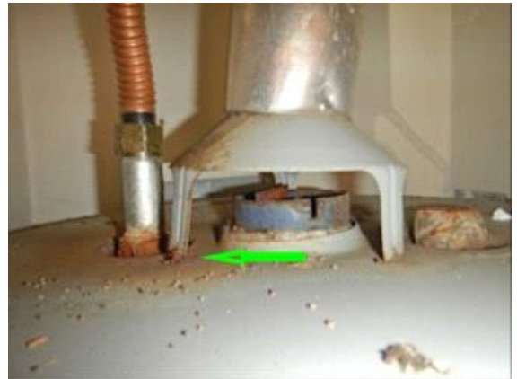
Draft Control/Vent: The water heater vent hood is not installed correctly, the left leg is not inserted
