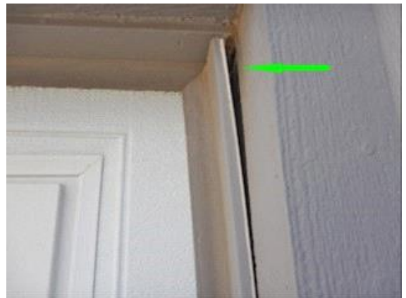
Overhead Garage Doors: the upper right garage door molding is not attached
