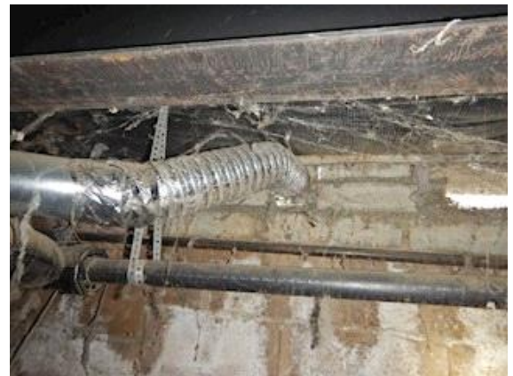
Laundry Facilities: dryer exhaust pipe
