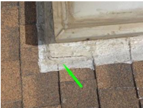
Skylights: noted cracked sealant in the large skylight
