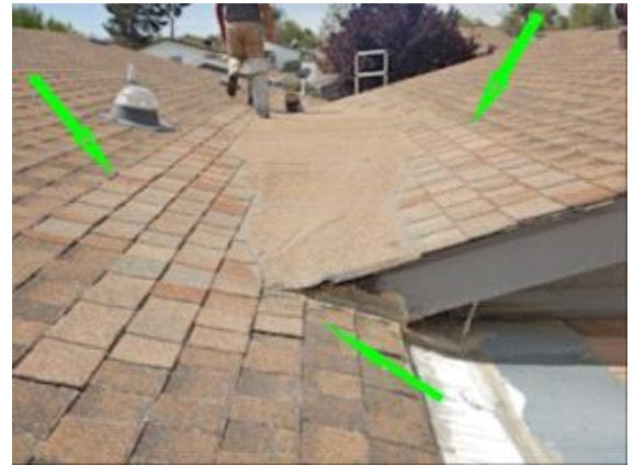
Roofing 1: observed previous roof repairs around the valley
