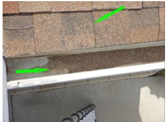
Roofing 1: noted roof granules in the gutters and dark areas on the asphalt shingles show evidence of missing granules
