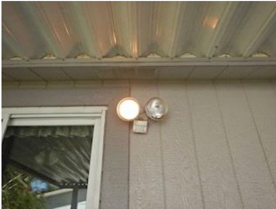
Exterior Surface: right side bulb is out
