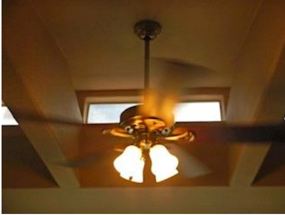
Living room: the ceiling fan is wobbling, needs adjustment
