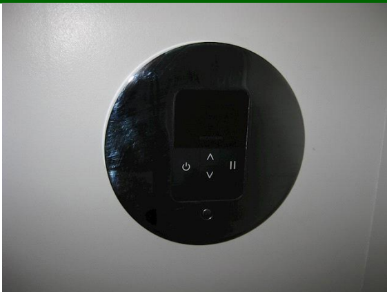
Control panel for steamer in shower
