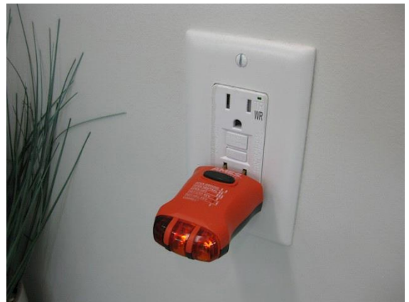
Outlets properly wired in this area
