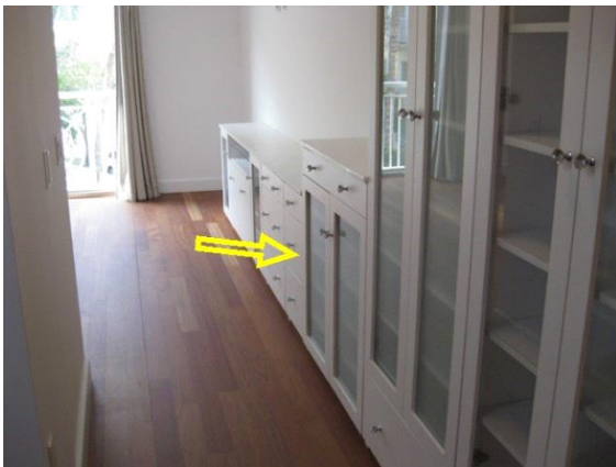
Some cabinets and closet doors did not have the slow-close function, recommend repair to prevent damage on cabinet fixtures
