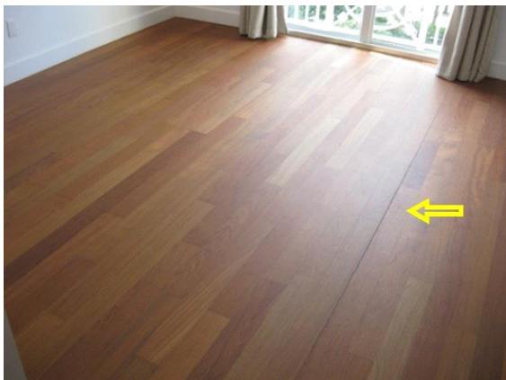
Vinyl flooring showed signs of separation at time of inspection, recommend repair
