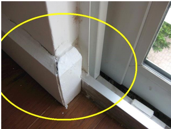
Area was seen to have evidence of moisture intrusion, area was tested with contact humidity meter and no elevated levels of humidity were noted at time of inspection, monitor area
