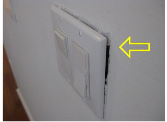
Electrical switch trim showed signs of damage, recommend repair
