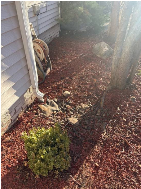
Neutral grading along the south foundation
