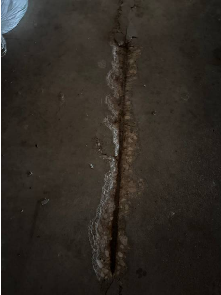
Deteriorated section of garage slab
