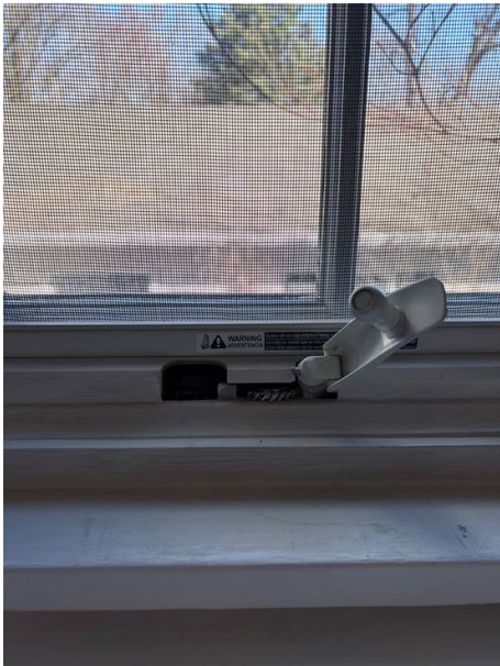
Window right of the fireplace in the living room is missing hardware
