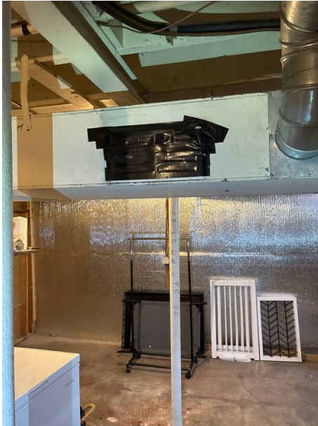
Tapped off vent observed in utility room
