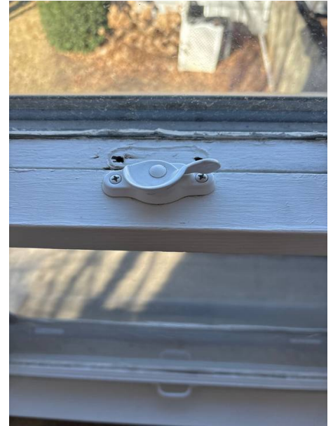
West facing window in south bedroom is missing locking hardware
