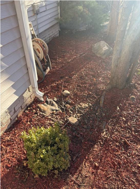
Neutral grading along the south foundation
