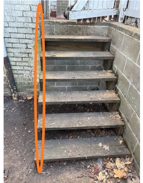
Missing handrail and guardrail on rear steps
