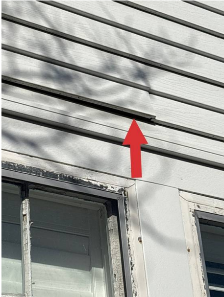
Gap in siding panels above the second-floor window on the east side
