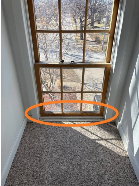
3rd floor window does not meet minimum height requirements and has broken locking hardware
