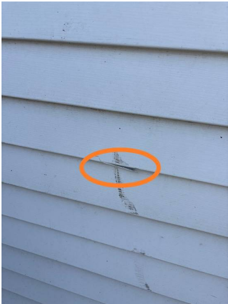
Crack in siding
