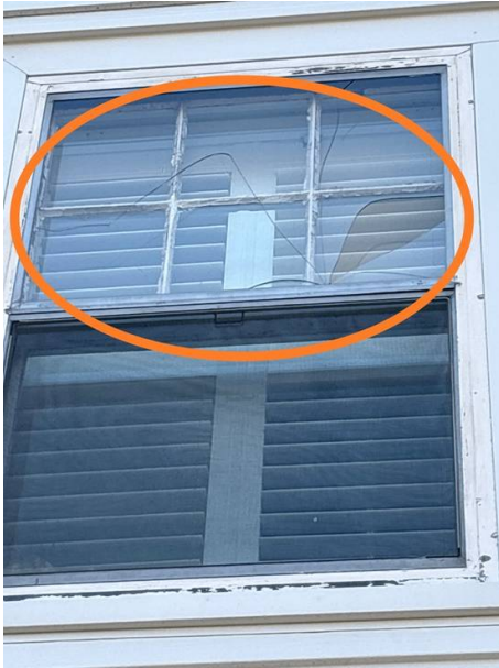
Broken 2nd floor, west facing window
