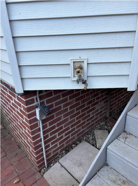
Hose bib at the bottom of the east deck stairs did not dispense water
