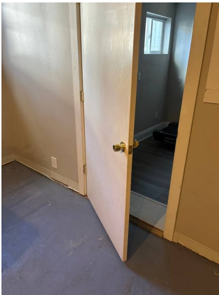
Door to east basement room rubs on floor and ceiling
