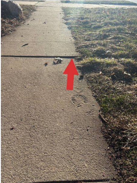
Trip hazard on sidewalk in front of the house
