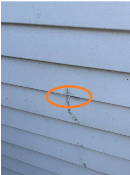
Crack in siding
