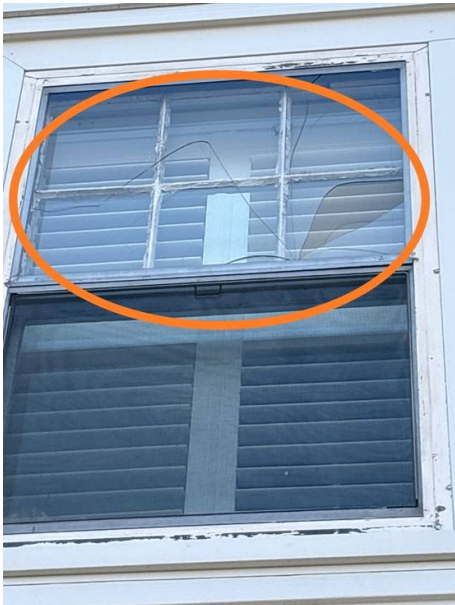
Broken 2nd floor, west facing window
