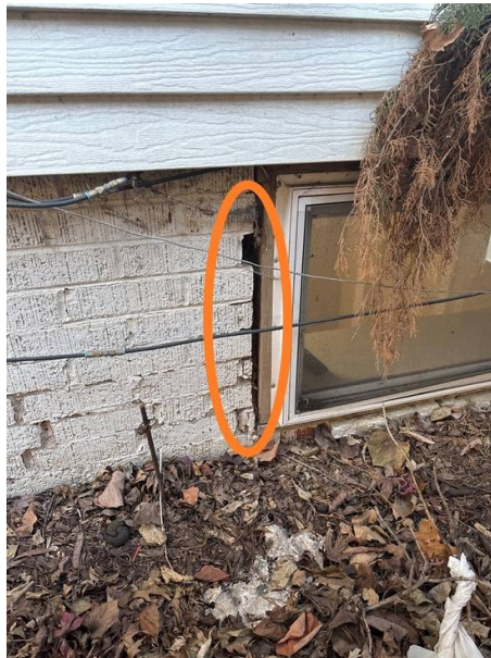
Northeast basement window - bare wood on window frame
