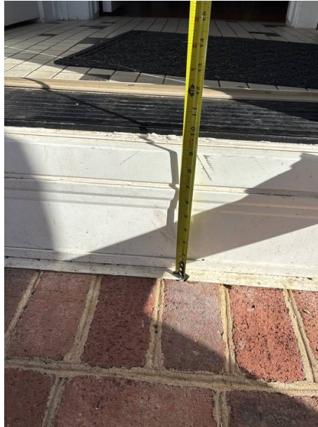
Top step leading to front door exceeds maximum height requirements
