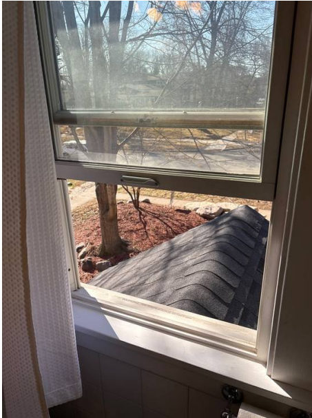
Upstairs hall bathroom window is missing its screen
