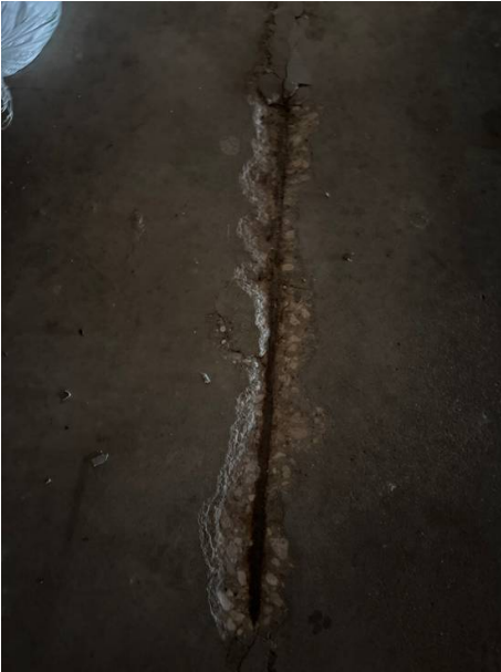
Deteriorated section of garage slab
