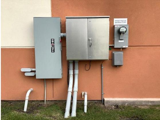
Electrical: Underground service, TECO meter, and electrical disconnect located at left exterior of building.
