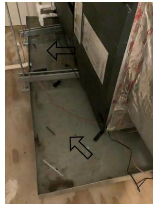
Cooling: Pan filled with water and overflowing in attic
