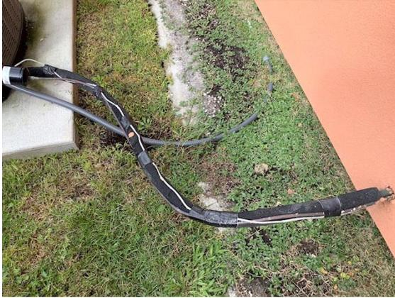
Cooling: Refrigerant lines appear properly insulated
