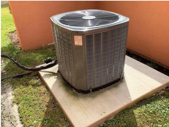
Cooling: Condenser installed on a level pad in like-new condition.
