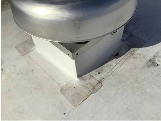
Flashing/Valleys: Typical flashing over garage area appears properly installed
