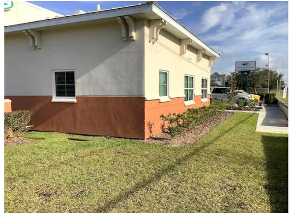
Grading / Drainage: View from rear left of property shows grading away from foundation.
