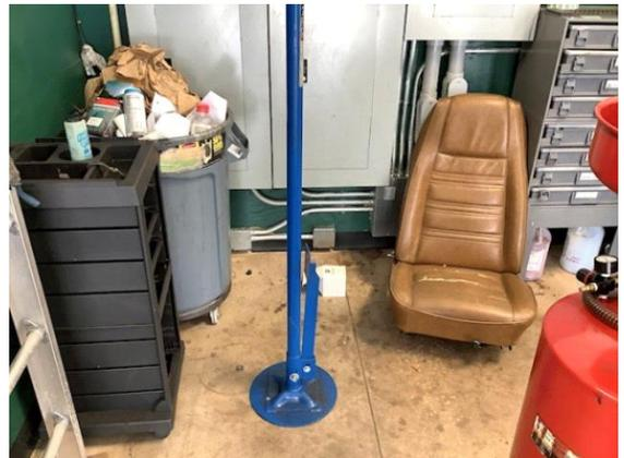
Electrical: Sub panels located on left wall of garage. No clear workspace marked along the floor in front and adjacent to the panels.
