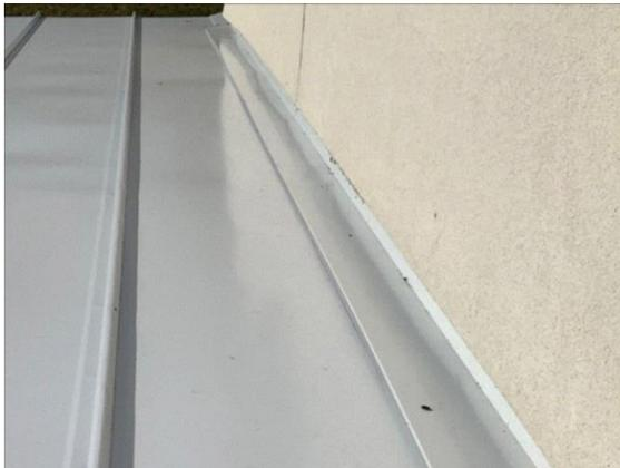
Proper intersection clearance where wall meets roof
