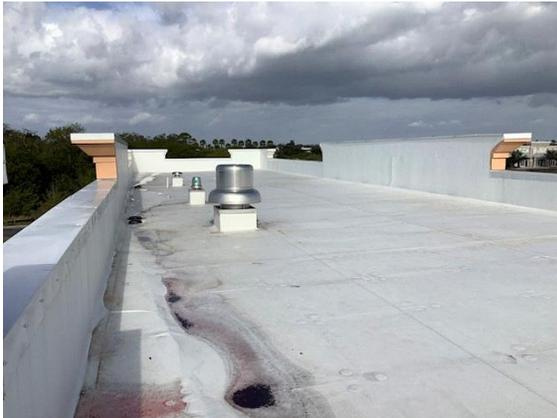
Roofing: TPO roofing over garage bays
