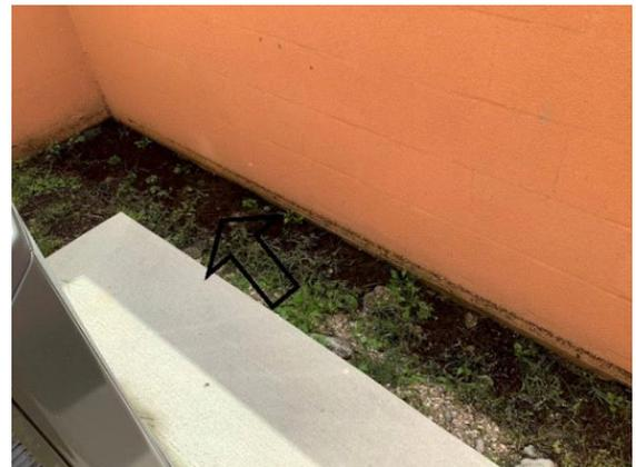
Cooling: Water cannot escape condenser enclosure. Weep holes needed or clogged.
