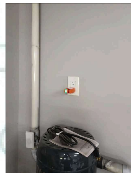
Missing GFCI - Garage
