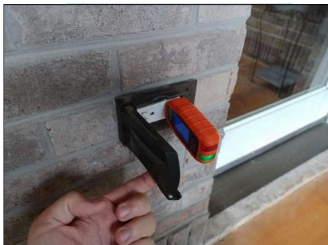
Missing GFCI - Exterior
