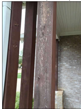
Deteriorated stain on front porch posts
