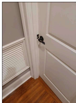
Door contacting frame - bedroom
