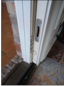
Damaged weather strip
