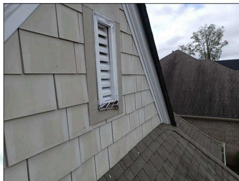
Damaged louver vent
