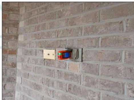
Missing GFCI - Exterior
