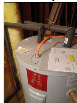
Missing electrical shutoff
