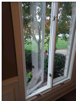
Loose hardware. Did not fully open.
