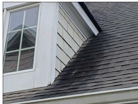
Inadequate gap between siding and shingles
