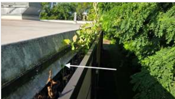
Membrane gutter overlap is loose at the flashing
