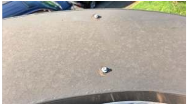
Deteriorated sealant
