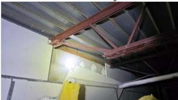
Steel roof trusses & metal roof sheathing
