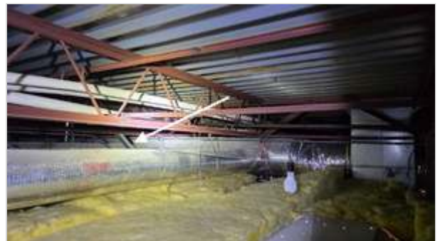
Support loading onto load bearing hallway walls
