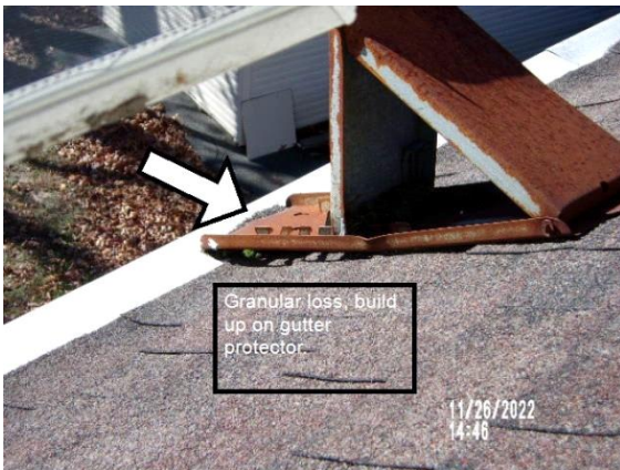
Roofing: Granular loss at bottom of old bracket.
