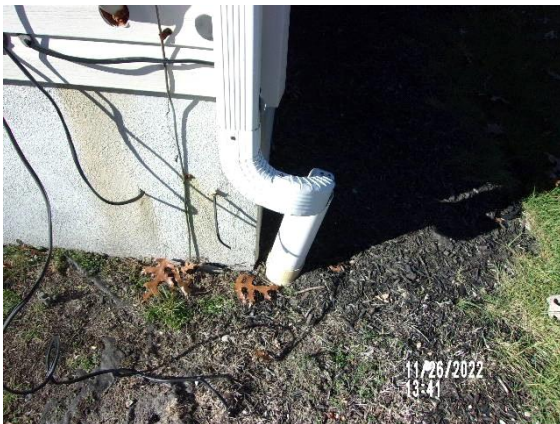
Gutters/Down Spouts: Emptying into underground piping.
