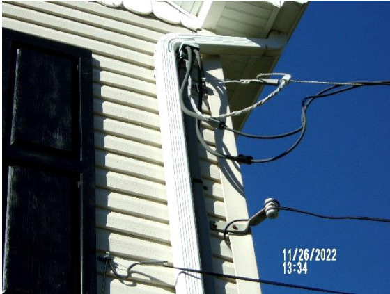
Electrical: Service drop - appears acceptable.
