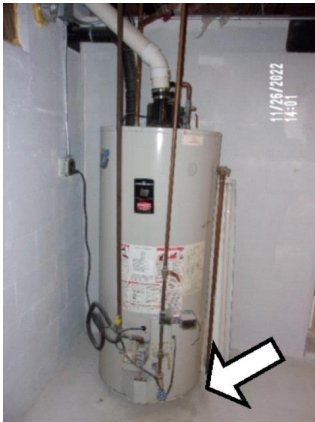
Water Heater: Missing drip/overflow pan.
