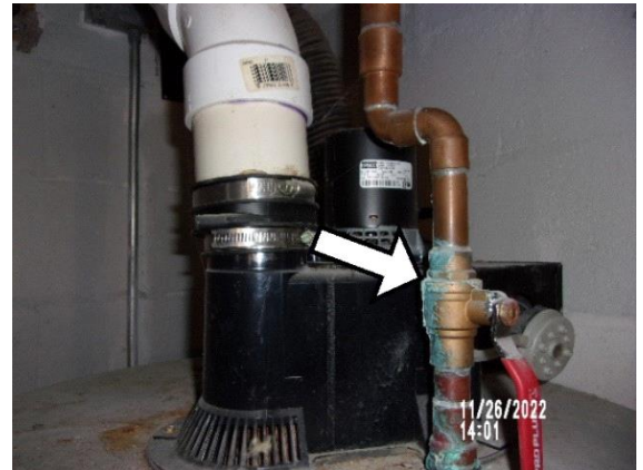
Water Heater: Corrosion on copper supply line.
