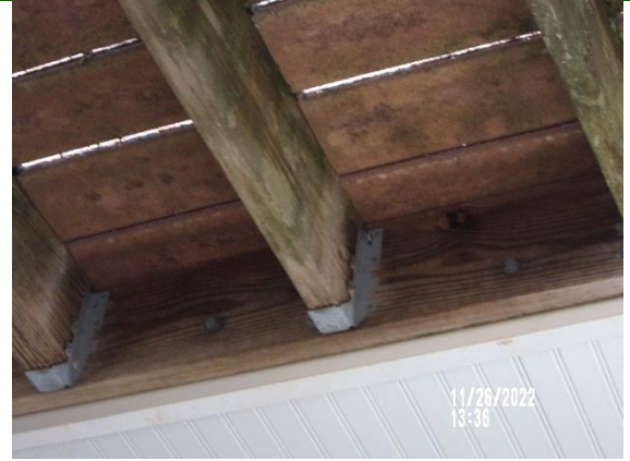
Decks / Balcony: Joist hangers in place.
