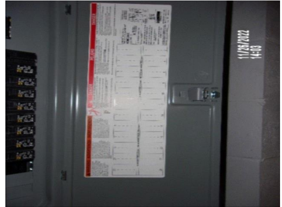
Electrical: Circuits not labeled
