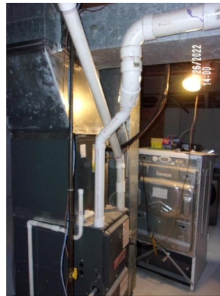
Plumbing: PVC vent piping.
