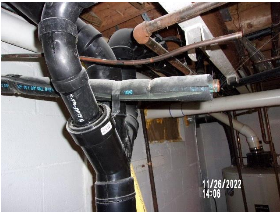
Plumbing: ABS waste piping.
