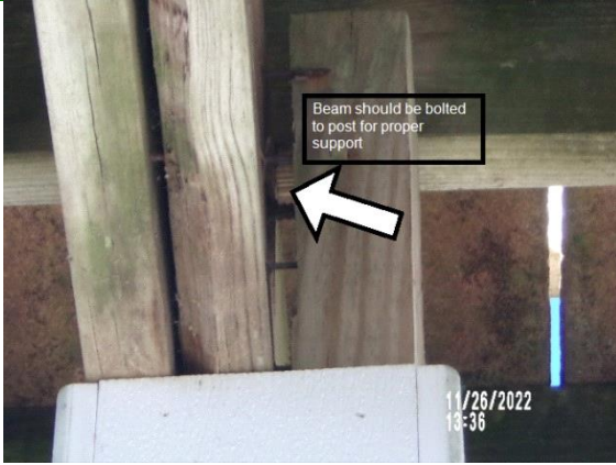
Decks / Balcony: Gap forming between beam and support post.
