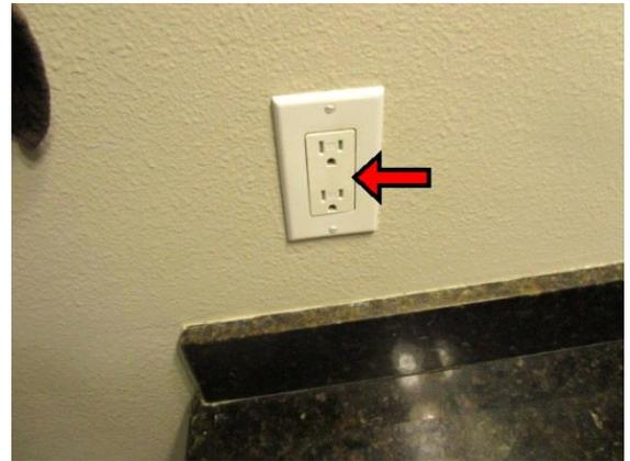
Bathroom Main Floor: Bathroom: GFCI circuitry not present
