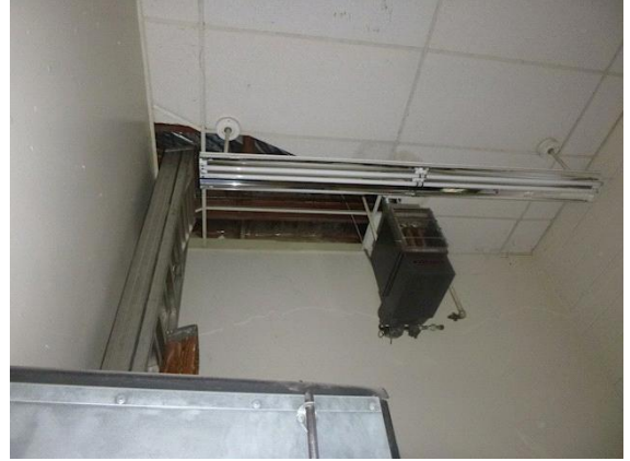
BREAKROOM/ STORAGE ROOM: The area heading to the loading dock has a heater that has been disconnected. Recommend capping the gas line.
