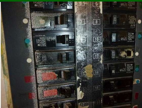
Electrical: Sub panel on the right hand side has a breaker that has been tripped and not reset.
