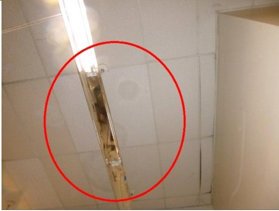
OFFICES/BACK OF HOUSE: Moisture stains on ceiling tiles.
