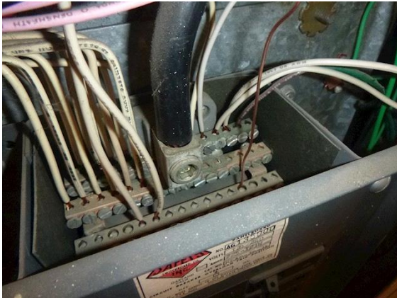
Electrical: Sub panel on the left has a mixed bus bar.
