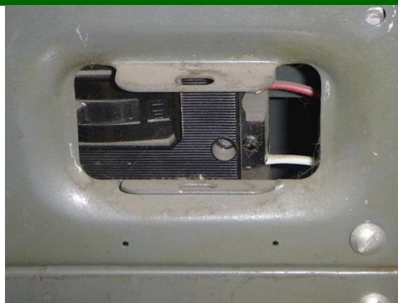
Electrical: At the main electrical panel there is a breaker that is misaligned and creates an open knockout in the dead front cover.
