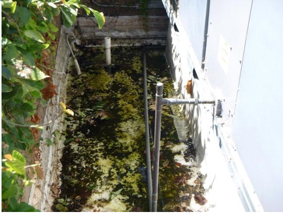
Roofing: Standing water on the roof near rooftop HVAC unit.
