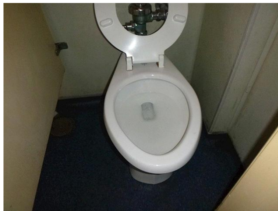
BATHROOM MENS: The right hand toilet is difficult to flush and may need a flush and fill kit.
