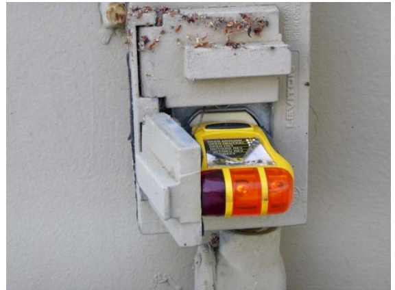
Exterior Surface: No power exterior electrical outlet.
