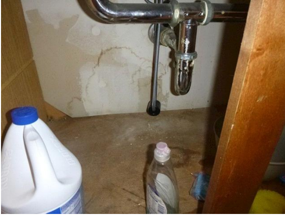
BREAKROOM/ STORAGE ROOM: Previous moisture under the sink in the break room.
