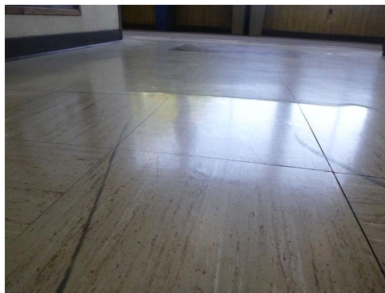
Floor/Slab: Areas of the floor in the PO box section has signs that the slab may be cracked and crowning in multiple locations
