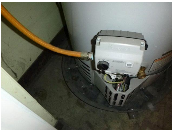
Water Heater: Missing drip pan.
