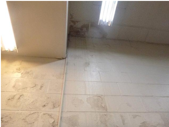
OFFICES/BACK OF HOUSE: Moisture stains on ceiling and walls.
