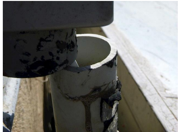
Roofing: Area of conduit damaged on the roof near rooftop AC unit.
