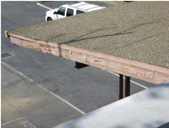
Exterior Surface: Loading dock has sign of moisture damage.
