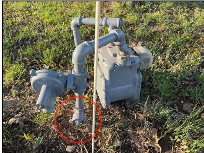
77. Gas meter/Main shut off
