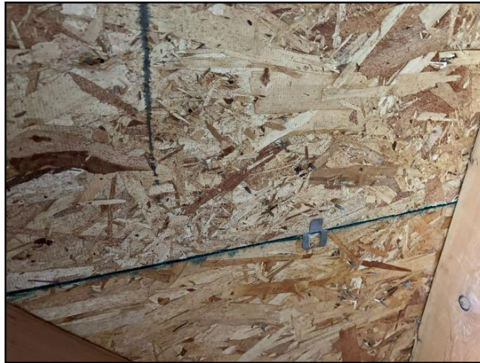
23. Oriented Strand Board (OSB) sheathing
