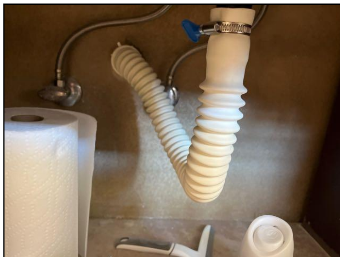
43. Nonstandard materials and patches
