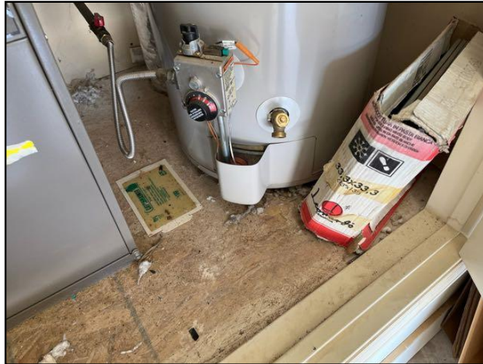
42. Safety pan and drain missing
