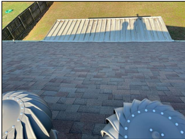
4. Asphalt shingles
