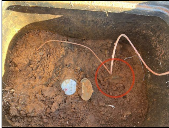
49. Meter/main shut off
