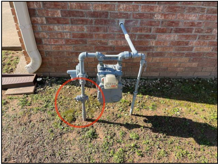
58. Gas meter/main shut off
