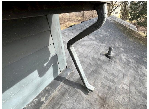
Gutters/Down Spouts: Gutter downspout has become detached.
