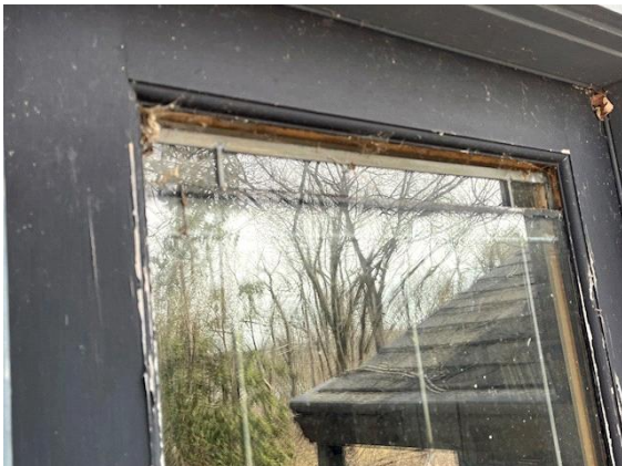
Exterior Doors: Balcony Door off Dining Room. Wood Frame is deteriorated and there is a Gap in the door between the Glass and the top of the frame.
