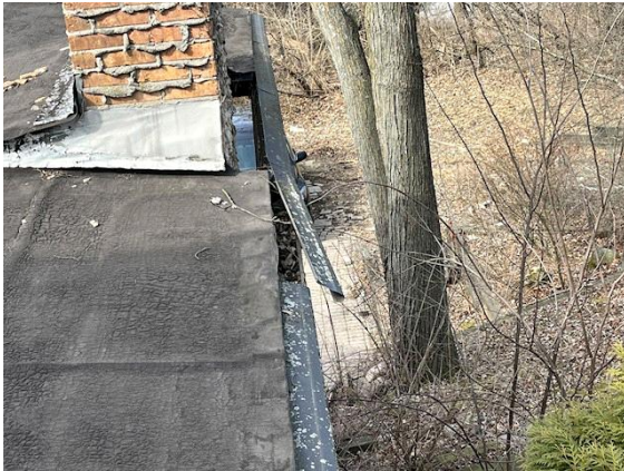
Gutters/Down Spouts: Gutter has become detached from fascia.
