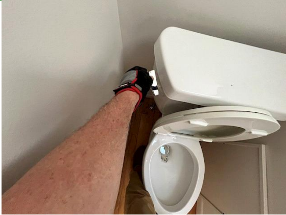
Bathroom - 2nd Floor: Flush handle disconnected
