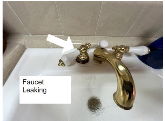
Bathroom - Full Guest Bathroom: Faucet Leaking
