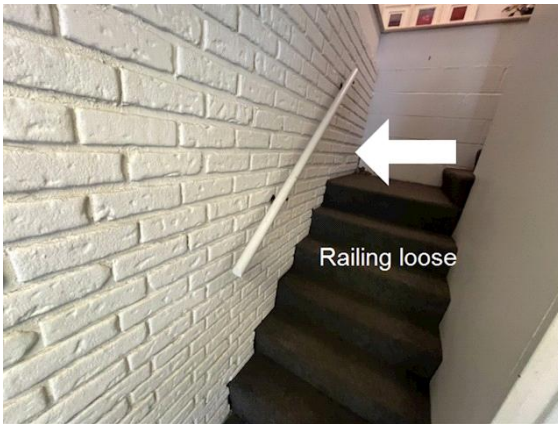
Stairs / Railings: Railing Loose
