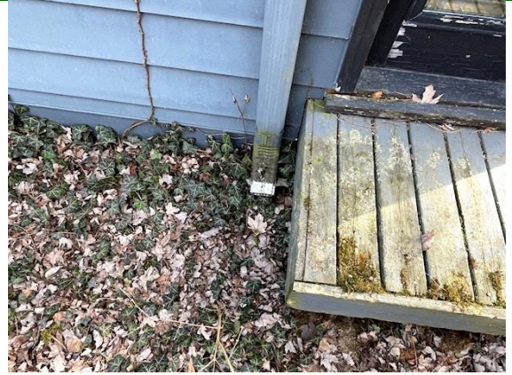
Gutters/Down Spouts: Missing Downspout extension to divert water away from the foundation.
