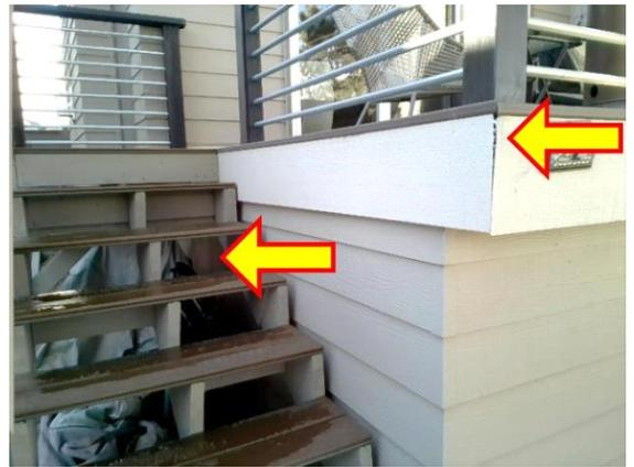
DECKS / BALCONY: Riser boards needed for steps; fascia board warped, caulk failed
