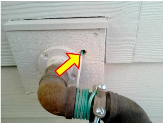
EXTERIOR SURFACE: open penetration, should be sealed, North side of home
