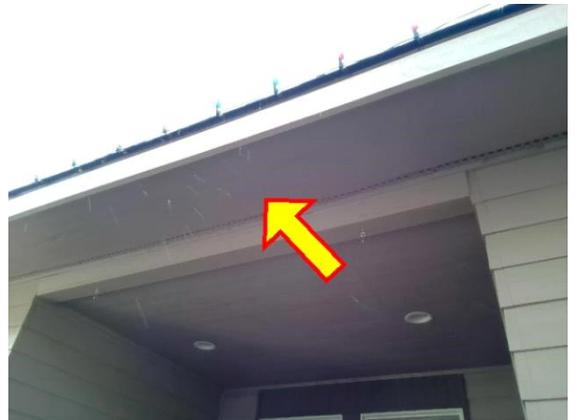
EXTERIOR SURFACE: soffit board bowed
