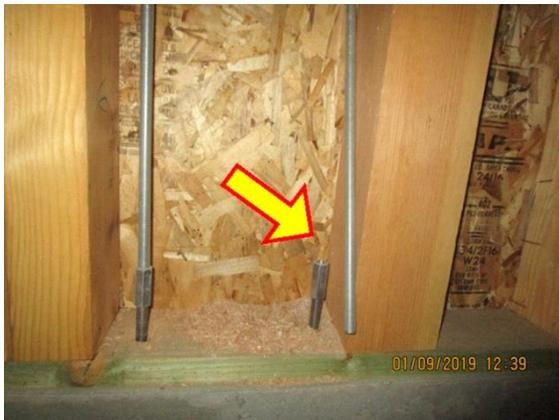
INTERIOR FOUNDATION: Location: East wall, to South side of home, anchor bolt unattached.
