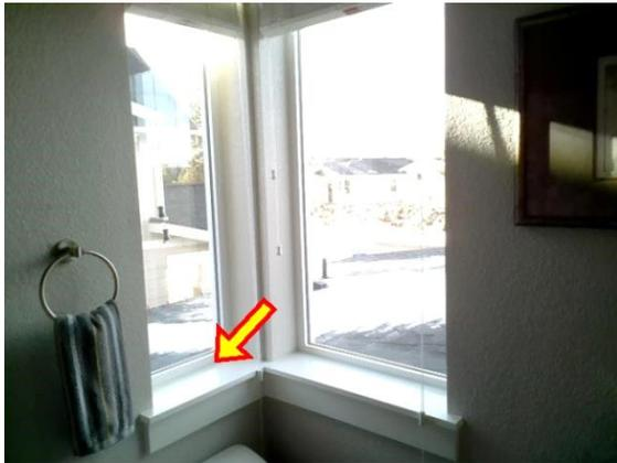
BATHROOM 2/ UP: caulking touch up needed here
