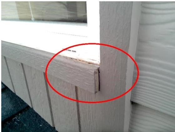
WINDOWS: SW 2nd story bathroom window, window trim board bowed, not attached correctly.
