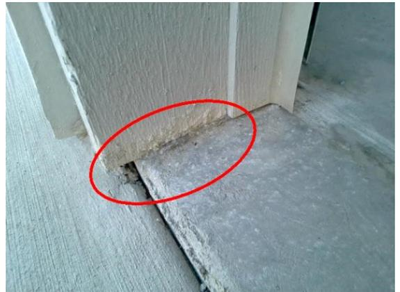
GARAGE/CARPORT: wood trim not cut back for water drainage, wood susceptible to water damage/rot
