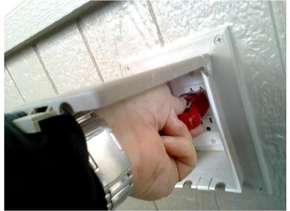
EXTERIOR SURFACE: Very difficult to plug tester into, South patio deck
