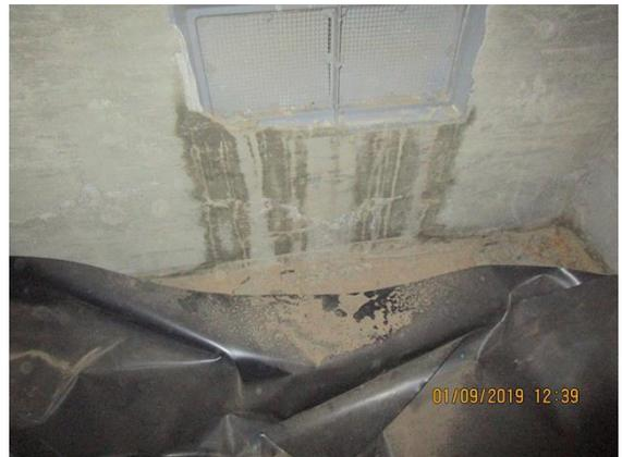
INTERIOR FOUNDATION: Evidence of previous water intrusion, South foundation wall vent
