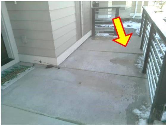
Walks / Steps: This section of concrete heaving/lifting
