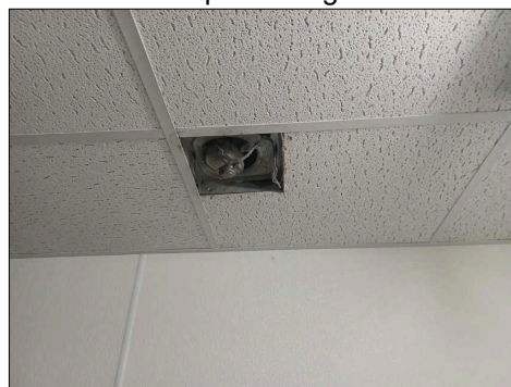
Inoperable bathroom exhaust fan
