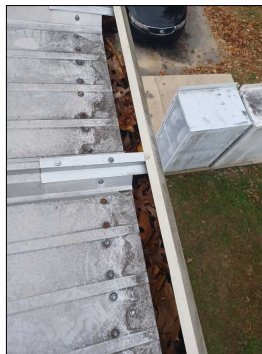
Debris in gutters
