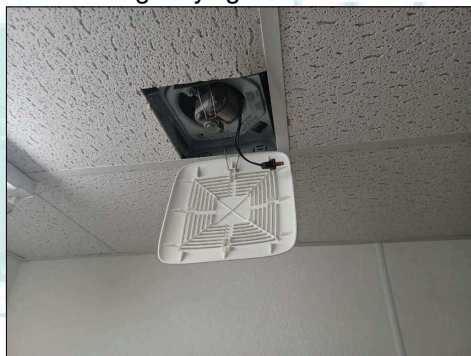
Inoperable bathroom exhaust fan
