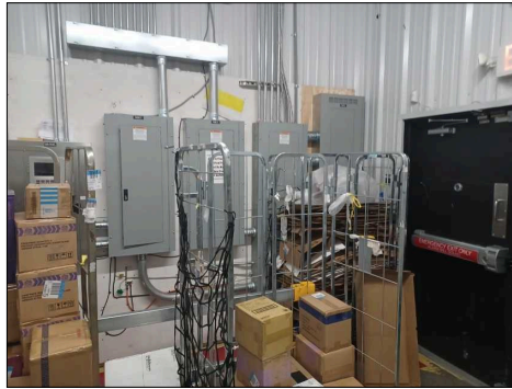
Breaker panels blocked
