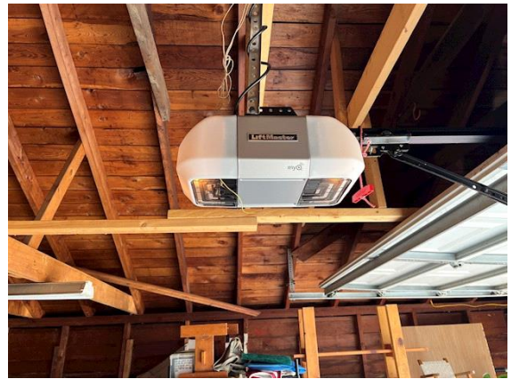
Overhead Garage Doors:
