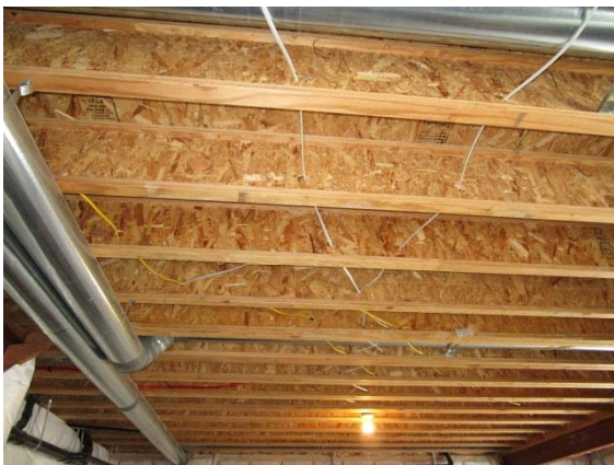
Under Floor Framing & Support:
