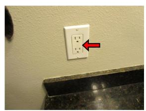
Bathroom Main Floor: Bathroom: GFCI circuitry not present
