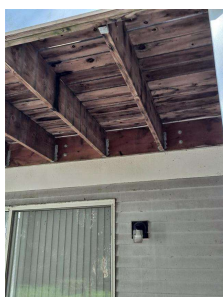
2.3 Item 2 (Picture) Proper lag bolts and joist hangers
