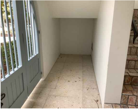
No storage below stairs
