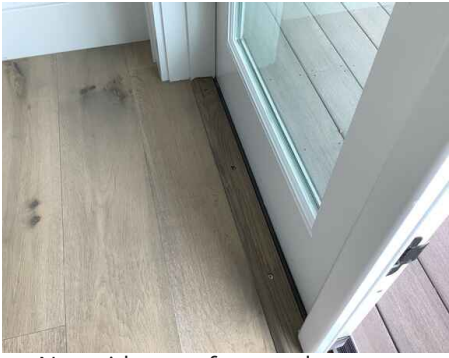
No evidence of water damage between interior and exterior door threshold
