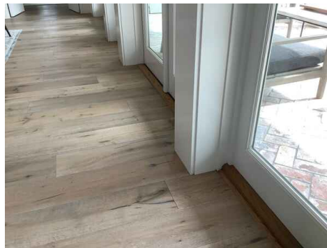
No evidence of water damage between interior and exterior door threshold
