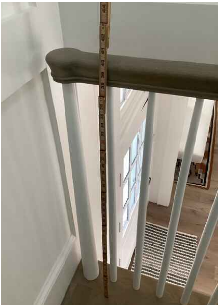
Guardrail also serves as a handrail, and is at least 34 and 38"
