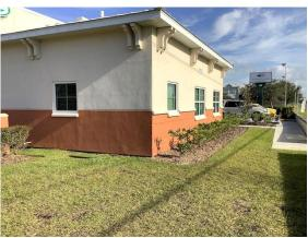
Grading / Drainage: View from rear left of property shows grading away from foundation.
