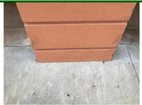
Exterior Surface: Inadequate clearance observed between the siding and exterior surfaces at the front bay areas.
