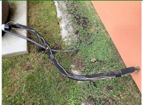
Cooling: Refrigerant lines appear properly insulated
