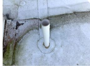
Roofing: Plumbing vent - missing screen
