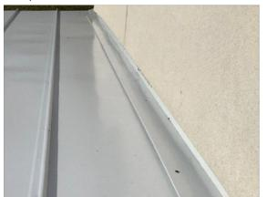
Proper intersection clearance where wall meets roof
