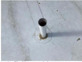
Roofing: Plumbing vent - missing screen
