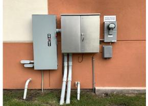
Electrical: Underground service, TECO meter, and electrical disconnect located at left exterior of building.
