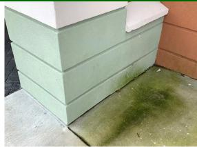
Exterior Surface: Pressure wash for mildew from drainage from metal roof. Also low clearance.
