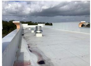
Roofing: TPO roofing over garage bays
