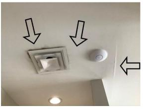
What appears to be microbial growth, water stains, and sagging in office ceiling from overfilled air handler pan above
