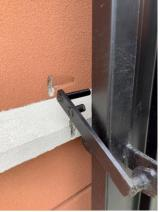
Exterior Surface: Wall damage from dumpster enclosure door
