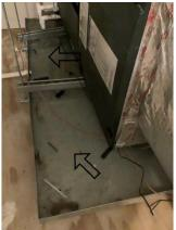
Cooling: Pan filled with water and overflowing in attic
