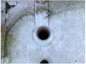
Roofing: Plumbing vent - missing screen
