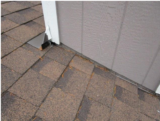
Chimney: chimney flashing
