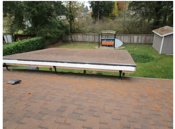
Patio: Patio roof
