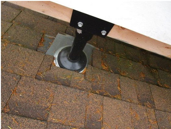
Patio: Patio roof support
