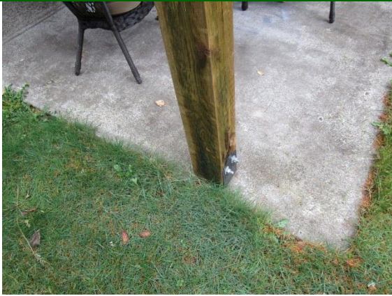
Patio: Patio roof footing
