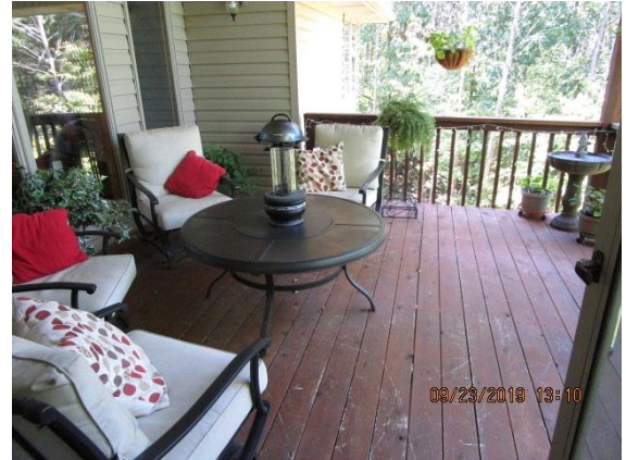
Decks / Balcony: Upper Deck
