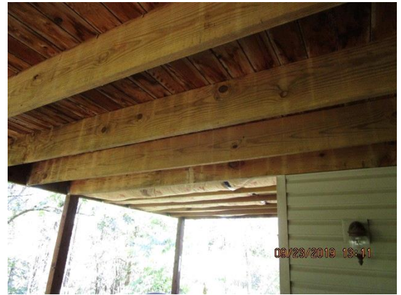
Grading / Drainage: Deck in Back of Home
