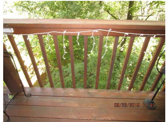
Grading / Drainage: Off Lower Deck
