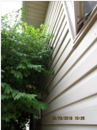
Grading / Drainage: East Side of House
