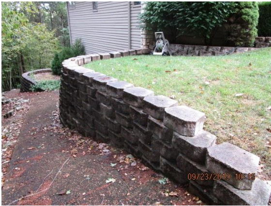
Grading / Drainage: West Side of Home
