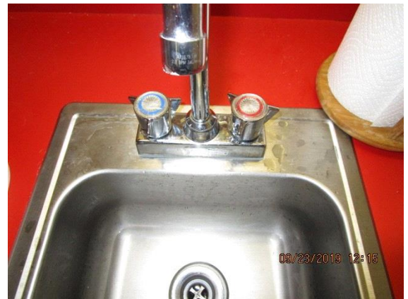
Basement: Basement Sink
