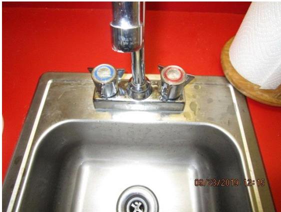
BASEMENT: Basement Sink
