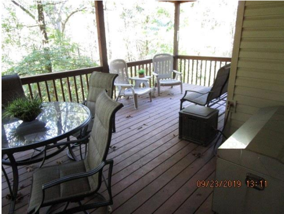
Decks / Balcony: Lower Deck
