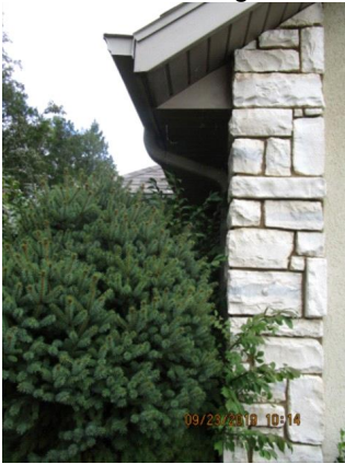
EXTERIOR SURFACE: Bushes against Synthetic Stucco
