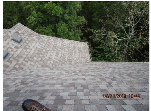
Roofing: Roof towards back of lot
