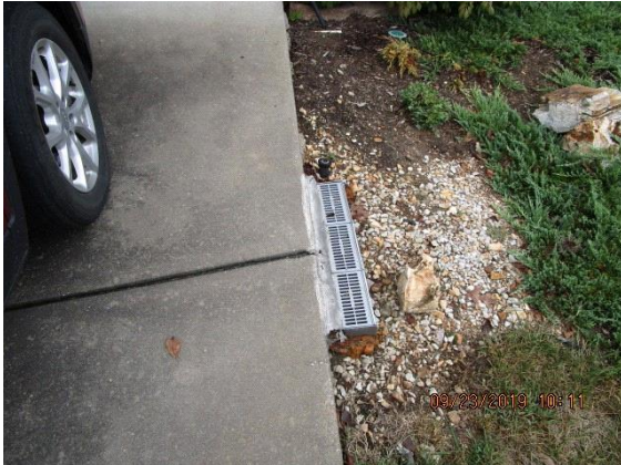
Driveway: Driveway drain
