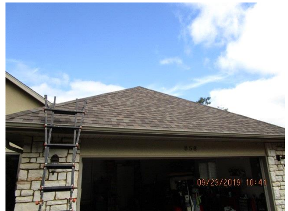
Roofing: Garage Front Roof
