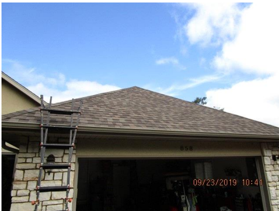
Roofing: Garage Roof Front
