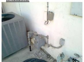
COOLING: No equipment disconnect within visible range.
