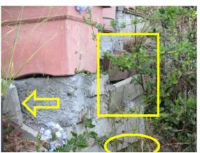
RETAINING WALLS (CONT): Arrow indicated form boards left in place, Circle indicates block not sitting on footing. Square shows form wood either left in place or used for support.
