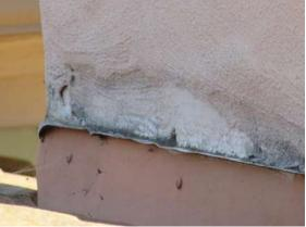
Chimney: Water damage at base of chimney at flashing.
