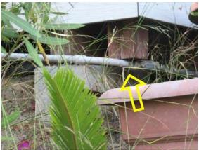
Retaining Walls (cont): Wood support post for deck resting on grey PVC pipe for support.
