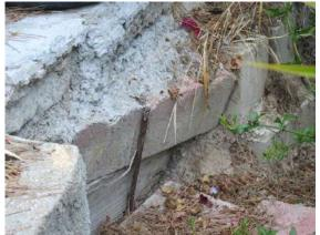
Retaining Walls (cont 2): Example of poor and unconventional workmanship encompassing the entire retaining wall structure.
