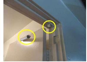
Garage Pedestrian Door into House: Automatic door closure disconnected.
