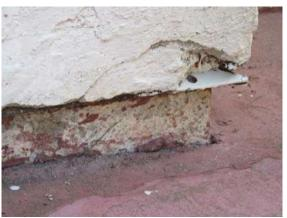
FOUNDATION APRON: Evidence of water damage at footing and stucco intersection with damaged & rusted drip screed. Also observed patching of flatwork next to house.
