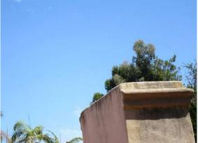
CHIMNEY: No rain cap/spark arrestor visible at the time of the inspection.
