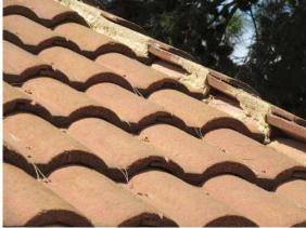
Roofing (cont 2): Unconventional repairs at location of previously suspected leak.
