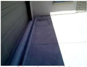
Driveway: Driveway berm/trench drain installation.
