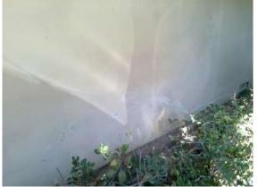
EXTERIOR SURFACE: Evidence of water staining and/or patching, potentially caused by irrigation. May warrant further investigation to resolve issue.
