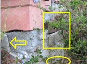
Retaining Walls (cont): Arrow indicated form boards left in place, Circle indicates block not sitting on footing. Square shows form wood either left in place or used for support.
