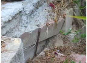
RETAINING WALLS (CONT 2): Example of poor and unconventional workmanship encompassing the entire retaining wall structure. MARGINAL
