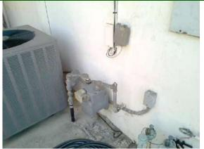
Cooling: No equipment disconnect within visible range.
