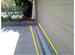
Foundation Apron: Installation of concrete berm & trench drain indicate possible past water intrusion issues.
