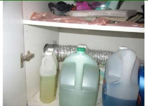
Laundry Facilities: Dryer vent snakes through back wall into cabinet, then garage, then under water heater to the outside.
