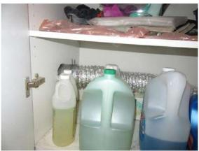
LAUNDRY FACILITIES: Dryer vent snakes through back wall into cabinet, then garage, then under water heater to the outside.
