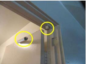
GARAGE PEDESTRIAN DOOR INTO HOUSE: Automatic door closure disconnected.
