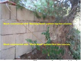
RETAINING WALLS: The use of various block construction patterns within the same wall indicates the likelihood that non or poor construction knowledge was used.
