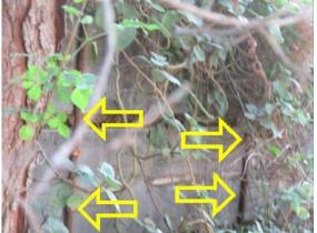
Retaining Walls: #3 or #4 rebar used on outside of wall for unknown reason.
