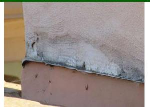
CHIMNEY: Water damage at base of chimney at flashing.
