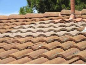
Roofing: Lighter tile indicate past repairs.
