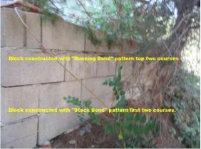
Retaining Walls: The use of various block construction patterns within the same wall indicates the likelihood that non or poor construction knowledge was used.
