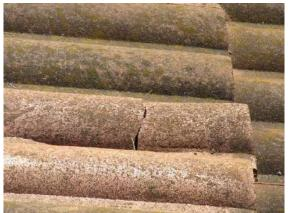
ROOFING (CONT 2): Some cracked tiles observed.
