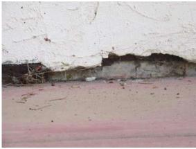
Exterior Surface: Water damage and rusty drip screed.
