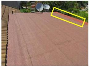
FLAT ROOF OVER SUNROOM: Location of previous roof repairs at location of suspected leaks.
