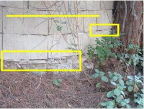
Retaining Walls: Appears to have been intentionally built out of level for unknown reasons. Boxes indicate examples of unconventional construction methods with the use of filler material at wall joints.
