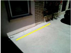
Driveway: Concrete repair potentially in conjunction with installation of driveway trench drain.
