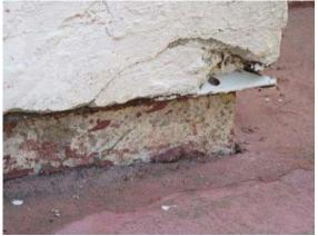
Foundation Apron: Evidence of water damage at footing and stucco intersection with damaged & rusted drip screed. Also observed patching of flatwork next to house.
