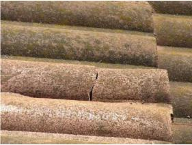
Roofing (cont 2): Some cracked tiles observed.
