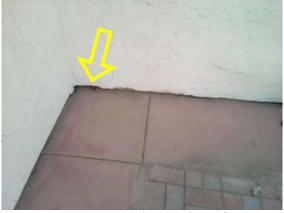
FOUNDATION APRON: Observation of concrete apron around structure. Arrow indicates potential past water damage.
