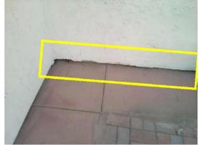
Exterior Surface: Water damage and rusty drip screed.
