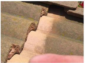
ROOFING (CONT): Lighter coloration of tile indicates areas where tiles have come loose.
