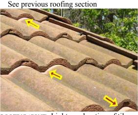
ROOFING (CONT): Lighter coloration of tile indicates areas where tiles have come loose.
