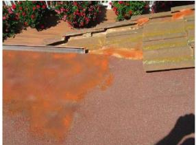
FLAT ROOF OVER SUNROOM: Evidence of unconventional repair methods with unknown materials indicates previous leaks.
