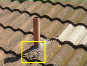
Roofing (cont 2): Unconventional repairs at location of previously suspected leak.
