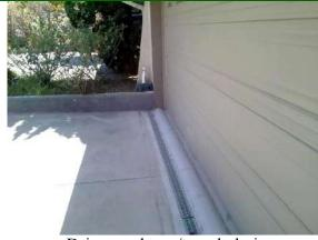
Driveway: Driveway berm/trench drain installation.
