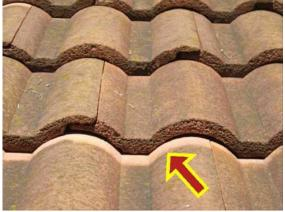
Roofing: Lighter tan line indicates tile have slipped down about an inch within the last few years.
