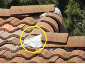
Roofing (cont): Unconventional repairs at location of previously suspected leak.
