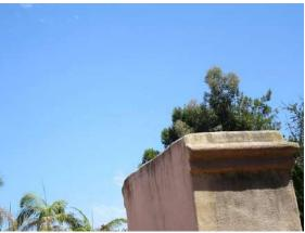
Chimney: No rain cap/spark arrestor visible at the time of the inspection.
