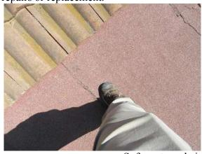
FLAT ROOF OVER SUNROOM: Soft spots and air pockets observed under rolled roofing indicating no adhesion or the adhesion has failed.
