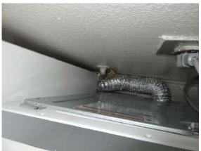
Laundry Facilities: Dryer vent snakes through back wall into cabinet, then garage, then under water heater to the outside.
