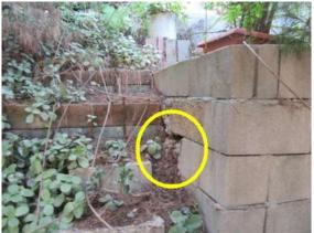
RETAINING WALLS: Evidence of possible lack of footings at retaining wall.
