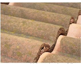
ROOFING (CONT): Lighter coloration of tile indicates areas where tiles have come loose.
