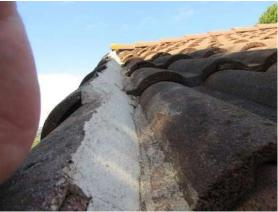
ROOFING (CONT): Unconventional repairs at location of previously suspected leak.
