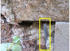
Retaining Walls (cont): Metal concrete form stake used in an unconventional manner.
