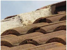
Roofing: Unconventional roof patch at location of previous leak.
