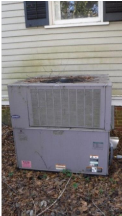
Cooling- Main House: Gas Pack
