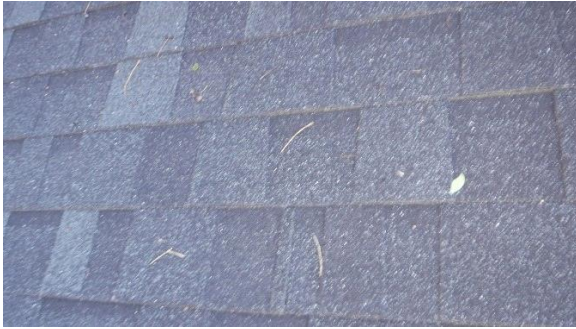
Roofing: Shingles- close up
