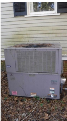
HEATING- MAIN HOUSE: Gas Pack- does not operate
