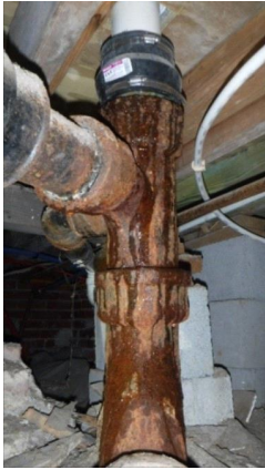
Plumbing: Drain line leak in crawl space
