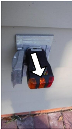
EXTERIOR SURFACE: Exterior electrical outlet- open ground connection
