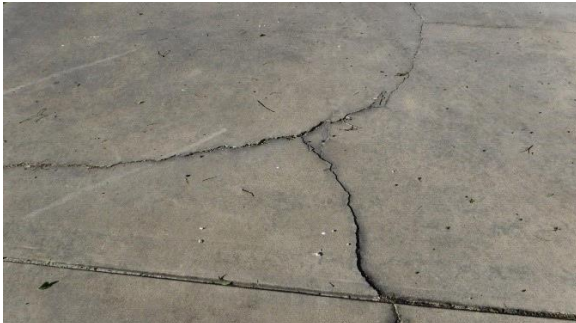
Driveway: Cracks in concrete
