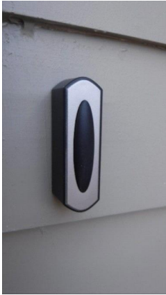
Ext Surface Misc Electrical Item: Rear door bell button
