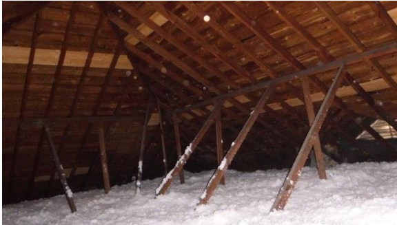
Attic Insulation: Blown insulation over main house
