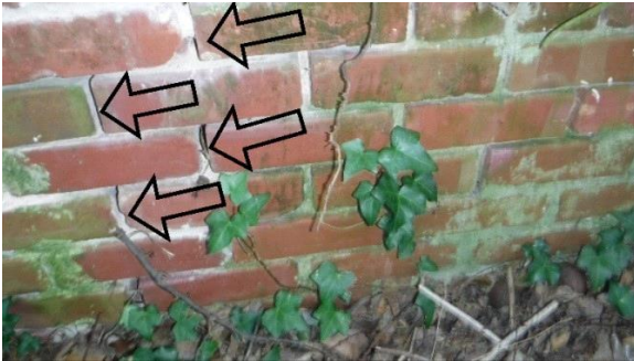
EXTERIOR FOUNDATION: Loose/missing mortar between bricks
