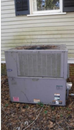
Heating- Main house: Gas Pack- does not operate
