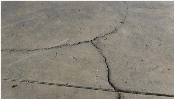
DRIVEWAY: Cracks in concrete
