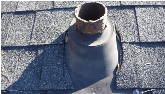
Plumbing vent boot Flashings:
