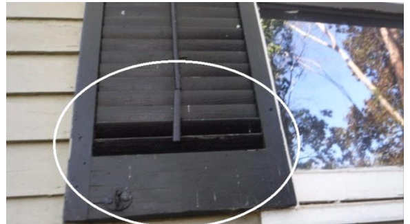
WINDOWS: Broken/ deteriorating window shutters
