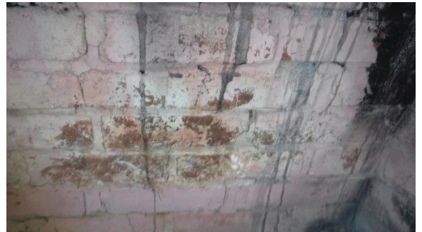
FIREPLACE: Loose/ missing mortar between bricks
