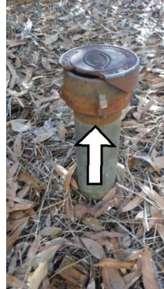
Heating- Main house: Underground oil tank
