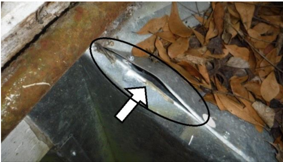
HVAC DISTRIBUTION: Exterior ductwork shroud
