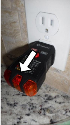
KITCHEN: Countertop outlets- open ground connections
