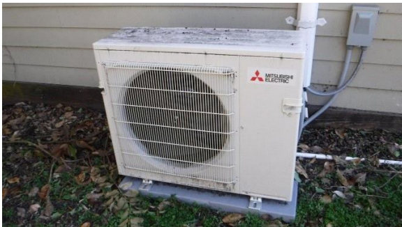
Heating- Rear additions: Mini Split
