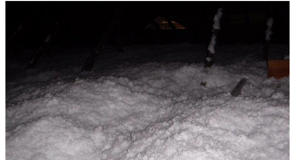
Attic Insulation: Blown insulation over main house
