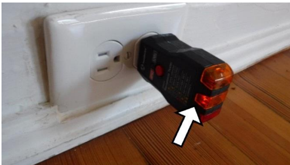
Living room: Electrical outlets- have open ground connections
