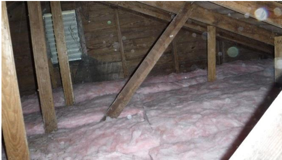
Attic Insulation: Batt insulation over bonus room
