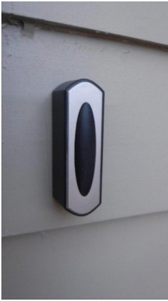
EXT SURFACE MISC ELECTRICAL ITEM: Rear door bell button
