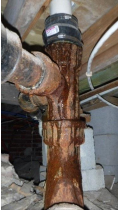
PLUMBING: Drain line leak in crawl space
