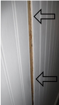
Rear bonus room: Loose wall paneling
