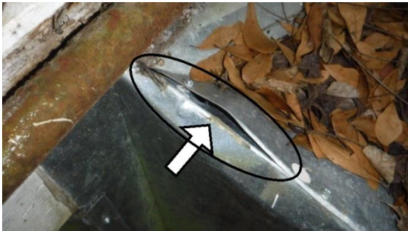
HVAC Distribution: Exterior ductwork shroud
