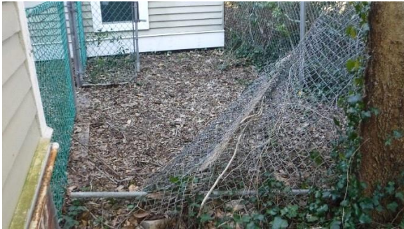
Fences / Gates: Broken fencing- right side of house
