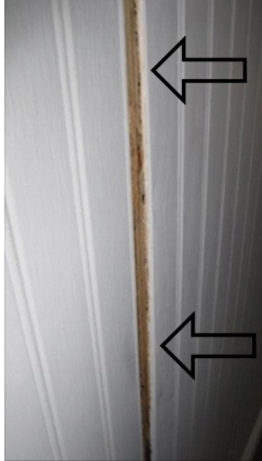
REAR BONUS ROOM: Loose wall paneling
