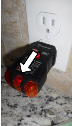
Kitchen: Countertop outlets- open ground connections
