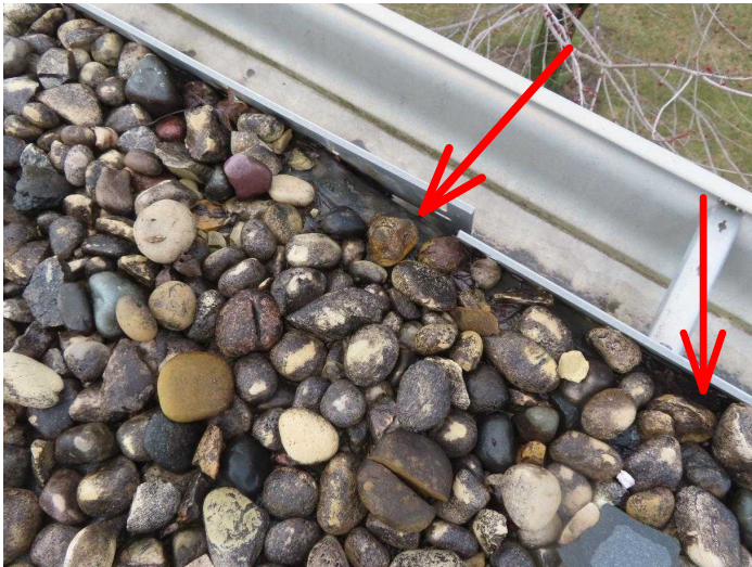
West Flashing To Gutter Transition
