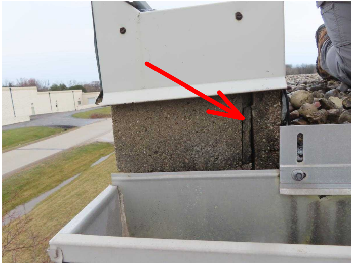
Tuck Point Maintenance Required
