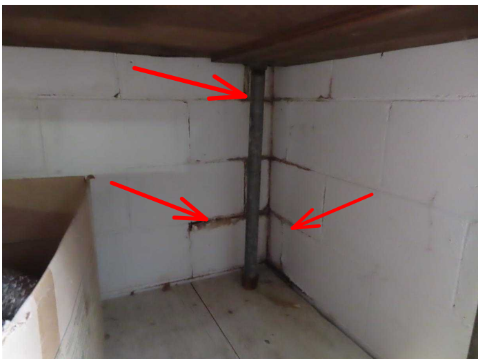
NW Wall Water Staining
