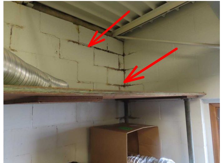
NW Wall Water Staining
