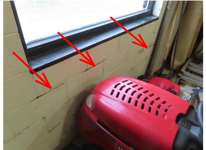
West Wall Water Staining
