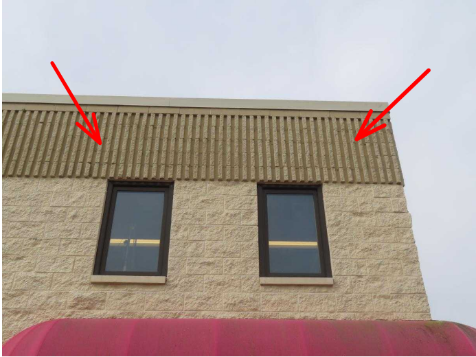
NE Wall Exterior Water Staining
