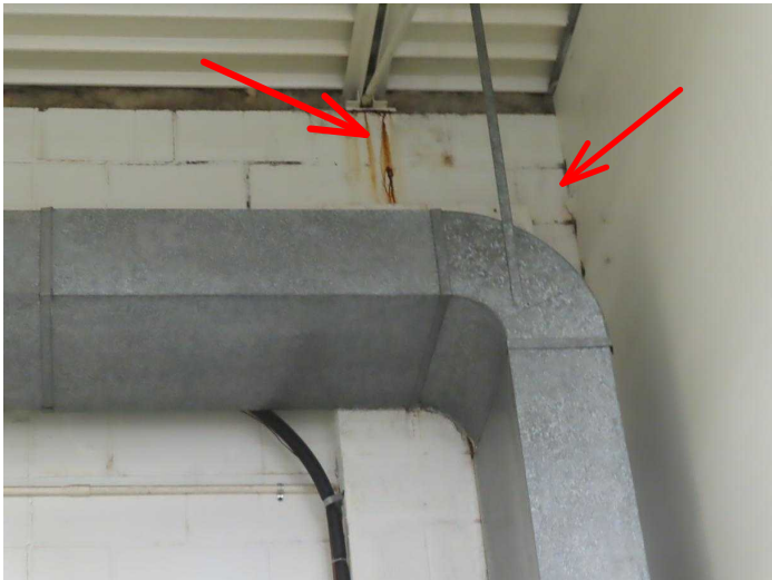
West Wall Water Staining
