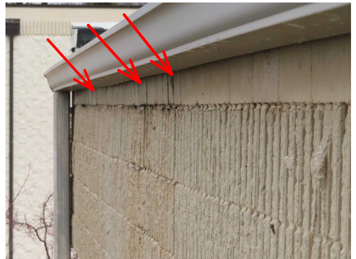
Possible Water Behind Gutter
