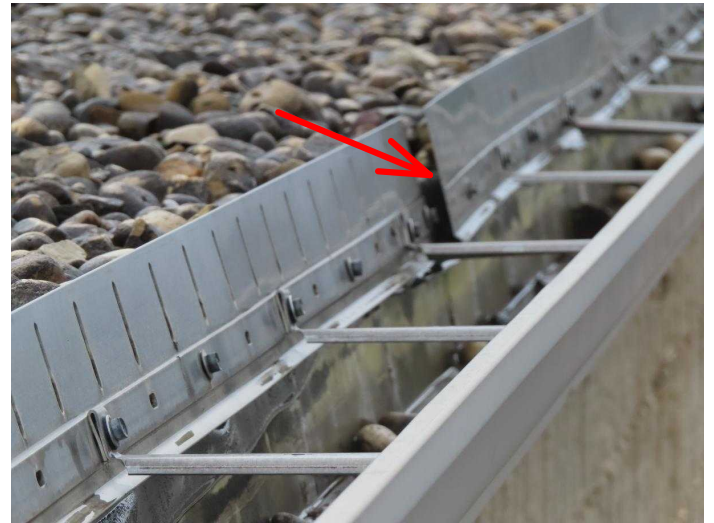
Possible Water Behind Gutter
