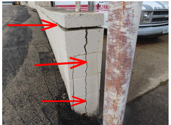
Loading Dock Wall Damage
