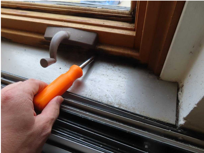
East Wall Dry Rotted Window
