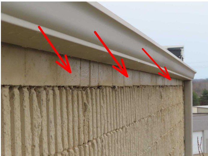
Possible Water Behind Gutter
