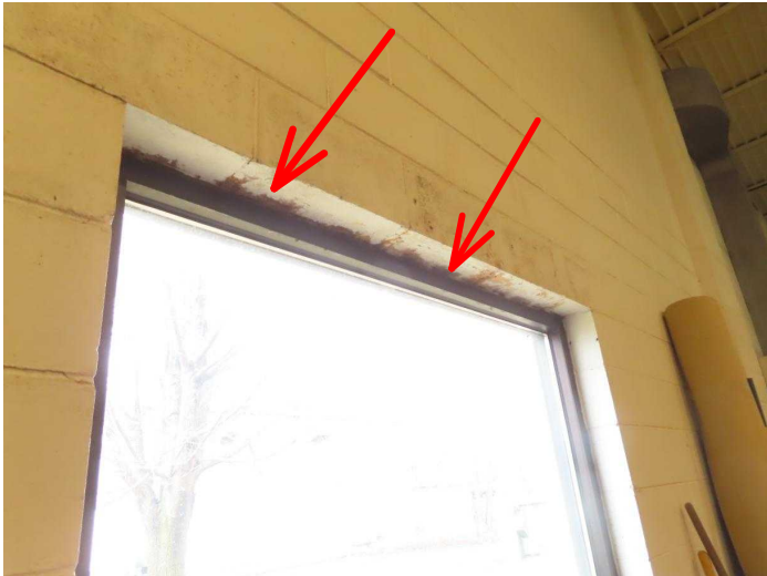
South Wall Water Staining
