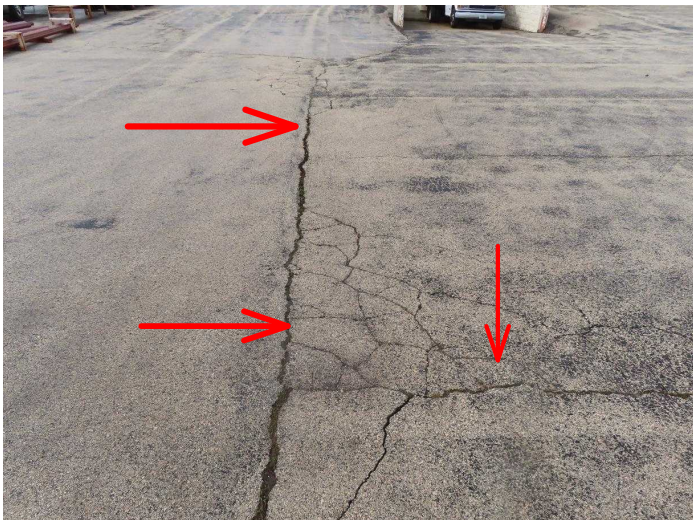
Cracks And Alligatoring
