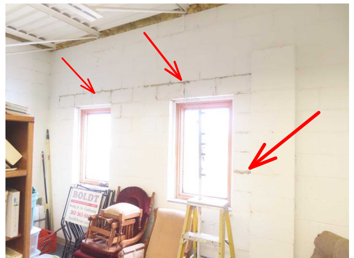
East Wall Water Staining
