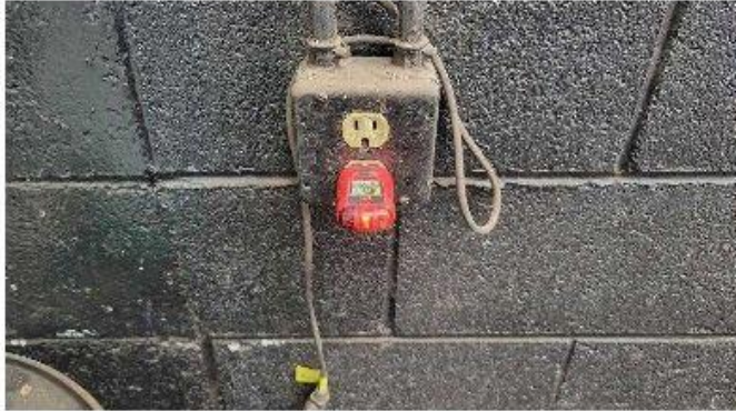
South Shop Outlet Open Ground
