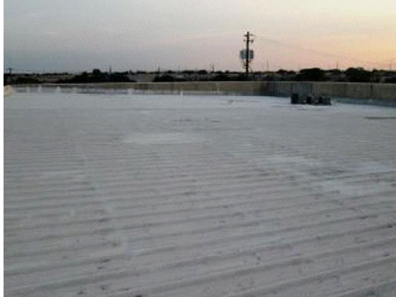
Roofing: Overall view of roof with spray-on elastomeric coating.
