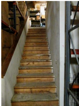
Stairs / Railings: Warehouse stairs to upper level.
