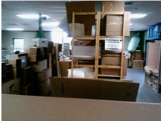
Heating: Obstructions preventing inspection of furnace.
