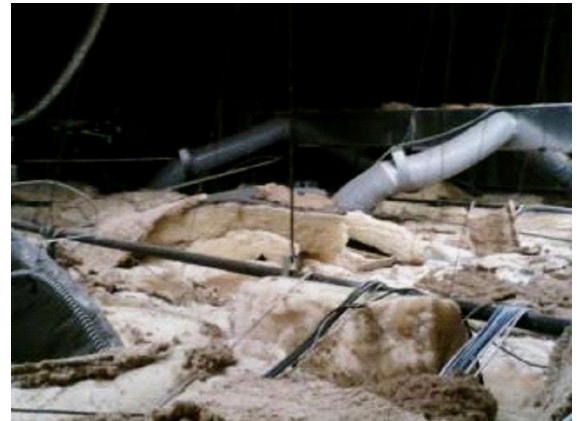
Insulation: Blanket insulation over ceiling grid in office.
