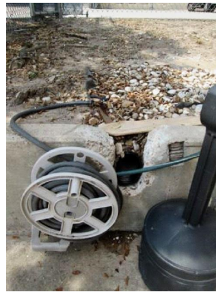
Grading / Drainage: Termination of perforated drain pipe.
