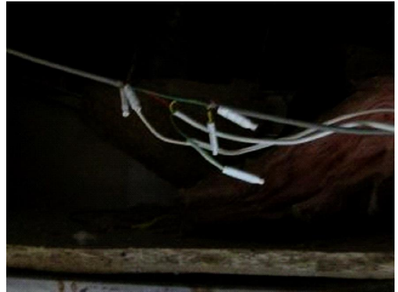
Attic Electrical: Open splices above ceiling grid.
