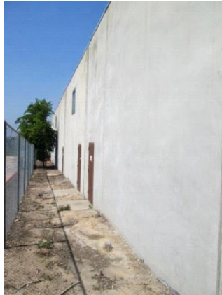
Grading / Drainage: Positive slope on east (back) wall.
