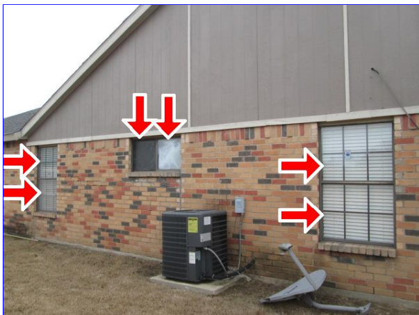
I. Item 5 6 on right wall
