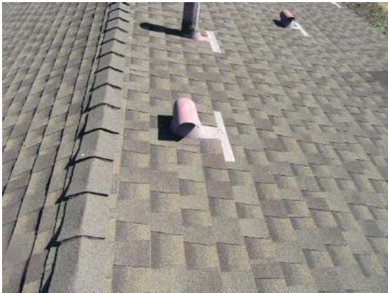
Flashing/Valleys: Typical flashing
