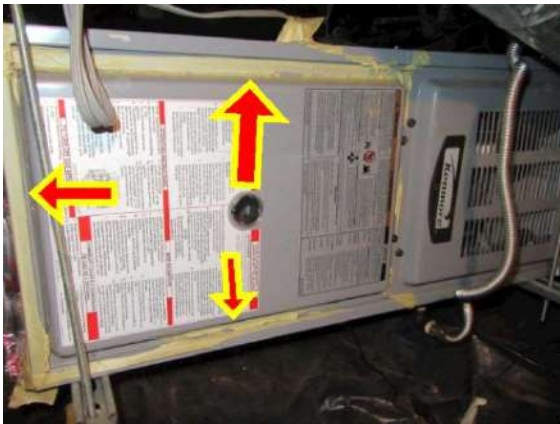
Heating: unit taped shut.
