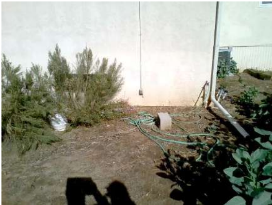
Foundation: Foundation not visible at slab-on-grade room addition.
