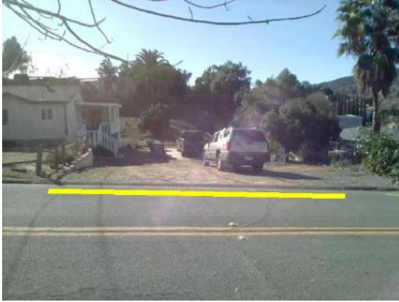
Driveway: Looking at driveway from street. Yellow line indicated asphalt berm between road and dirt driveway which will divert water towards bottom of street rather than homeowner's driveway.
