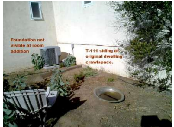
Foundation: See notes on photo.
