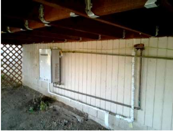
Decks / Balcony: Proper hangers installed at bottom of west side deck. Tankless water heater located beneath west side deck.
