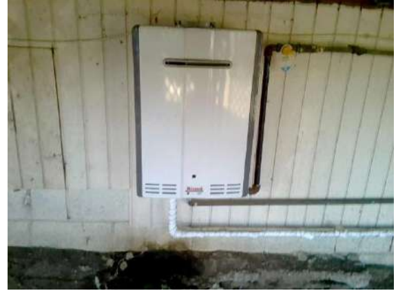
Water Heater: Tankless water heater located under west deck.
