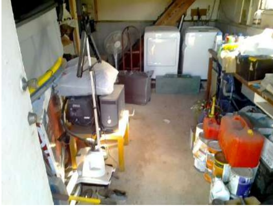
Floor/Slab: Concrete slab located in basement below room addition.
