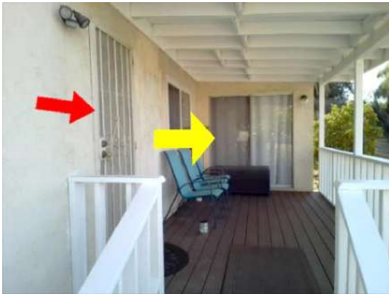
Exterior Doors: Red arrow id door to kitchen and yellow arrow is pointing to master bedroom slider.
