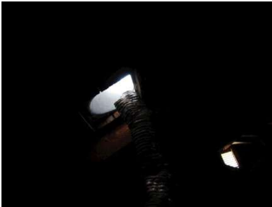
Attic Ventilation: Restroom ventilation does not exit through roof but rather terminates in attic near ventilation turbine.
