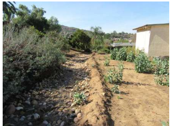
Grading / Drainage: Rear culvert running across rear of property.
