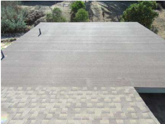
Roofing: Flat roof located over room addition at master bedroom.
