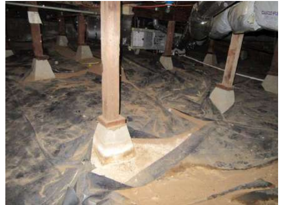
UNDER FLOOR FRAMING & SUPPORT: No connection between concrete pier and wood posts. (typical)
