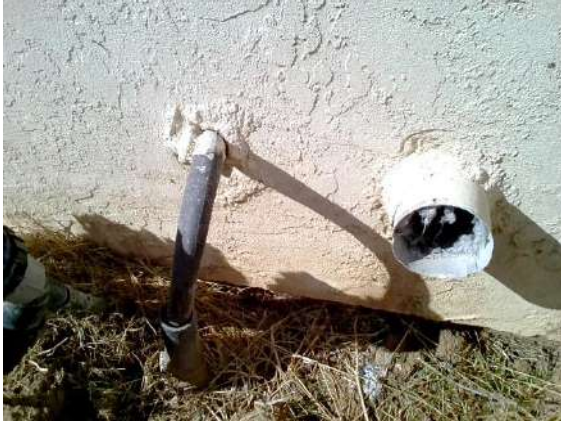
Laundry Facilities: Dryer vent termination point does not have a screen or flapper to keep animals from entering. Recommend installing one.
