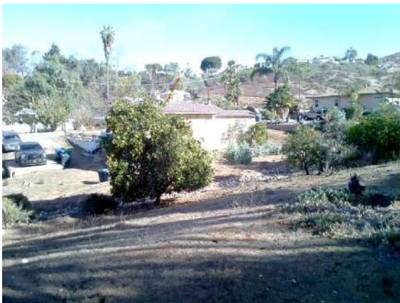
Grading / Drainage: Negative slope looking from back of slope towards front of home.
