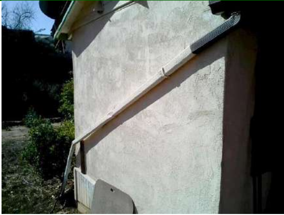
Gutters/Down Spouts: Typical gutter
