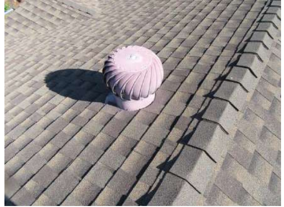
Flashing/Valleys: Attic ventilator
