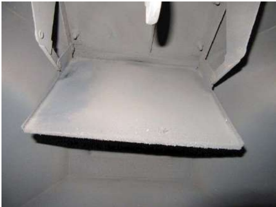
Fireplace/Stove: Did not appear to have the stopper bracket placed on damper to insure damper is never fully closed.
