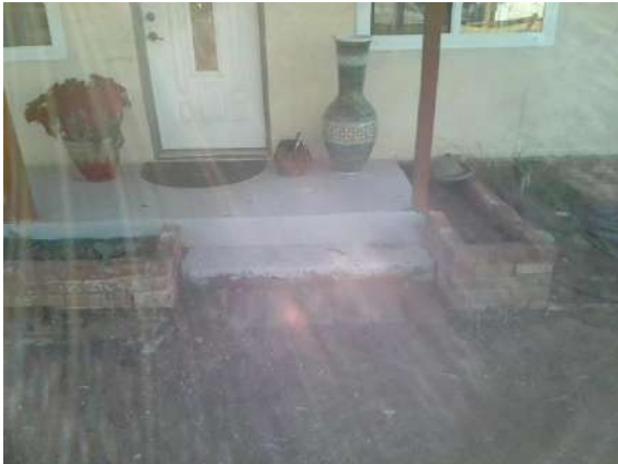
Walks / Steps: Front porch concrete step.
