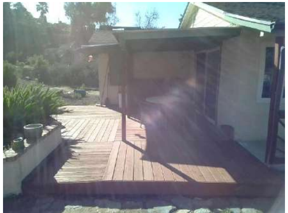
Decks / Balcony: East side wood deck.
