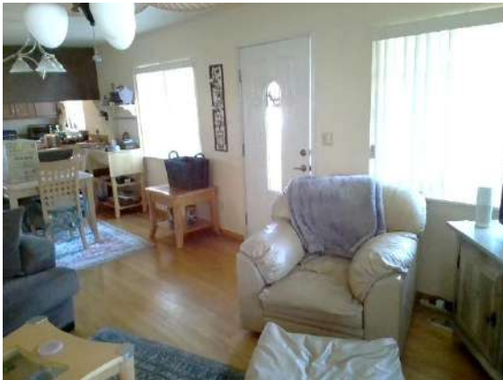
Floor/Slab: Furniture and rugs covered most of common area floors which limits inspection at time of inspection. No issues were observed in the areas that were inspected.
