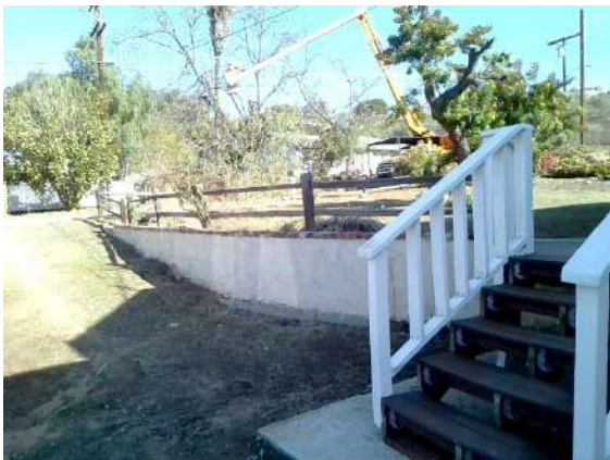
Retaining Walls: Block retaining wall between driveway and front yard.
