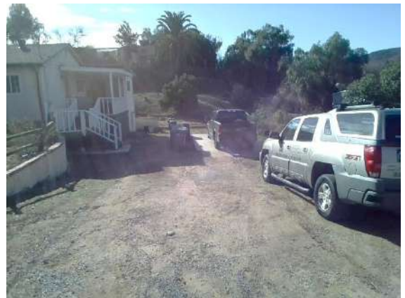
Grading / Drainage: Negative grade from street to old garage concrete pad. Water is directed to riprap culvert at rear of house.
