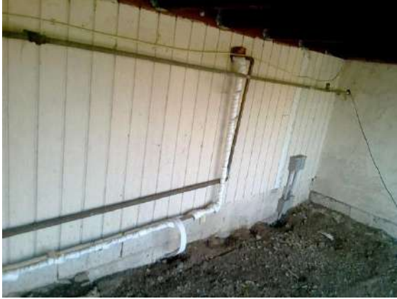
Water Heater: Water piping under west deck to tankless water heater.
