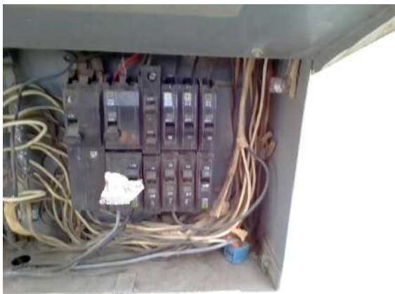
ELECTRICAL: No dead man cover on main electrical distribution panel.
