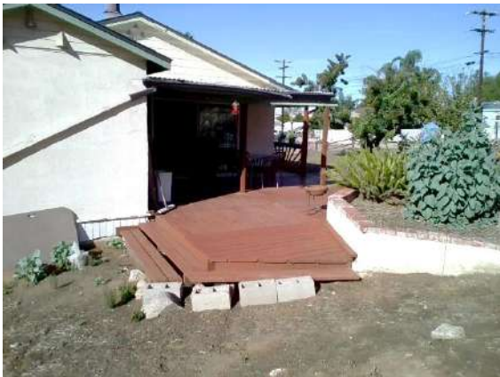
Decks / Balcony: East side wood deck.
