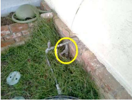
Plumbing: water shut-off
