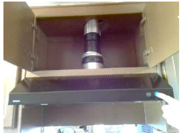
Kitchen: Exhaust hood over stove piped directly to attic. Recommend the pipe be continued through the roof by a licensed, professional roofer.
