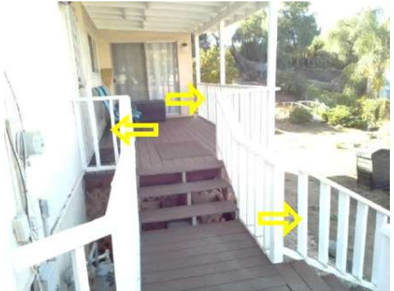
Decks / Balcony: Handrail spacing wider than 4". Recommend repairs which may include removing and replacing or adding a baluster between each existing balusters.
