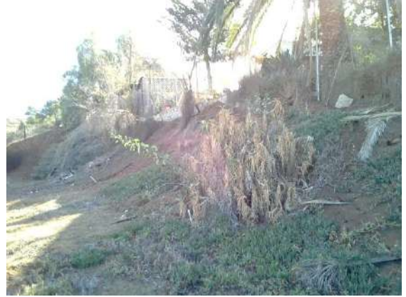
Grading / Drainage: Slope at back of property.
