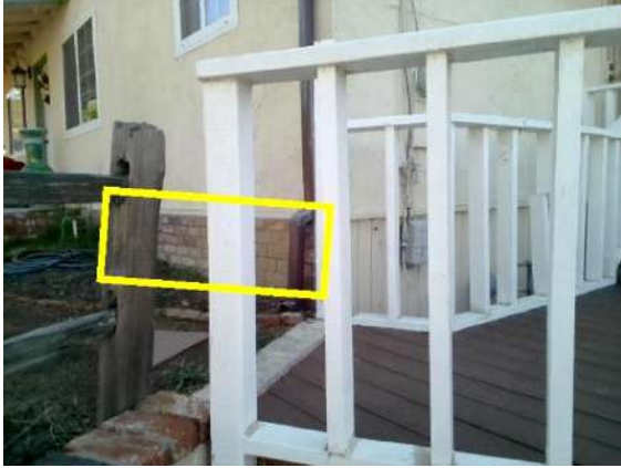
Foundation: Brick facade in front of crawlspace foundation.
