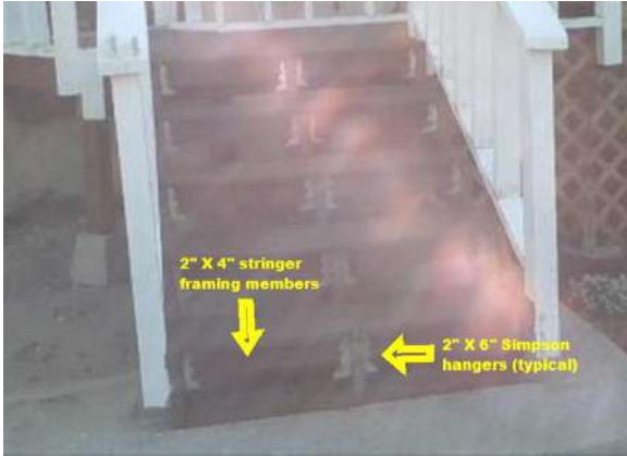
Walks / Steps: Incorrect hangers applied to stair open risers/horizontal supports.
