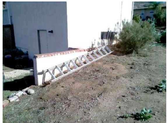
Retaining Walls: Partial stucco faced masonry wall about 48" which acts as a retaining wall for about 12" of rear yard.
