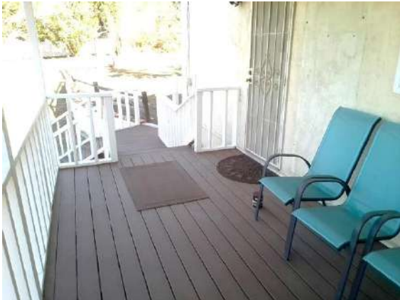
Decks / Balcony: West side composite decking planks.
