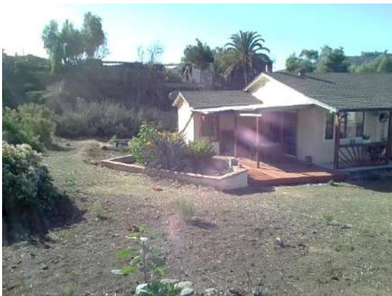
Grading / Drainage: East side of yard.
