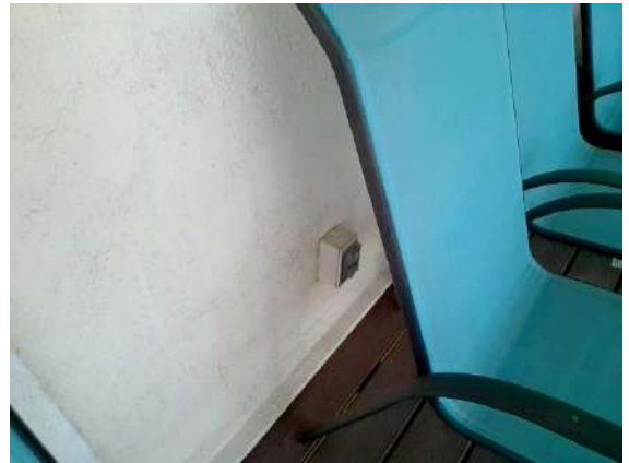
Exterior Surface: Exterior electrical outlet located on west deck.
