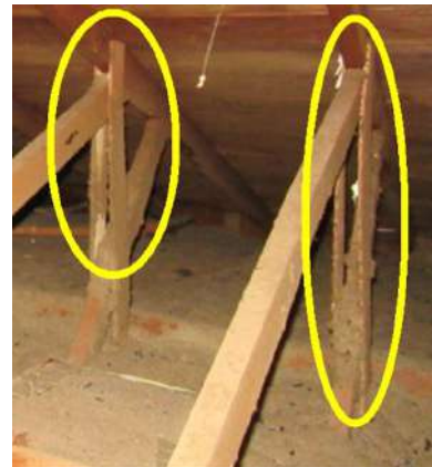
Attic Framing/Sheathing: Vertical white pieces are particleboard repairs/added support to rafters and need to be reviewed by a structural engineer. Though of no structural value, the reason they were added in the first place should be determined and remedied.
