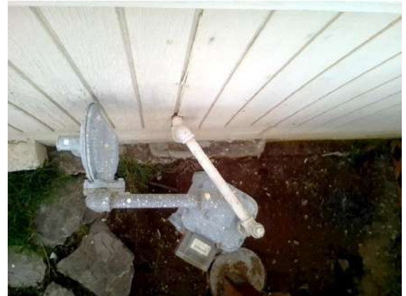
Plumbing: Gas meter located on west side of house under deck.
