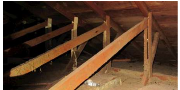
Attic Framing/Sheathing: Vertical white pieces are particleboard repairs/added support to rafters and need to be reviewed by a structural engineer. Though of no structural value, the reason they were added in the first place should be determined and remedied.
