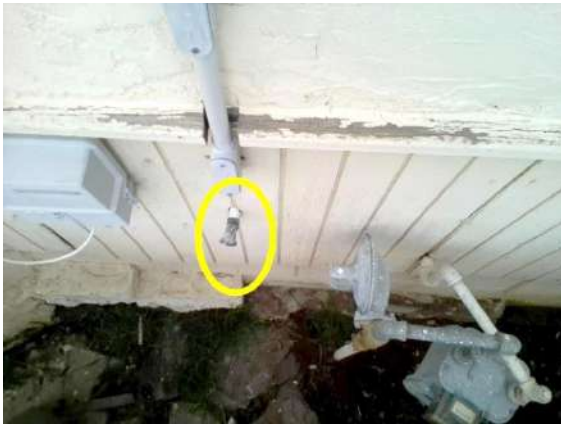
Exterior Surface: Hose bib on west side of house.
