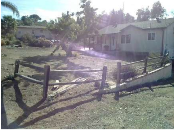
Grading / Drainage: Front of home.
