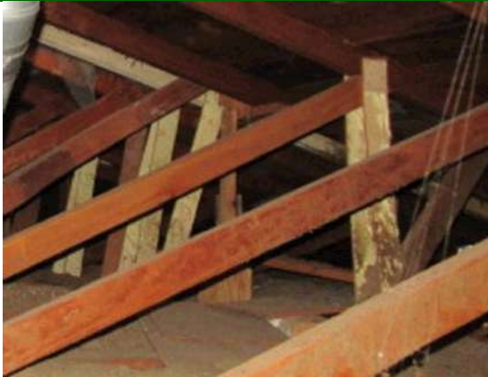
Attic Framing/Sheathing: Vertical white pieces are particleboard repairs/added support to rafters and need to be reviewed by a structural engineer. Though of no structural value, the reason they were added in the first place should be determined and remedied.
