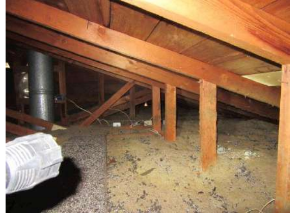
Attic Framing/Sheathing: Roof deck of original structure consists of planks.
