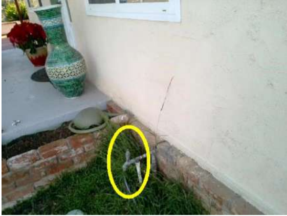
Exterior Surface: Hose bib in front west of porch.
