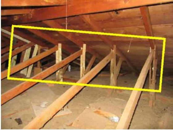
Attic Framing/Sheathing: Vertical white pieces are particleboard repairs/added support to rafters and need to be reviewed by a structural engineer. Though of no structural value, the reason they were added in the first place should be determined and remedied.
