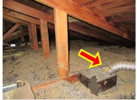
Attic Ventilation: Hallway bathroom exhaust fan and flexible pipe which terminates in attic near ventilation turbine.
