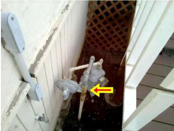
Plumbing: Gas shut-off
