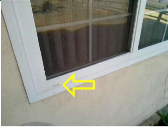
Windows: Weep holes (typical)
