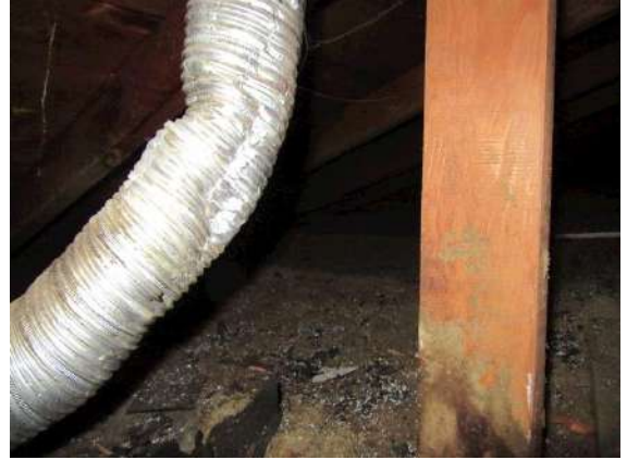
Attic Ventilation: Minor kink located in hallway bathroom flexible exhaust pipe.
