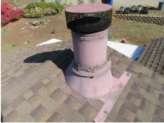
Flashing/Valleys: Living room chimney flue
