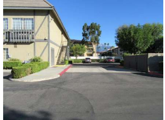
Walks / Steps: Sidewalk at rear of property.
