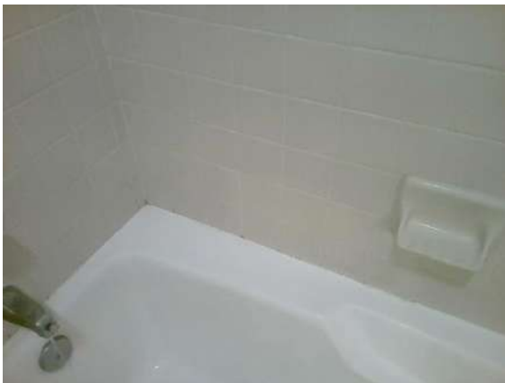
Guest Bathroom 258: Slight mold and/or mildew present or caulk cracking at joint.
