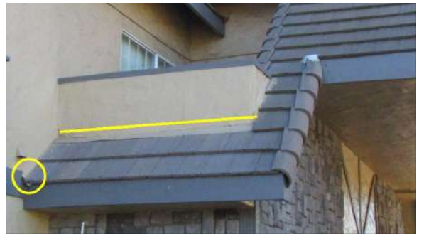
Flashing/Valleys: Step flashing observed. Typical.
