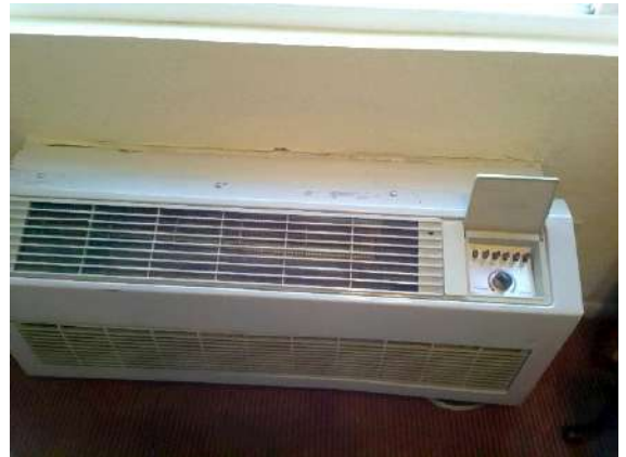
Guest Room 114: Older style HVAC wall air conditioner separating from wall slightly. Unit was operational at time of inspection.
