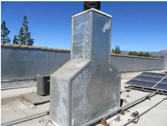
Front Lobby Fireplace/Stove: Chimney on roof.
