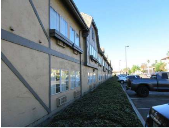
North Retaining Wall: North side of building from north-east corner of building.
