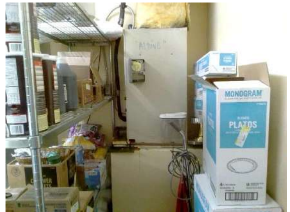
Heating: Small furnace/air ventilation unit servicing meeting room.
