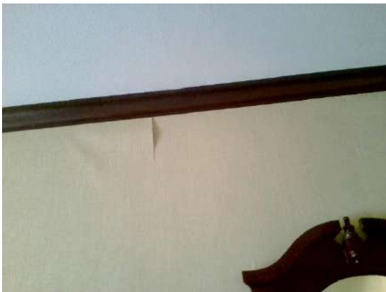
Guest Room 211: Slight tear in wallpaper.
