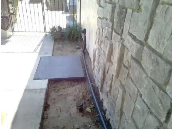
Exterior grease trap for new kitchen being installed, not complete.
