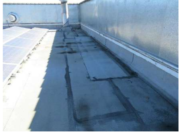
MAIN FLAT ROLLED ROOFING: Evidence of another recent roof repair.
