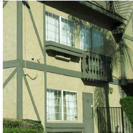
Windows: Combination of newer vinyl and older steel windows throughout the property.
