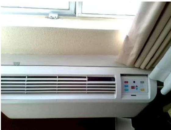
Guest Room 134: Newer style HVAC wall unit operational at time of inspection.
