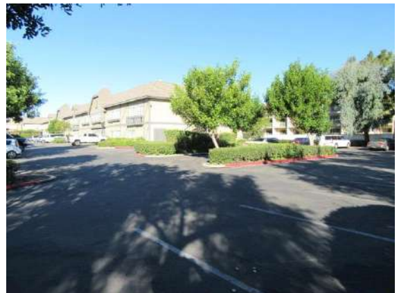
Parking Area: Looking from furthest south-west corner of lot.
