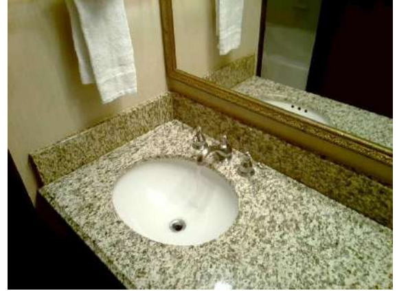
Guest Bathroom 211: stopper missing
