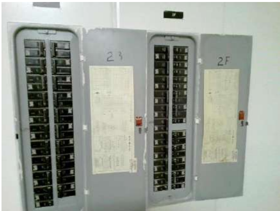
Common Areas Electrical: Sub panels in exercise room.
