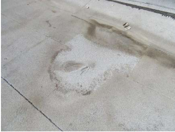
Main Flat Rolled Roofing: Evidence of ponding and granular loss with it piling up at low spots.
