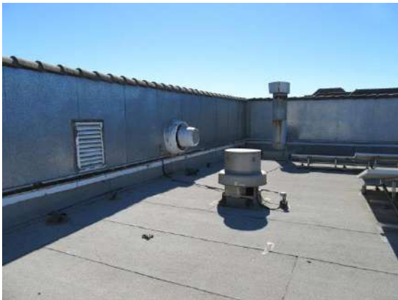
Attic Ventilation: Mansard roof ventilation observed.
