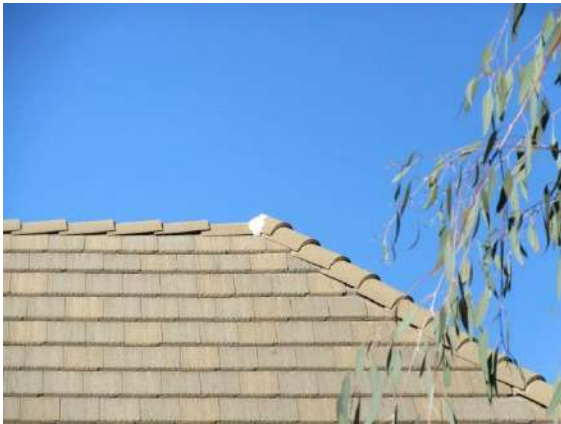
Flashing/Valleys: Typical concrete tile roof ridge.
