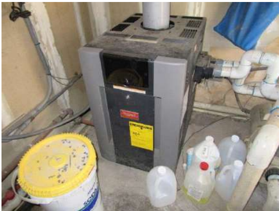
Swimming Pool Equipment : Pool gas heater.
