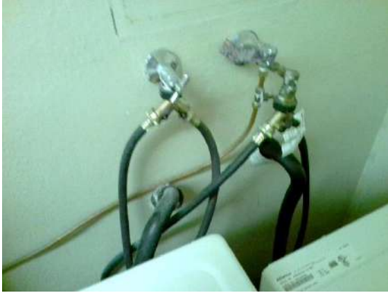
Guest Laundry Facilities (Second Floor): Water hookups and drain pipe.
