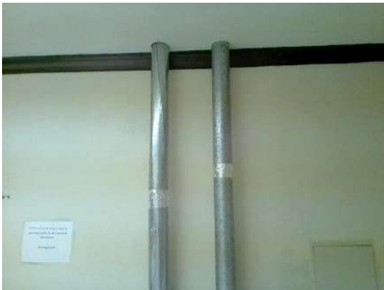
Guest Laundry Facilities (Second Floor): vertical vent pipe from dryers.
