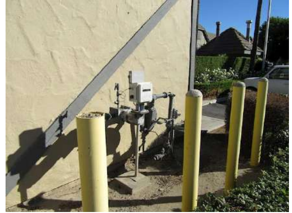
Utility Connections: Gas distribution regulator.
