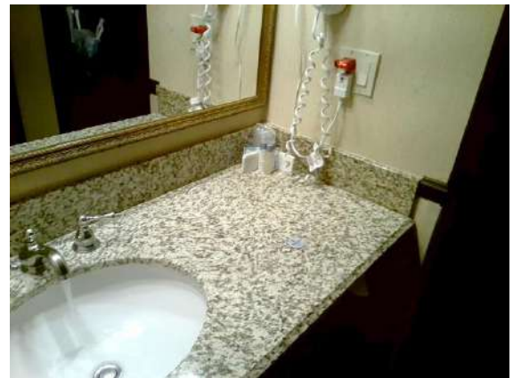
Guest Bathroom 209: GFCI installed and operational
