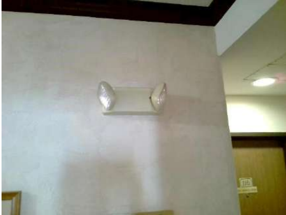
Low voltage/Fire Alarm Panel.: "Bug Eye" emergency lighting in place. Typical.
