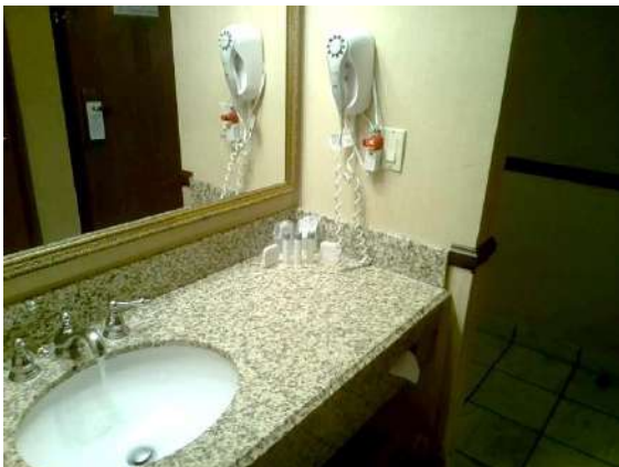
Guest Bathroom 134: GFCI installed and operational
