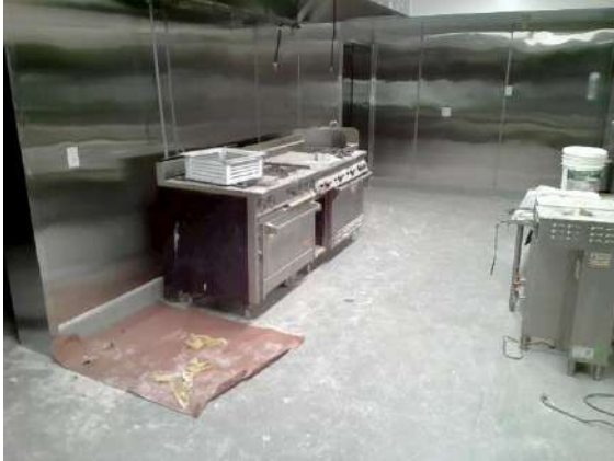
Kitchen: Kitchen under construction
