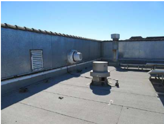
Rooftop Power Ventilation: Laundry room ventilator.
