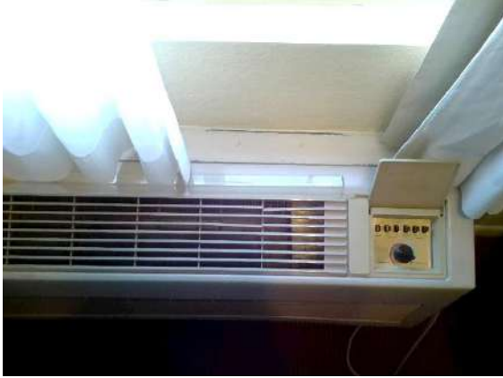
Guest Room 120: Older style HVAC wall unit operational at time of inspection.
