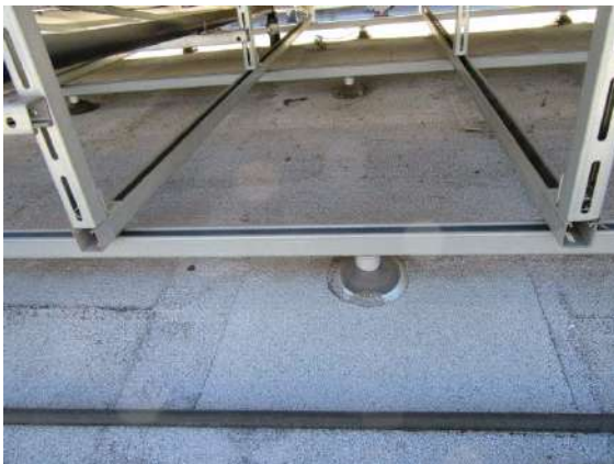
Solar Panels Installed on Roof: Solar panel rack assembly roof attachments appear of good workmanship with rolled roofing material applied over Vulcan flashing boot.
