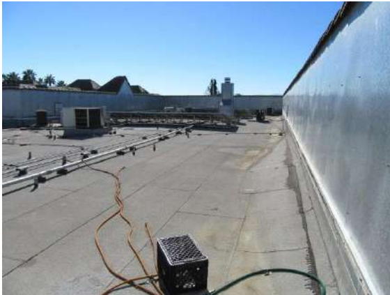
Main Flat Rolled Roofing: Field view of flat roof.
