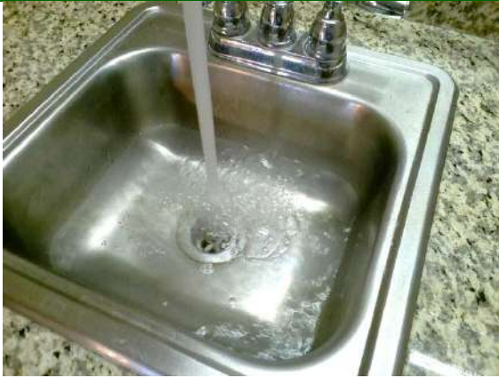
Guest Room 209: Sink slow to drain.
