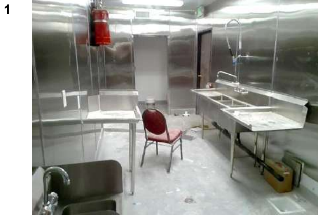
Kitchen under construction.
