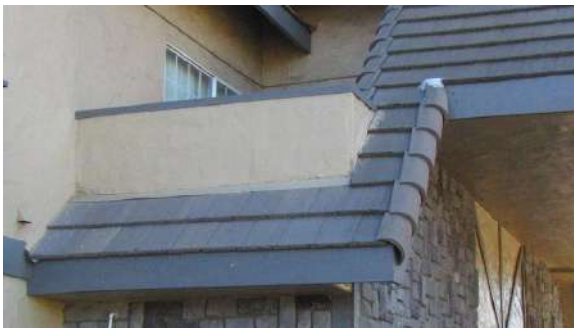
Mansard Concrete Tile Roofing: Typical view of various transitions in concrete roof tile.
