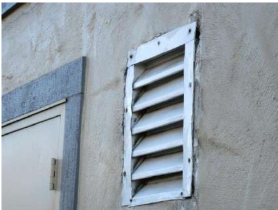
Exterior Surface: Vent repair not complete. Requires stucco repair and paint.
