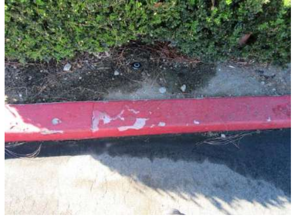
Driveway: Fire lane curb paint peeling.
