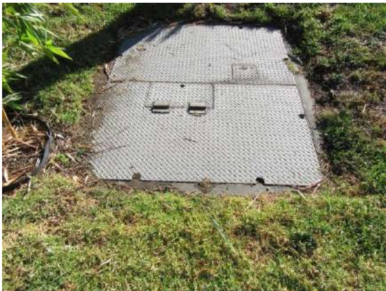
Utility Connections: Gas/electric vault located in front of property.
