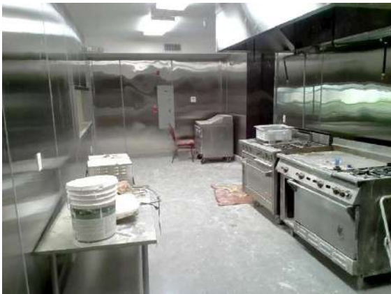
Kitchen: Kitchen under construction
