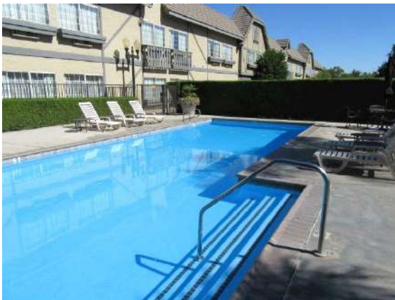
Safety/Signage/ADA: Handrail & steps entering pool
