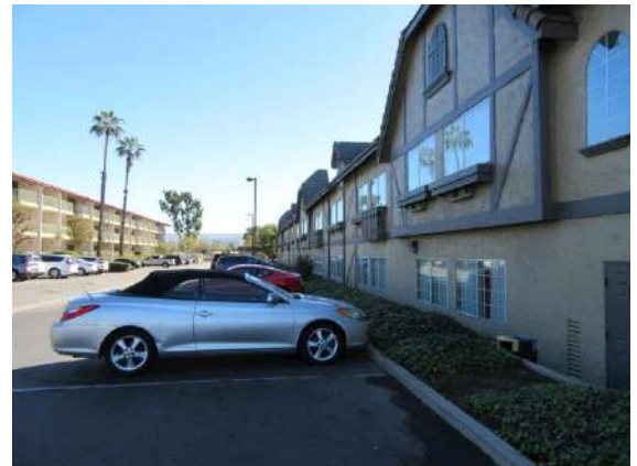
North Retaining Wall: Parking lot is another property.
