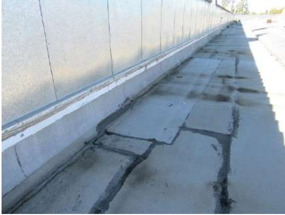
Main Flat Rolled Roofing: Evidence of recent patch.
