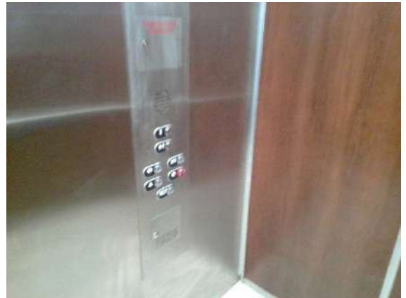
Elevator: Control panel of elevator.
