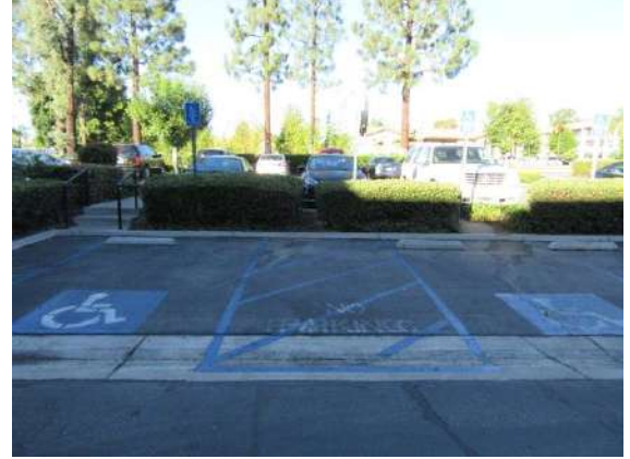
ADA/Handicapped Parking & Path of Travel: Handicap parking with required van access.
