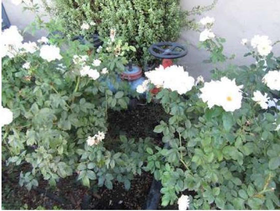
Utility Connections: Main water shut-off/backflow preventer.
