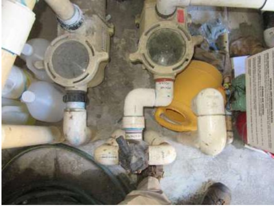
Swimming Pool Equipment : Inspection portal shows no "bubbles" indicating no leak within the system.
