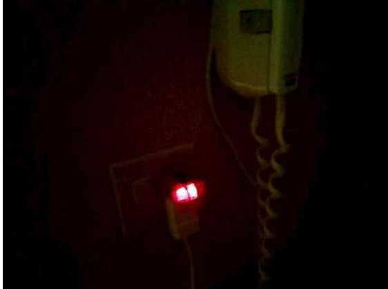
GUEST BATHROOM 241: Bathroom in room 241 has the wires crossed - the hot and neutral have been reversed.
