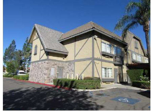
Mansard Concrete Tile Roofing: Typical field of concrete tile roofing shingles on perimeter of entire building.
