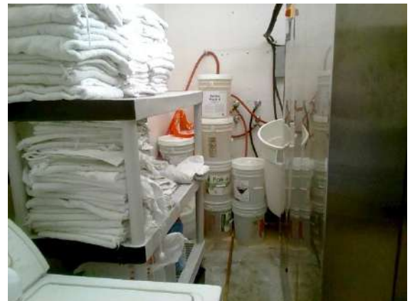
Hotel Laundry Facilities (First Floor): Water connections for washing machines.
