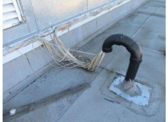
Low voltage wiring pipe chase.
