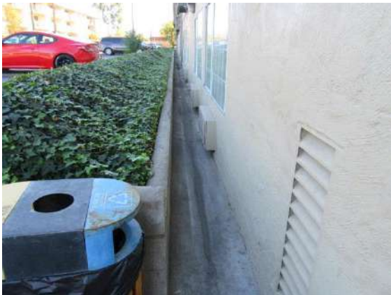
North Retaining Wall: North side of the building from about center of retaining wall length..
