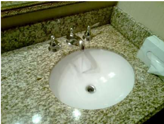
Guest Bathroom 241: Sink drain stopper missing.
