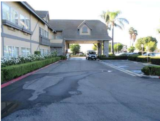
Driveway: North looking south (towards airport.).
