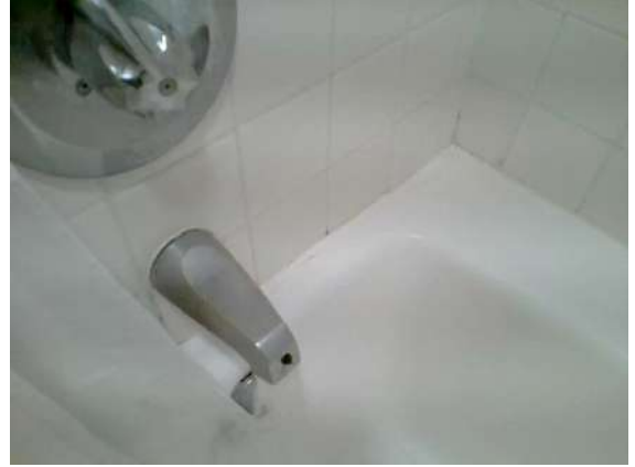
Guest Bathroom 241: Shower diverter missing - could not turn on shower.
