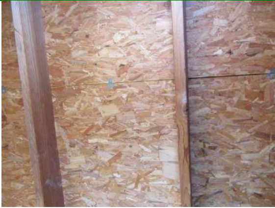
Interior of Mansard Facad: OSB used to sheath deck of concrete tiled mansard roof.
