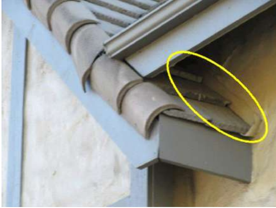
Flashing/Valleys: Step flashing observed. Typical.
