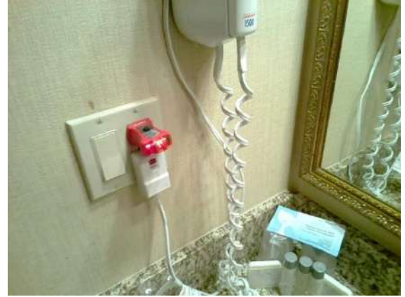
Guest Bathroom 241: GFCI installed and operational however the hot and neutral have been reversed.
