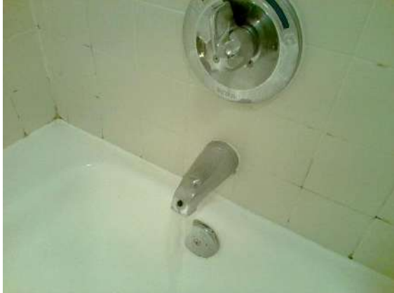
GUEST BATHROOM 229: Shower/tub diverter broken, can't use shower
