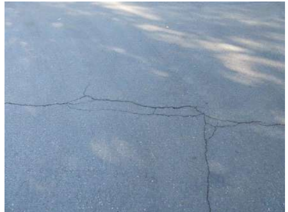
Driveway: Typical cracking in a few places with cracks no wider than 1/4".
