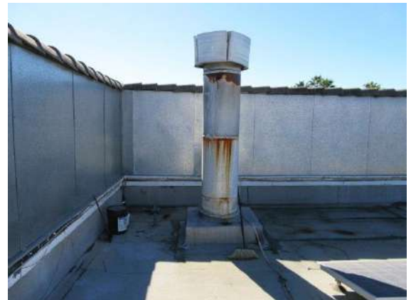
Rooftop Power Ventilation: Laundry room & equipment ventilator.
