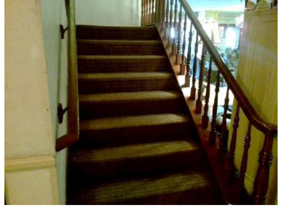
First Floor Lobby Stairs:
