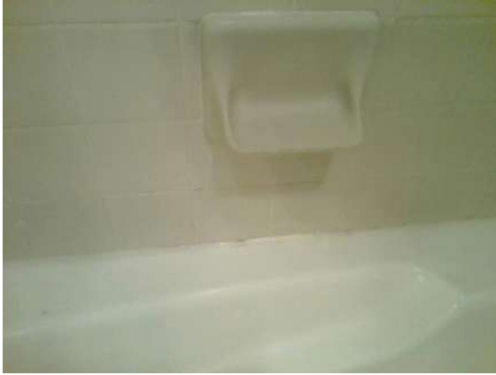
Guest Bathroom 211: Slight mold and/or mildew present or caulk cracking at joint.
