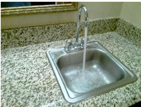
Guest Room 119: Sink slow to drain
