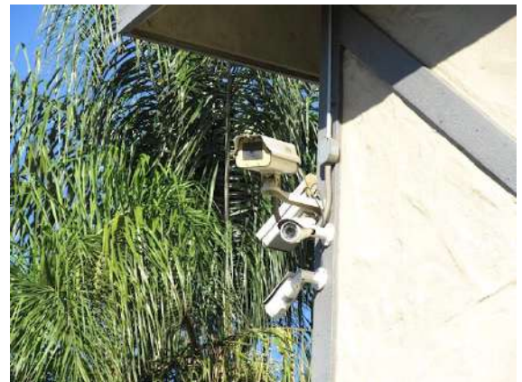
Security System: Typical CCTV located throughout the exterior of the property.
