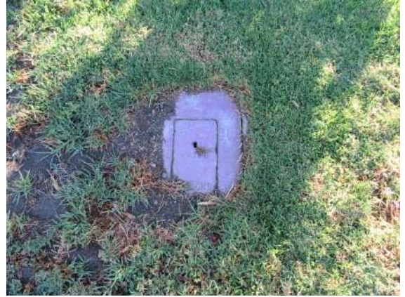
Utility Connections: "Purple pipe" recycled water control box.
