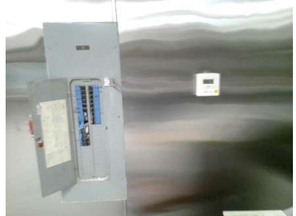
Kitchen: Electrical sub panel for kitchen.
