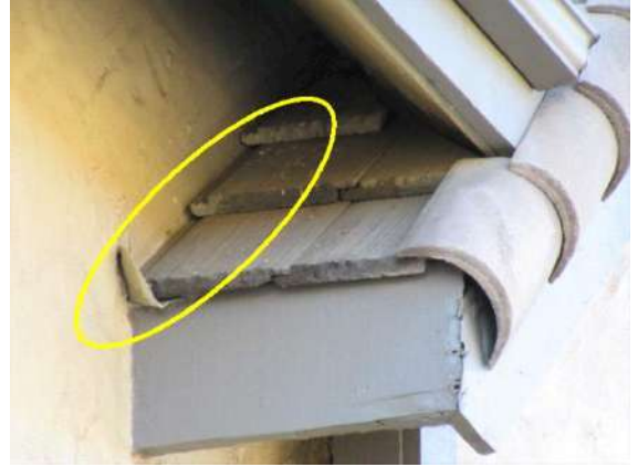
Flashing/Valleys: Step flashing observed. Typical.
