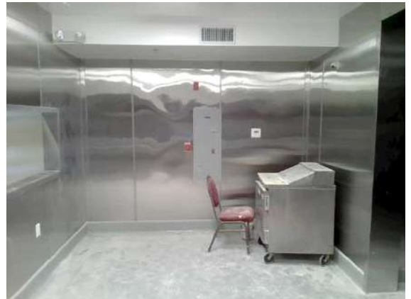
Interior wall which used to be exterior doors as shown in the previous photo.
