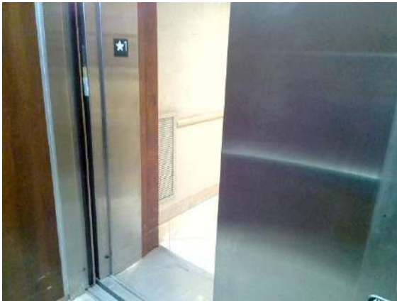
Elevator: Door operational.
