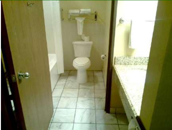
Guest Bathroom 134: So far all the exhaust fans seem to work
