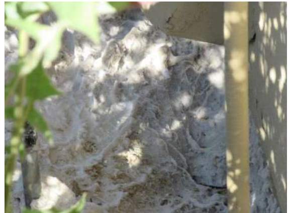
HOTEL LAUNDRY DRYER VENTING: Accumulation of dryer lint in planter bed directly outside commercial dryer.
