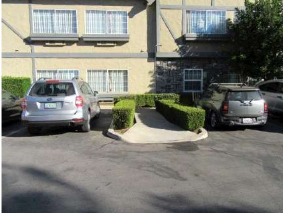
Walks / Steps: Access to exterior hallway doors at south side of building.
