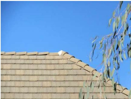
Mansard Concrete Tile Roofing: Concrete applied to ridge tile where transition is made. All appeared to be in good condition.
