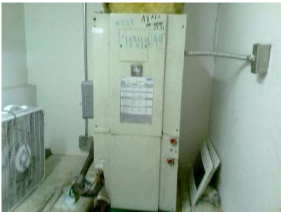
Heating: Heat/ventilation unit in kitchen undergoing remodeling.
