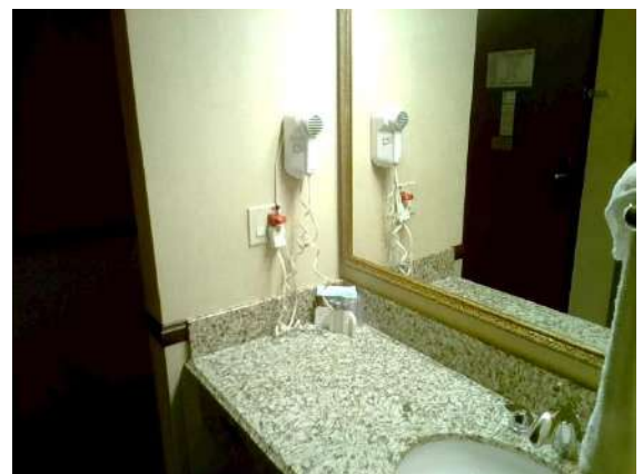
Guest Bathroom 258: GFCI installed and operational
