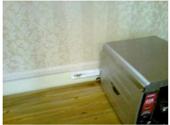
Meeting Room - currently being used as breakfast room: Burnt power strip still plugged into wall. Recommend removal.
