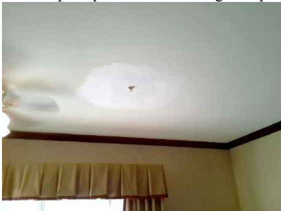
GUEST ROOM 235: Incomplete patch around ceiling fire sprinkler & masking tape on wallpaper seam.
