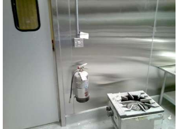
Kitchen under construction.
