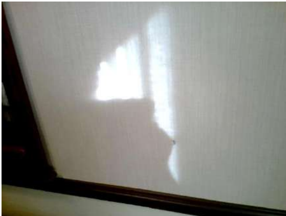
Guest Room 241: Wallpaper seam separating
