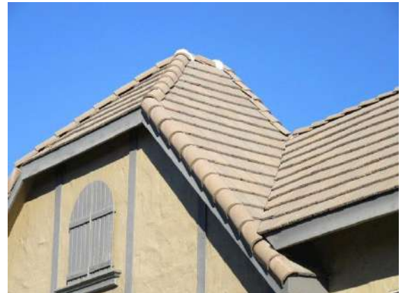
Flashing/Valleys: See next photo for close-up.
