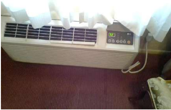
Guest Room 229: Newer style HVAC wall unit operational at time of inspection.
