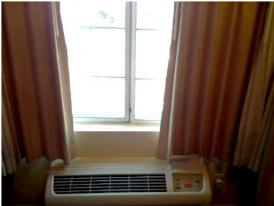
Guest Room 209: Steel windows difficult to open. Newer style HVAC wall unit operational at time of inspection.
