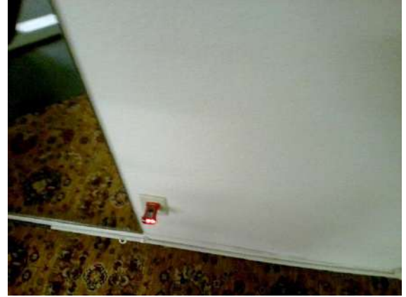
Exercise Room: Random sampling of electrical outlets indicated proper operation.
