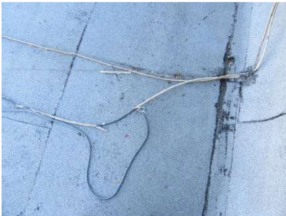
Low voltage/Fire Alarm Panel.: Low voltage wire (system unknown) on roof exposed to the elements and missing wire nuts.
