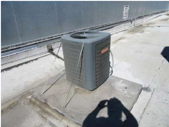
Rooftop HVAC Units: Newer rooftop condenser HVAC unit.
