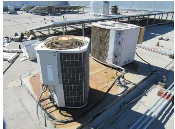
Rooftop HVAC Units: Average life remaining on these two HVAC units.
