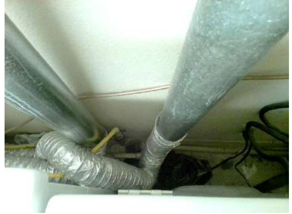
Guest Laundry Facilities (Second Floor): Improper transition vent used to connect dryer to vertical steel vent pipe.
