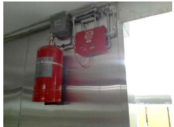
Kitchen: Fire suppression system partially installed. Requires charging. Recommend professional expert be hired to verify operation once construction is complete.
