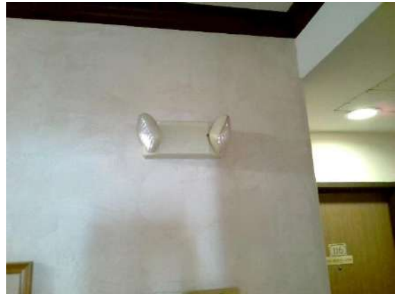
First Floor Hallways: Emergency lighting during power failure throughout. Typical.
