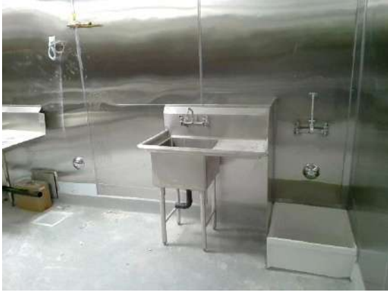
Kitchen: Kitchen under construction
