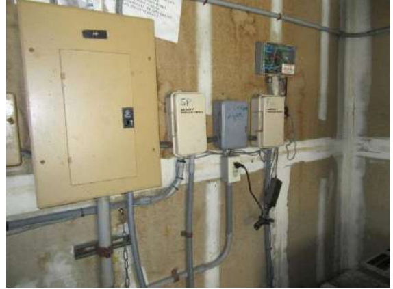
Swimming Pool Equipment : Pump room electrical sub panel and low voltage time clocks.
