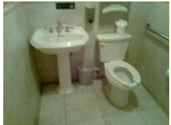
First Floor Women's Restroom:
