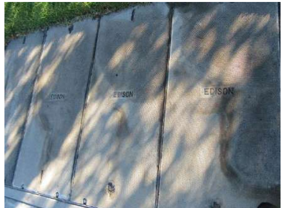
Utility Connections: Electric vault located in front sidewalk.
