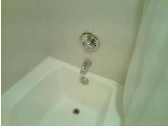
Guest Bathroom 120: Slight mold and/or mildew present or caulk cracking at joint.
