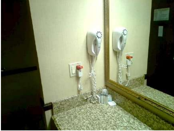
Guest Bathroom 119: GFCI installed and operational
