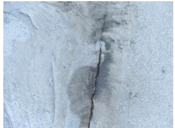
Main Flat Rolled Roofing: Existing crack and point of water intrusion that needs to be repaired before next rainfall.
