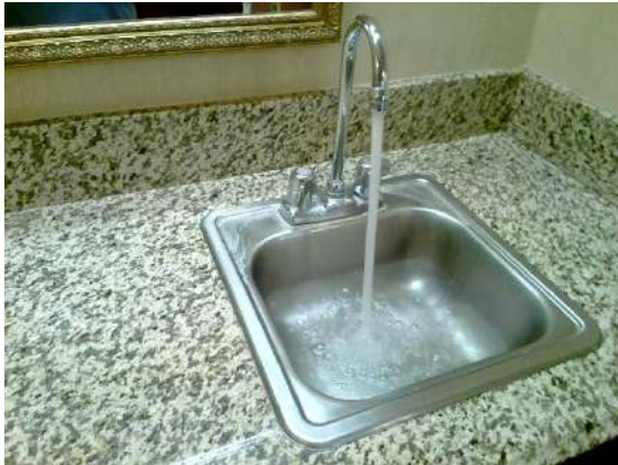
GUEST ROOM 119: Sink slow to drain
