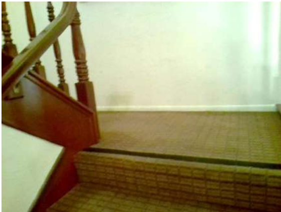
First Floor Lobby Stairs:
