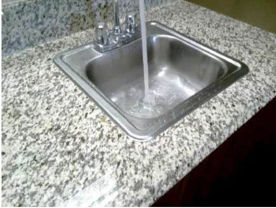
Guest Room 104 (handicapped): Water slow to drain from sink.
