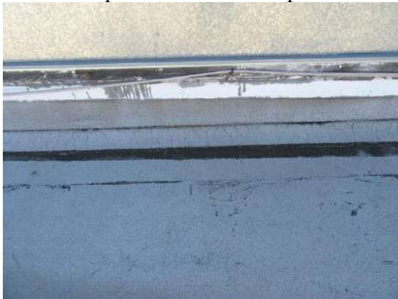
MAIN FLAT ROLLED ROOFING: Typical wear and slight cracking at coping material run up parapet wall.
