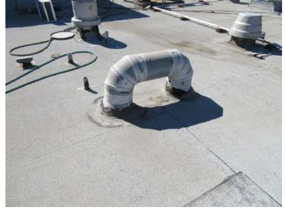
Rooftop Power Ventilation: Unfamiliar with this type of ducting. Recommend professional mechanical contractor review and advise.
