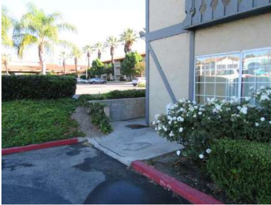
North Retaining Wall: North-west corner of building in front.
