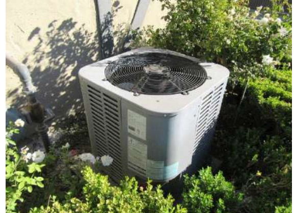
Interior/Ground Based Cooling: Outside compressor unit for hotel laundry facility.
