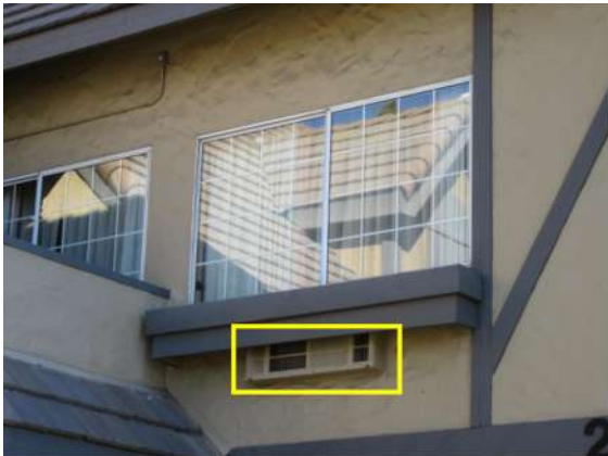
Interior/Ground Based Cooling: Typical 2nd floor guest room wall unit located under each room's window.
