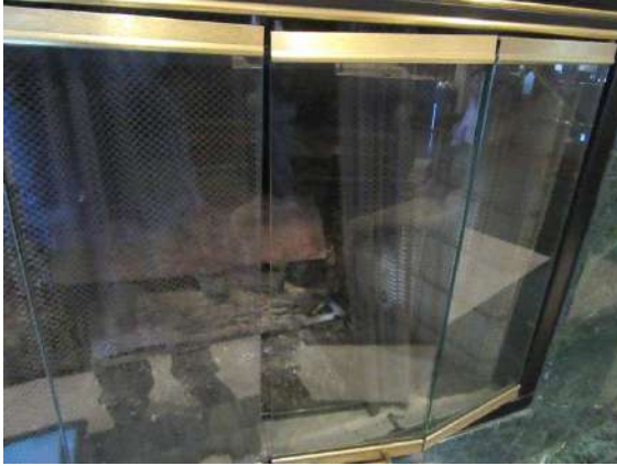
Front Lobby Fireplace/Stove: Fireplace located in lobby. Glass doors closing off fireplace broken.
