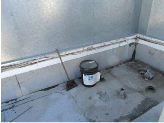
MAIN FLAT ROLLED ROOFING: Evidence of continuous roof patching with 5 gallon pail of mastic (one of two found on roof)
