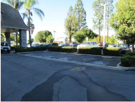
ADA/Handicapped Parking & Path of Travel: Four handicap spaces located adjacent to the lobby entrance.
