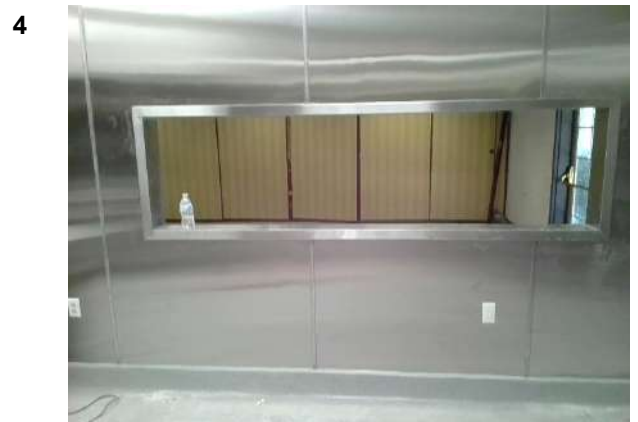
Kitchen under construction.
