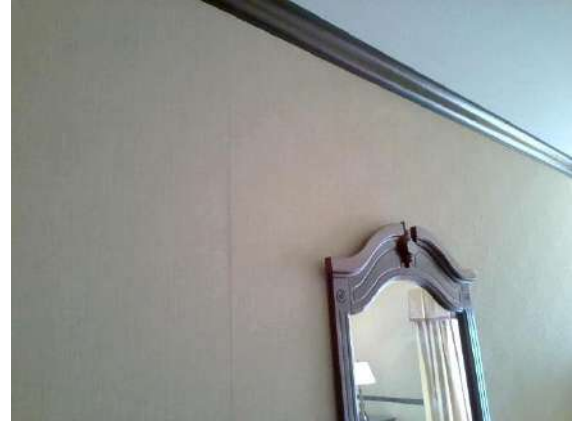
Guest Room 235: typical this room wallpaper seams peeling
