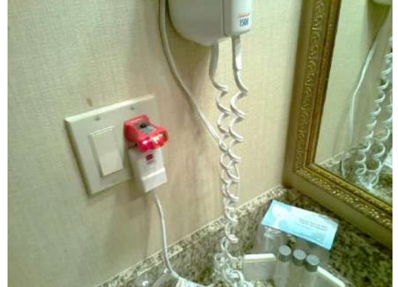
GUEST BATHROOM 241: GFCI installed and operational however the hot and neutral have been reversed.
