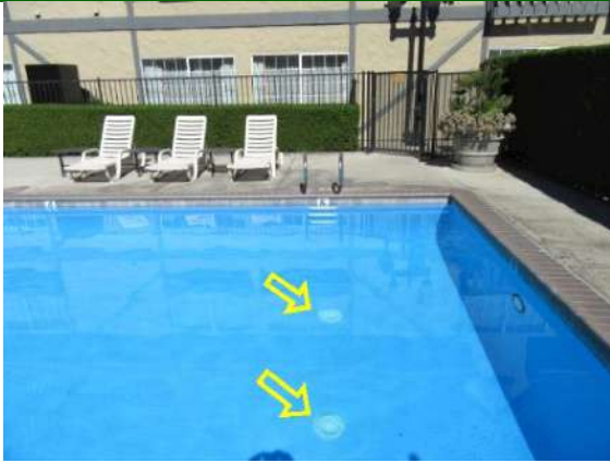
Safety/Signage/ADA: Dual suction intake drains located minimum 5 feet apart.
