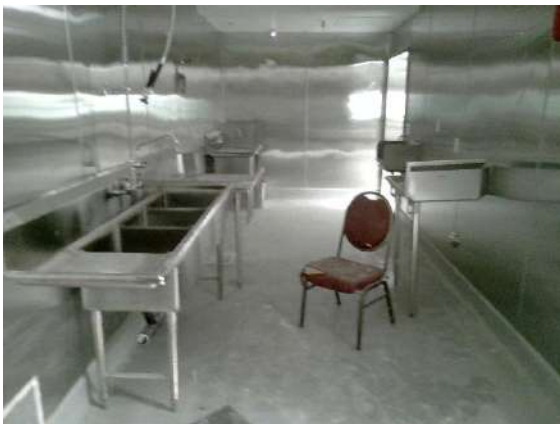
Kitchen: Kitchen under construction
