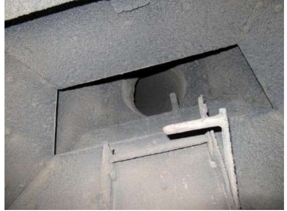
Chimney: Looking inside from fireplace hearth.
