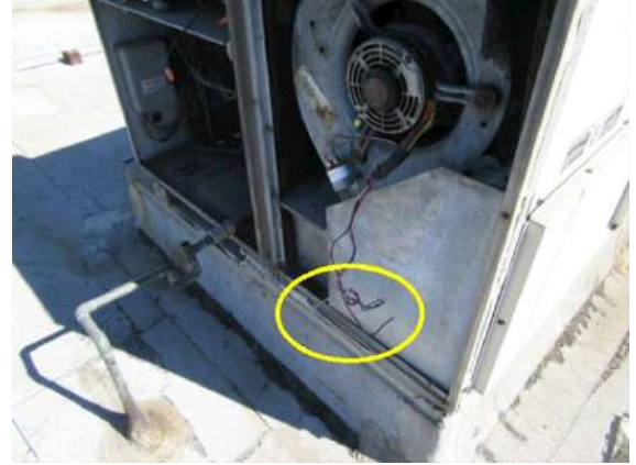
Rooftop HVAC Units: Wires disconnected from unit.
