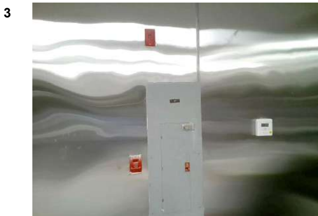
Kitchen under construction.
