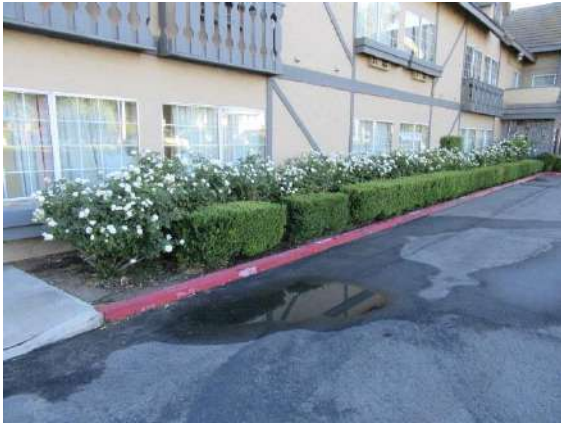
Windows: Combination of newer vinyl and older steel windows throughout the property.
