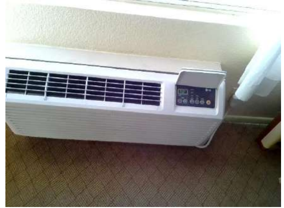
Guest Room 235: Newer HVAC wall unit was operational at time of inspection.
