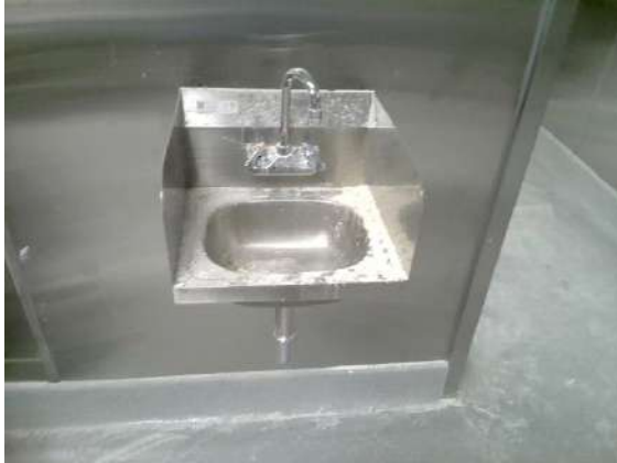
Kitchen under construction.
