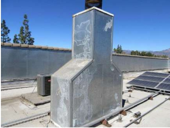
Chimney: Chimney for fireplace located in front lobby.
