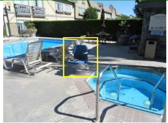
Hot Tub / Spa: ADA assistance chair device for hot tub/spa.
