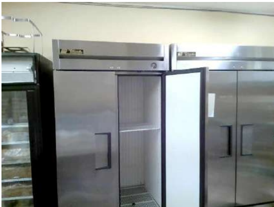
Temporary Kitchen/Coolers/Storage/Warming Room: Cooler not operational.
