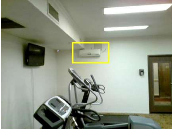
Interior/Ground Based Cooling: One of two split systems located in Fitness Center. Compressor part visible in rooftop HVAC section.
