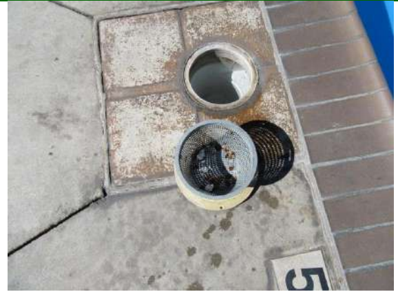
Safety/Signage/ADA: Skimmer basket
