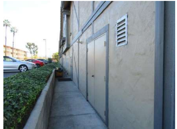
Walks / Steps: Walkway on north side of front of building.
