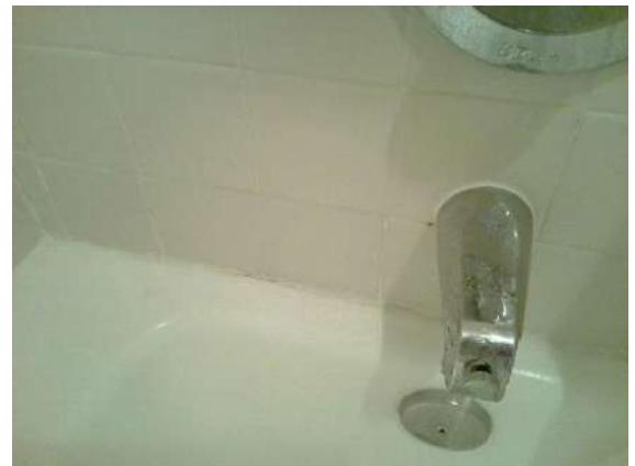
Guest Bathroom 209: Slight mold and/or mildew present or caulk cracking at joint.
