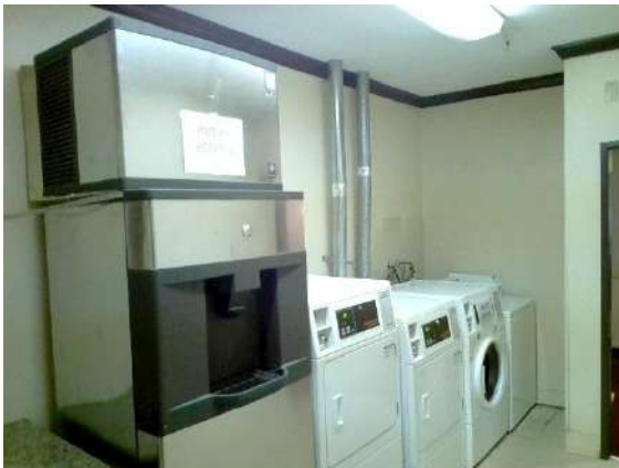
Guest Laundry Facilities (Second Floor): Guest 2nd floor coin operated laundry facility. Some of the equipment non-operational.
