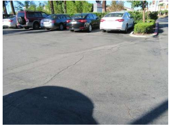
Parking Area: Occasional small cracks observed.
