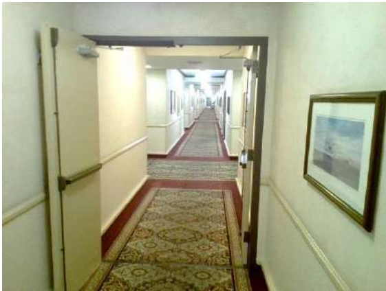
First Floor Hallways: Automatic fire doors, typical.
