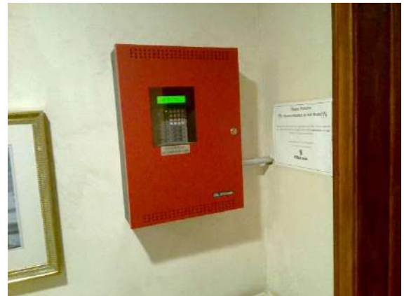
Low voltage/Fire Alarm Panel.: Fire panel located in first floor south corridor next to elevator.
