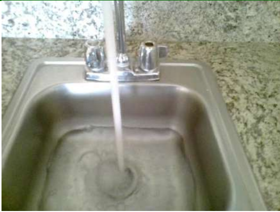
Guest Room 134: Sink slow to drain.
