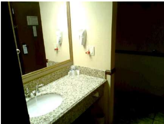
Guest Bathroom 211: GFCI installed and operational
