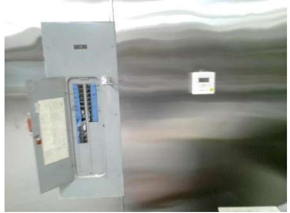
Common Areas Electrical: Sub panel located in kitchen.
