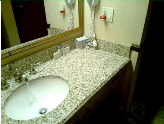
Guest Bathroom 229: GFCI installed and operational
