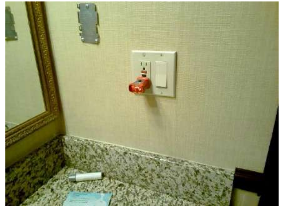
Guest Bathroom 114: GFCI installed and operational
