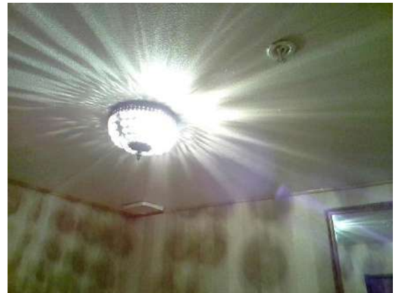
First Floor Lobby Men's Restroom:
