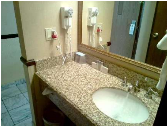
Guest Bathroom 235: GFCI installed and operational
