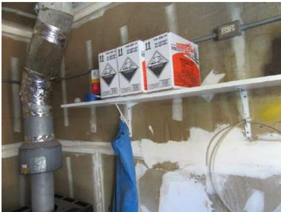
Swimming Pool Equipment : Boxes of Muriatic Acid used for cleaning.
