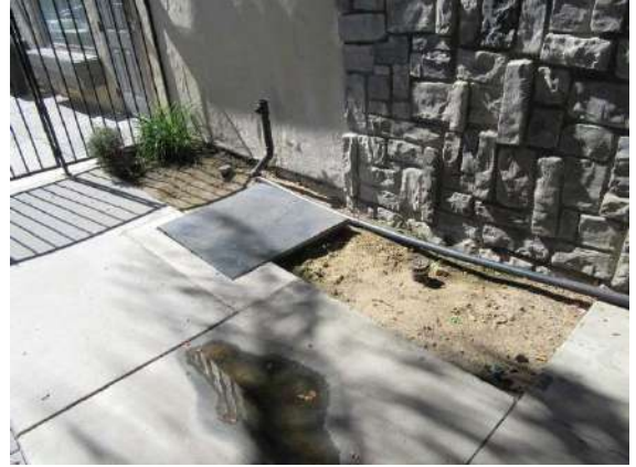
Kitchen: New kitchen grease trap/collector is being installed as part of kitchen remodel.
