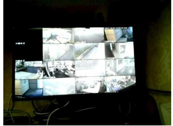
Security System: Monitors for security system located in office behind reception desk.
