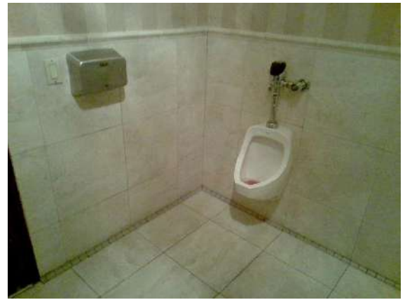
First Floor Lobby Men's Restroom:
