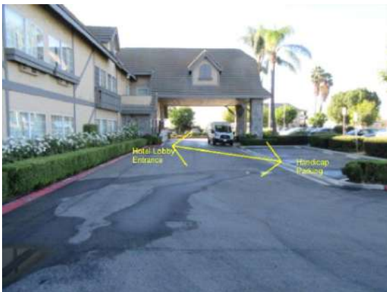
ADA/Handicapped Parking & Path of Travel: Path of travel between parking area and hotel lobby free of obstructions and tripping hazards.
