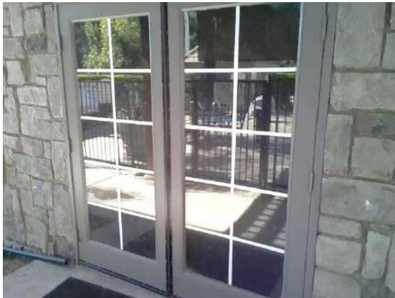
Exterior door has been covered up in new kitchen. See next interior photo.
