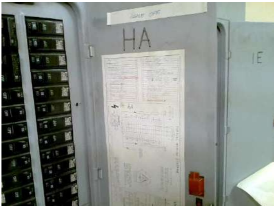
Common Areas Electrical: Sub panels in temporary prep kitchen.
