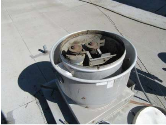
Rooftop Power Ventilation: Rooftop ventilator disassembled and inoperable.
