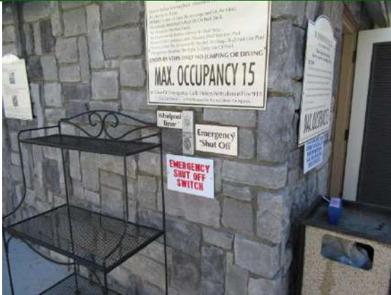
Safety/Signage/ADA: Emergency switch located close to hot tub.
