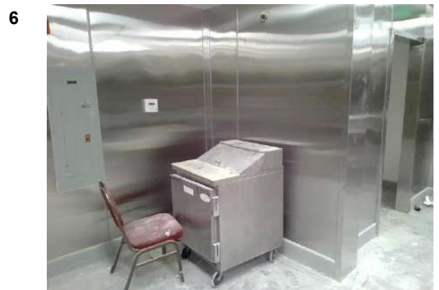
Kitchen under construction.
