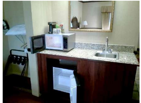
Guest Room 104 (handicapped): Refrigerator and microwave appear operational. Hot water present Water pressure good. No Ground Fault Circuit Interrupter (GFCI) on electrical outlet within 5 feet of sink. This may or may not be grand-fathered in due to age of building, Suggest contacting a professional licensed electrical contractor for review.
