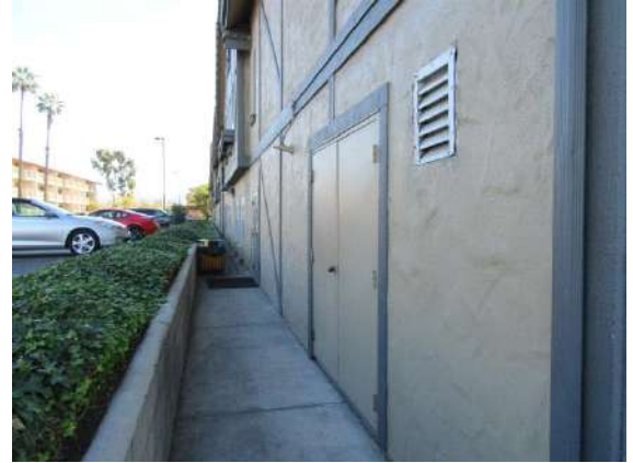
North Retaining Wall: North side of building on the west end.
