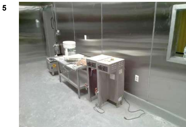
Kitchen under construction.
