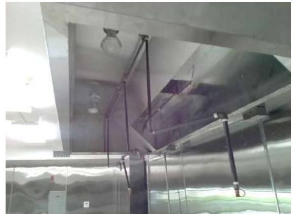
Kitchen: Fire suppression system partially installed. Recommend professional expert be hired to verify operation once construction is complete.
