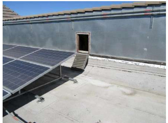
Attic Ventilation: Mansard roof ventilation observed.
