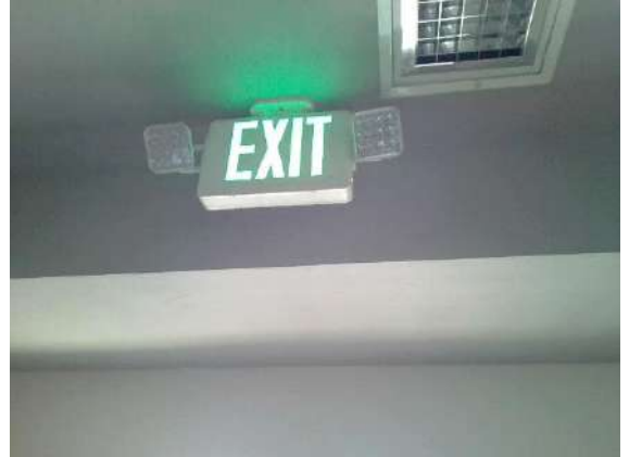
Typical emergency egress lighting.
