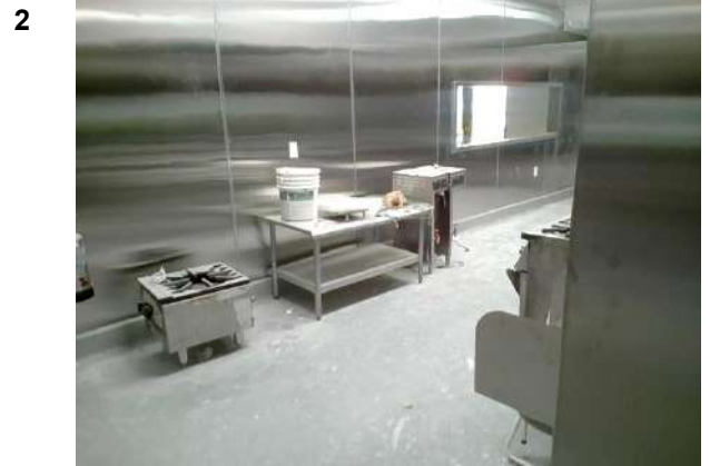
Kitchen under construction.
