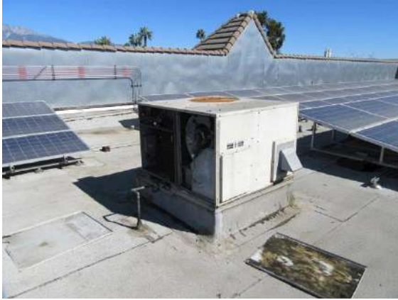
Rooftop HVAC Units: This unit has been abandoned and should be replaced, see next photo.
