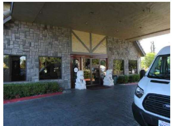
ADA/Handicapped Parking & Path of Travel: NO threshold entrance.
