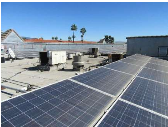
Solar Panels Installed on Roof: Typical array of solar panels on stanchions.
