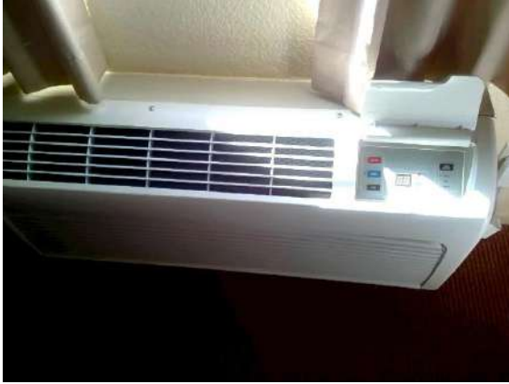
Guest Room 104 (handicapped): Newer style HVAC wall unit operational at time of inspection.
