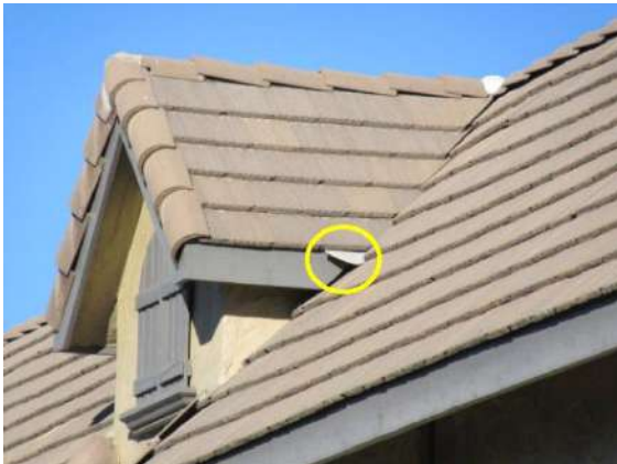
Flashing/Valleys: Valley flashing observed. Typical.
