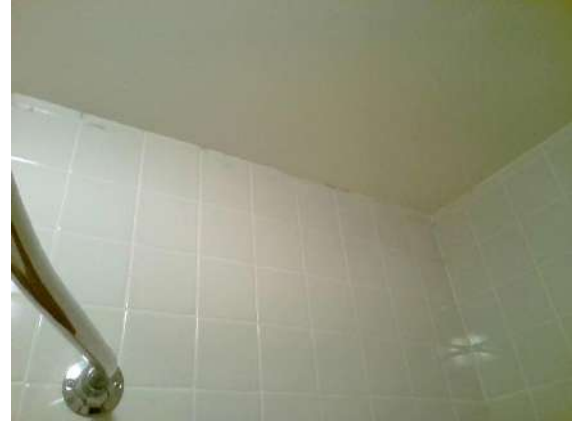
Guest Bathroom 229: Slight mold and/or mildew present or caulk cracking at joint.
