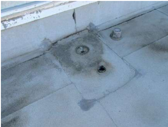
Gutters/Down Spouts: Internal downspout drain missing debris cap. Typical.
