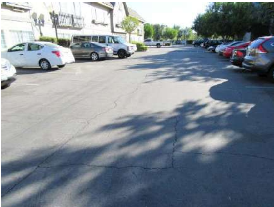
Parking Area: Driveway looking from front south-west corner looking east.
