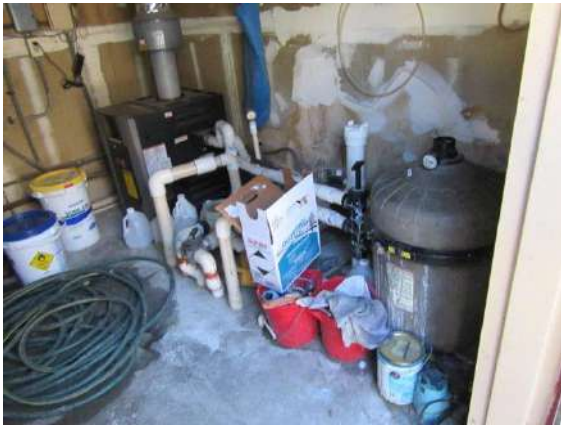
Swimming Pool Equipment : Diatomaceous earth used as filter media.
