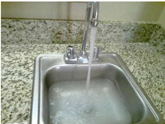
Guest Room 241: Drain slow to drain. Hot water handle nameplate missing.
