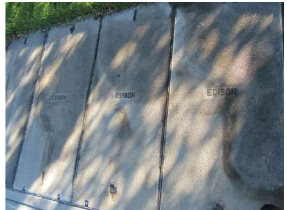
Common Areas Electrical: Main property vault for electrical service located at street within sidewalk in front of property.
