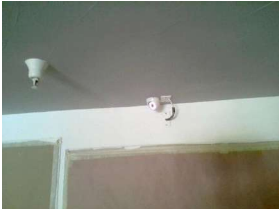
Security camera inside dining room.
