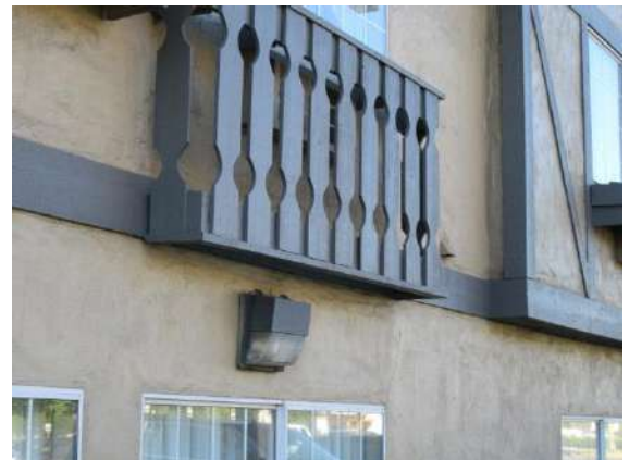
Exterior Surface: Typical 2nd floor surface structure to mimic a Juliet balcony.
