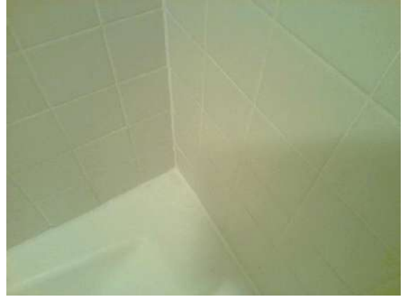
Guest Bathroom 235: Slight mold and/or mildew present or caulk cracking at joint.
