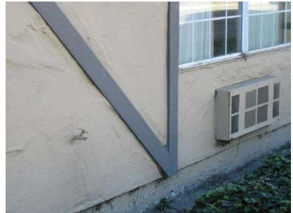
Interior/Ground Based Cooling: Typical built-in HVAC unit located in each guest room under the window.
