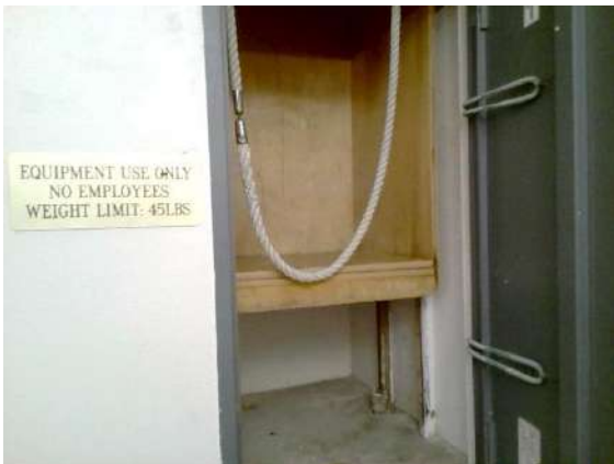
Hotel Laundry Facilities (First Floor): Dumb Waiter to deliver clean sheets, towels, etc to second floor.
