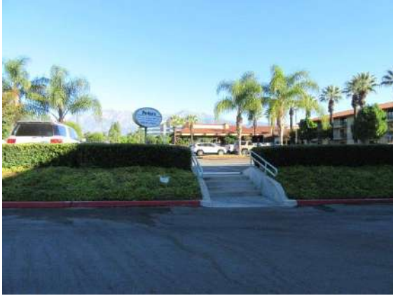
Walks / Steps: Stairs leading from Folk Inn to adjacent property at northeast corner of west/front parking area.
