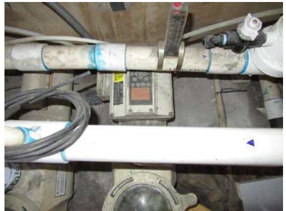
Swimming Pool Equipment :
