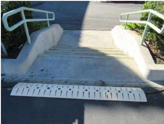
Walks / Steps: Steps leading from adjacent property to Folk Inn parking lot.
