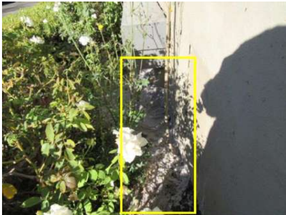
HOTEL LAUNDRY DRYER VENTING: Commercial laundry dryer vented directly outside near ground
