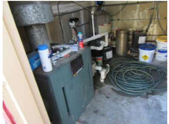
Swimming Pool Equipment : Spa gas heater.
