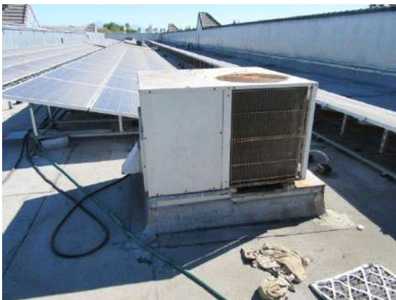
Rooftop HVAC Units: Older HVAC rooftop condensing unit.
