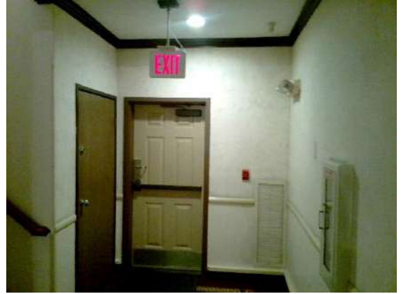
First Floor Hallways:
