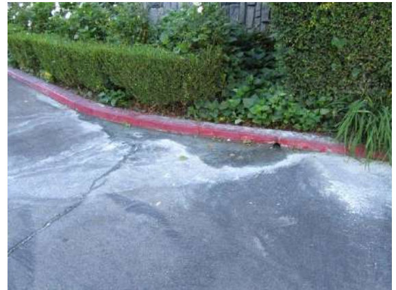
Landscaping: Typical landscaping around area between parking lot and structure.
