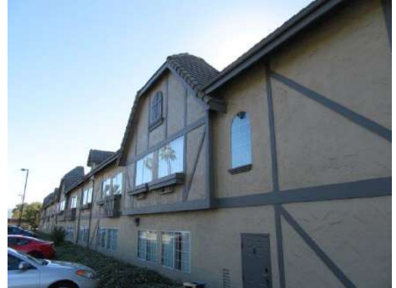
Exterior Surface: Typical stucco and wood siding in the tradition of the Tudor style.
