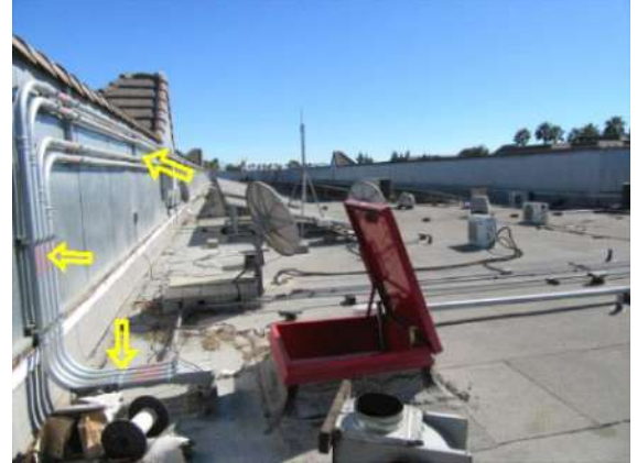
Solar Panels Installed on Roof. Conduit for solar panel connection to inverter.
