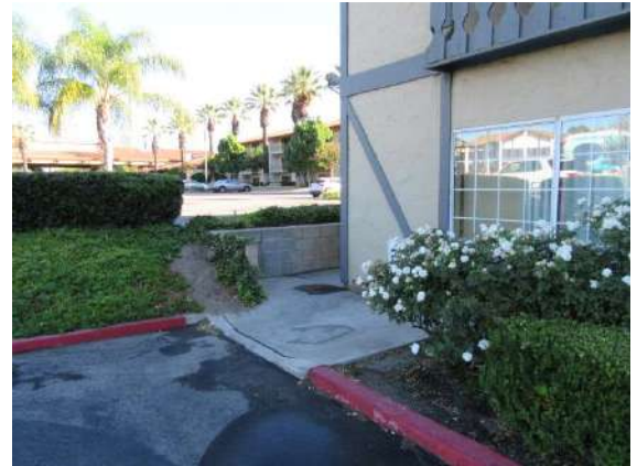
Walks / Steps: ADA/Handicap access to walkway on north side of building.
