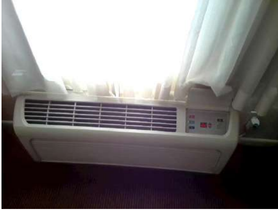
Guest Room 241: Newer style HVAC wall unit was operational at time of inspection.
