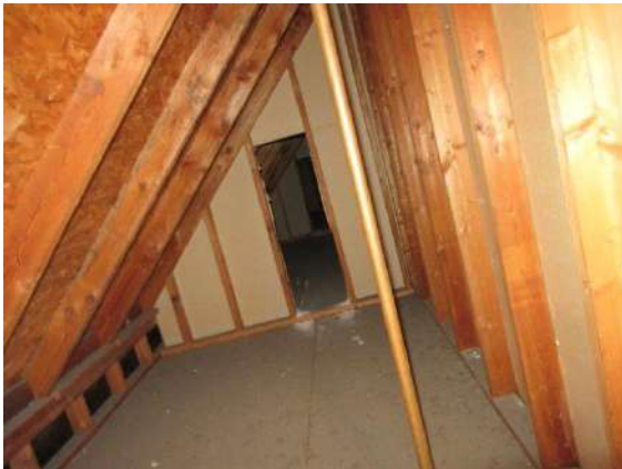
Interior of Mansard Facad:
