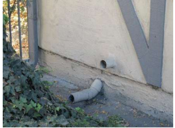
Gutters/Down Spouts: Exit point of internal drain system.
