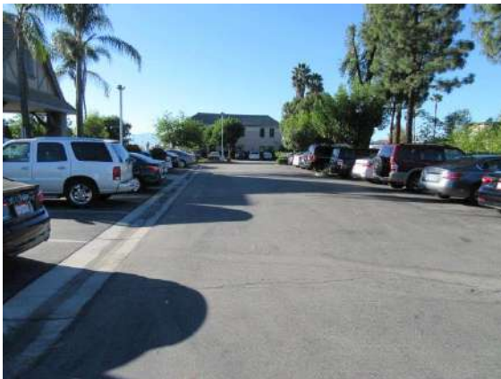
Driveway: East looking west on south side of building
