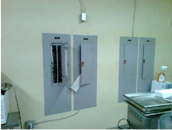
Common Areas Electrical: Electrical sub panels located in temporary food prep area servicing breakfast area.
