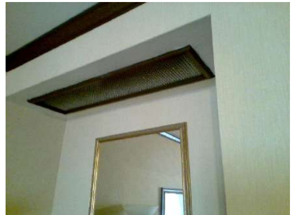
Guest Room 258: Light over sink inoperable
