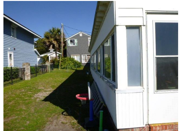
Grading / Drainage: View of right side property and grading
