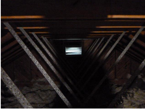
Attic Ventilation: View of gable vents located on each end of attic
