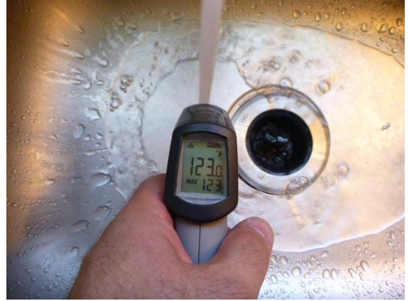
Water Heater: View of water temperature at the kitchen sink
