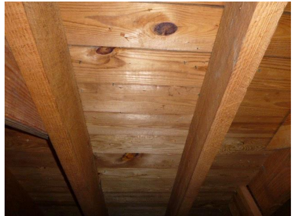
Attic Framing/Sheathing: Views of attic framing and sheathing
