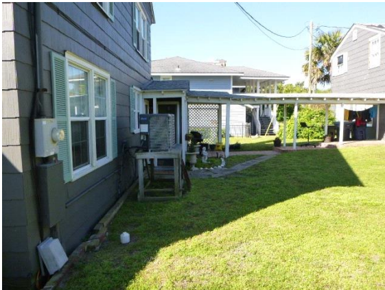
Grading / Drainage: View of front property and grading
