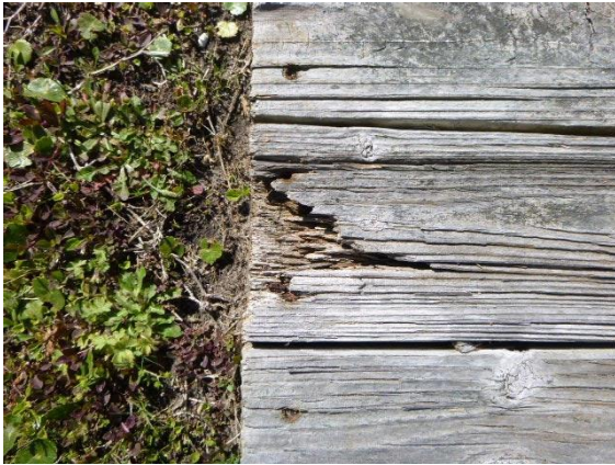
Rear Wood Walkway: Views of weather boards on rear wooden walkway
