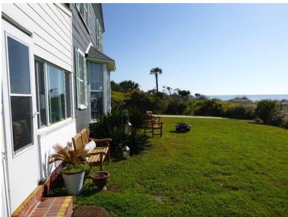
Grading / Drainage: View of rear property and grading
