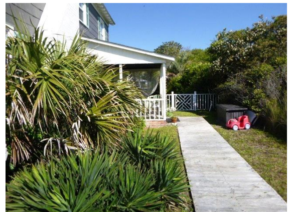
Grading / Drainage: View of left side property and grading
