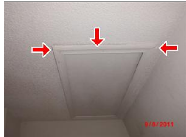
12.0 Picture 2 seal attic access
