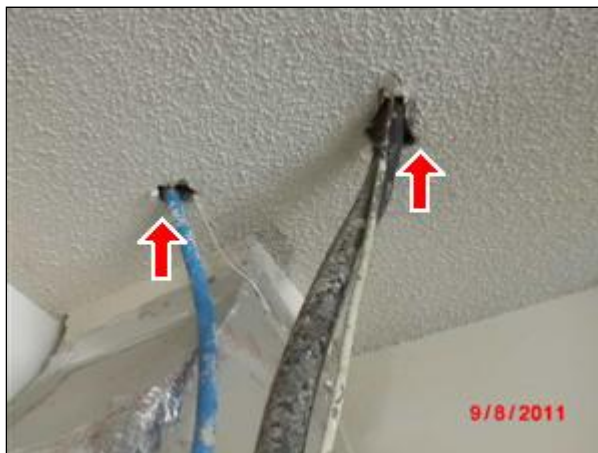
3.0 Picture 1 sela around pipes
