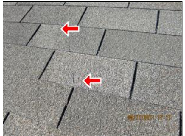
C. Picture 2 Granules have come off at the edges
