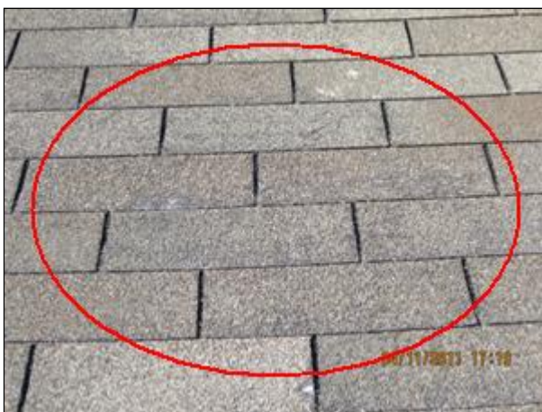
C. Picture 3 Hail damage and lost granules
