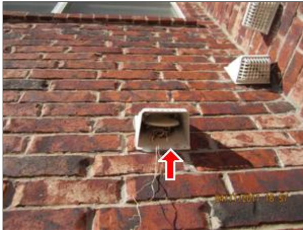
J. Picture 1 Dryer vent has birds nest inside
