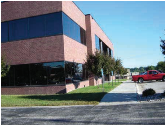
Grade and landscaping
