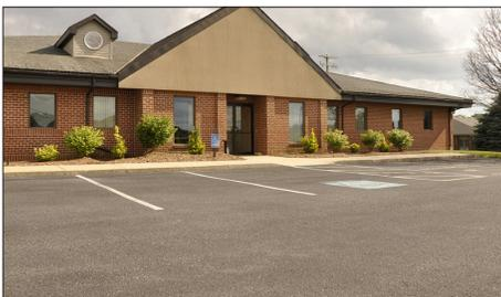
» Asphalt is composed of aggregates bound together with asphalt cement. The mixture is heated and combined with hot asphalt cement and installed over a base, usually compacted aggregate.
