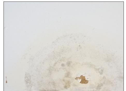
The first step is to find out what caused the stain — it was likely a leaky roof or pipe — and fix the problem. Otherwise, once you cover the ceiling stain, you'll just wind up with another one in its place. As soon as possible, call a certified roofing contractor or plumber to fix the problem. After the leak is fixed, the next step is to repair or replace the areas in the ceiling that were damaged.
