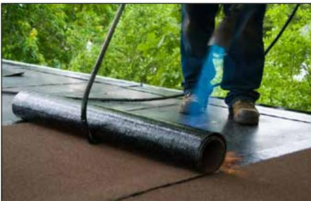
In general, a flat roof begins with the roof decking, the material covering the metal or wooden trusses supporting the roof. Next is a layer of rigid foam insulation. The roof membrane and a waterproofing material form the topmost layer of the roof. The waterproofing material is held in place with glue, mechanical means, or a covering of ballast — small granular minerals.
