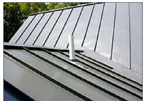
Standing seam metal actually offers clear advantages to other roof types when mounting equipment becomes necessary. Unlike other types of roofing, metal is a rigid, high tensile material. The seam area creates a beam-like structure that can provide convenient anchorage for things like walkways, solar panels, condensing units, gas piping, and the like without damaging the roof membrane.
