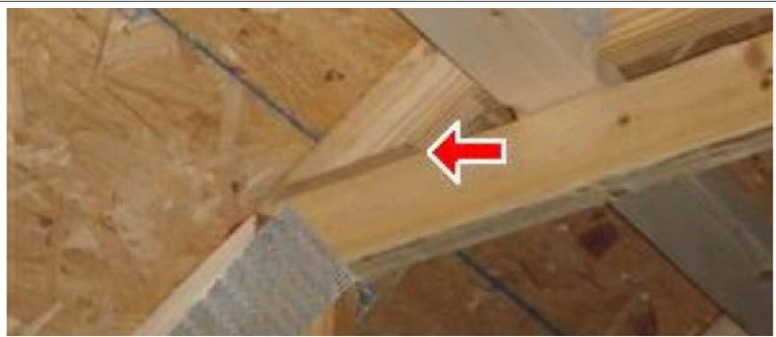
The photo above shows the gap between the piggyback trusses and the sheathing laps — approximately 3 inches with no 2x4 connection support on angle chords. In this case, there should be at least one 6-foot-long 2x4 fastened to the side of the angle chords of the trusses. This board should be centered on the gap.
