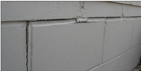
Diagonal cracks, many times starting in a corner or at a window or door opening, or horizontal cracks indicate foundation wall movement. This movement is usually
